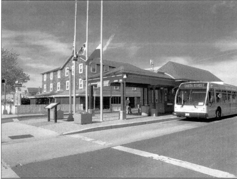
Figure 1: Facade and side elevation, DSCN6721 (RCG&A 2021)
