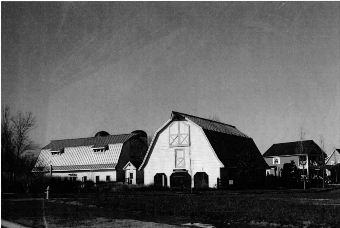
Tenant Farm Complex, general property overview, looking west
