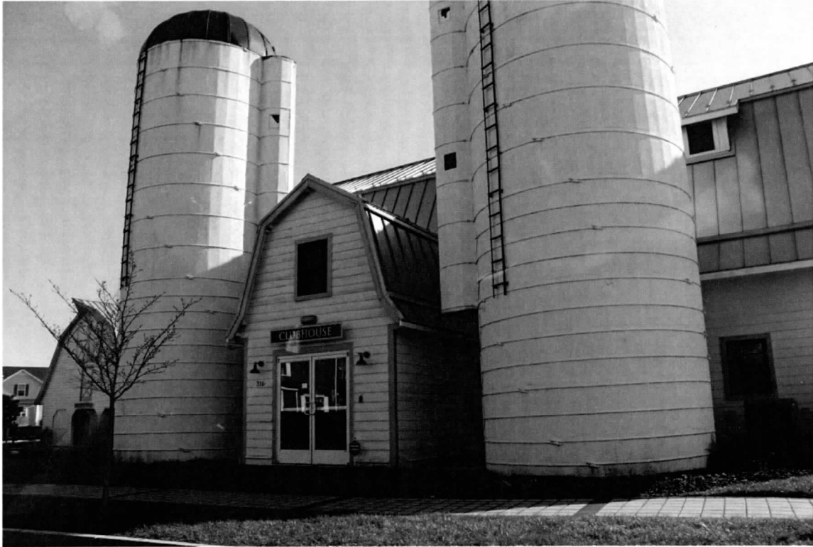
Tenant Farm Complex, west barn, northwest façade, looking southeast
