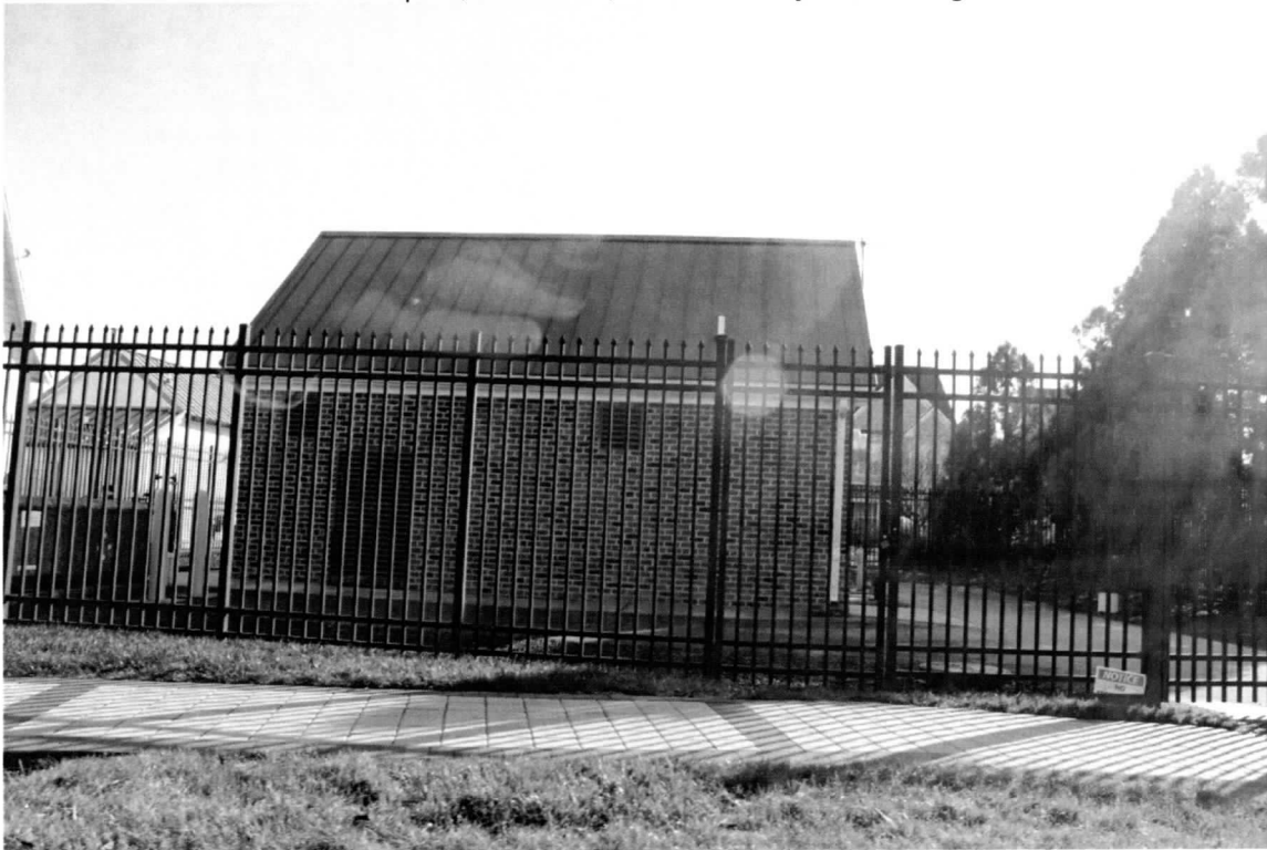
Tenant Farm Complex, pumping station, northwest elevation, looking southeast
