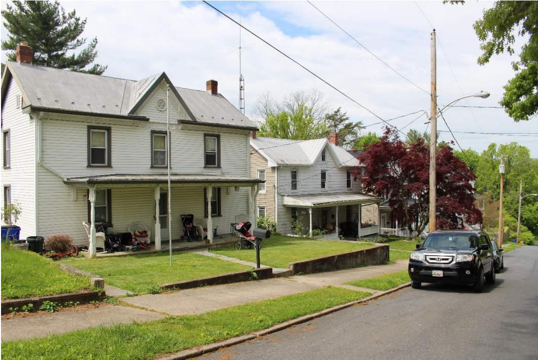
Photo 9 of 34: MD_FrederickCounty_BrunswickHD(Addl Doc)_009.tif I Houses along Park Avenue, Looking Southwest
