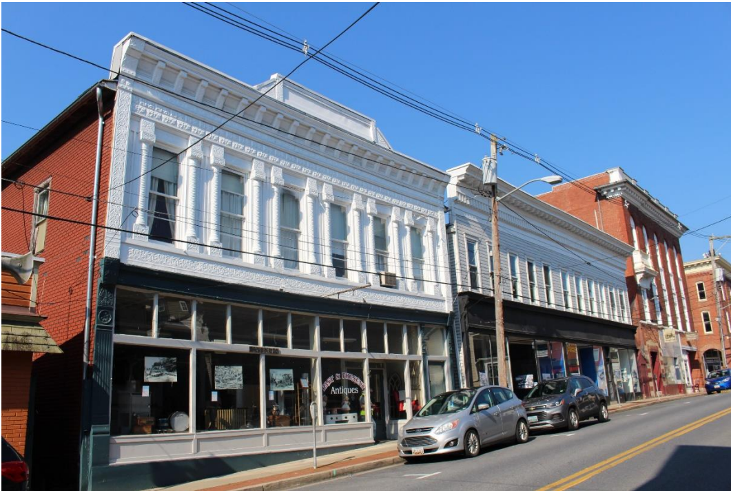
Photo 17 of 34: MD_FrederickCounty_BrunswickHD(Addl Doc)_017.tif Masonry Commercial Buildings on West Potomac Street, facing southwest
