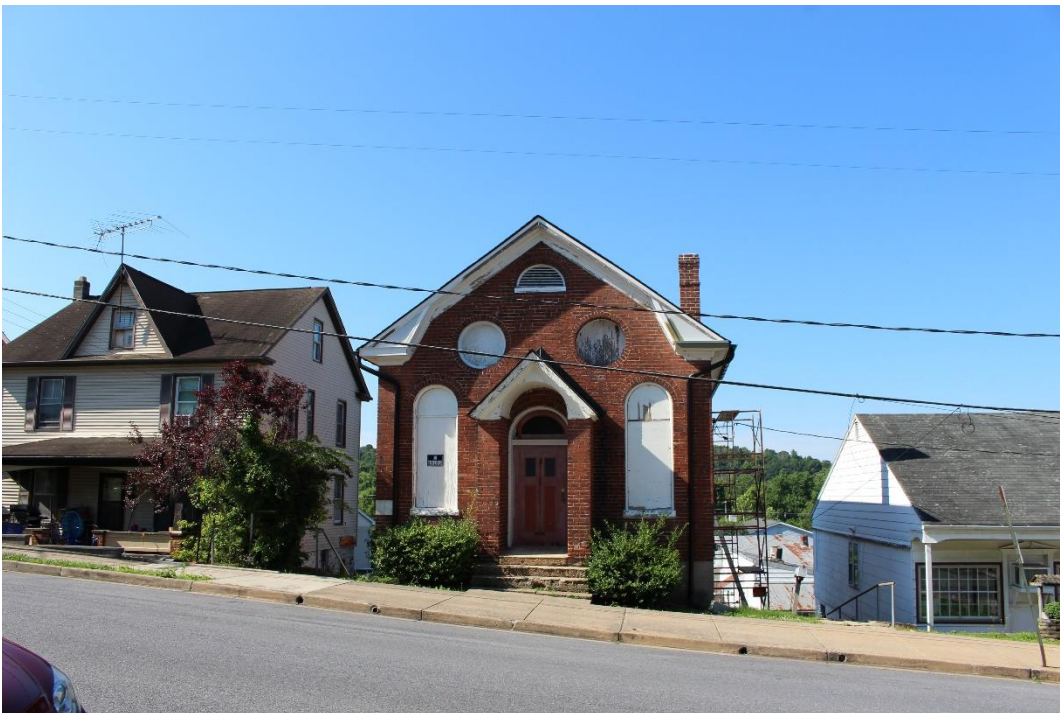
Photo 28 of 34: MD_FrederickCounty_BrunswickHD(Addl Doc)_028.tif Beth Israel Synagogue 14 East A Street, facing northeast
