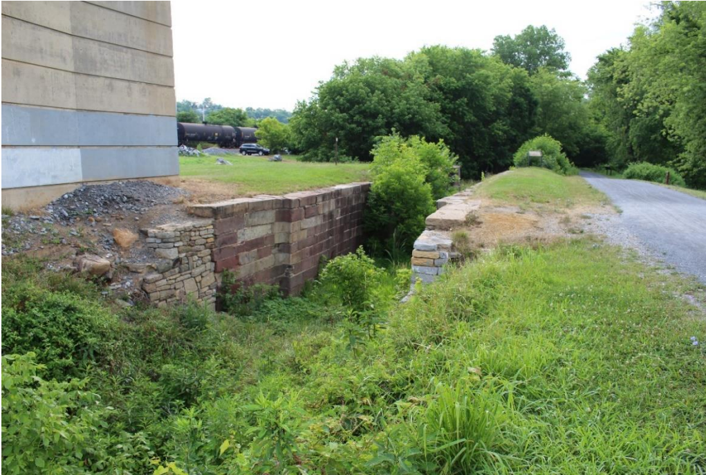
Photo 31 of 34: MD_FrederickCounty_BrunswickHD(Addl Doc)_031.tif C&O Canal, Lock 30, facing east
