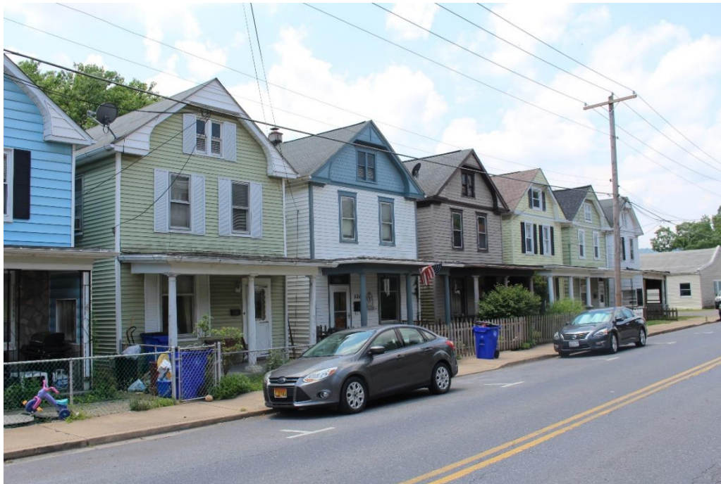
Photo 4 of 34: MD_FrederickCounty_BrunswickHD(Addl Doc)_004.tif B&O Worker Housing 526-536 West Potomac Street, facing southwest
