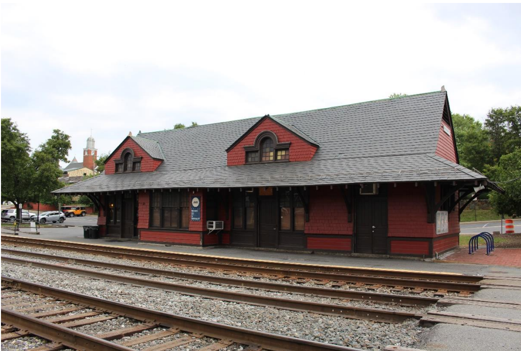
Photo 34 of 34: MD_FrederickCounty_BrunswickHD(Addl Doc)_034.tif B&O Passenger Station, facing northwest
