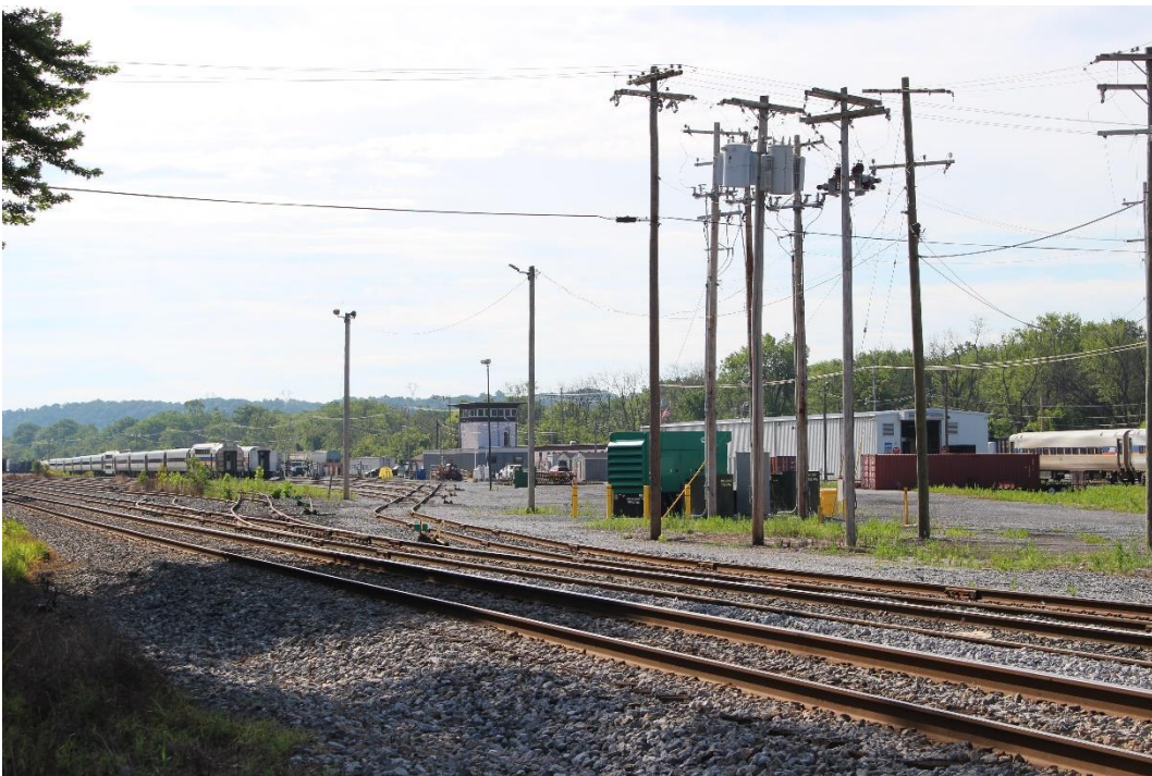
Photo 32 of 34: MD_FrederickCounty_BrunswickHD(Addl Doc)_032.tif B&O Freight Yard, facing southeast
