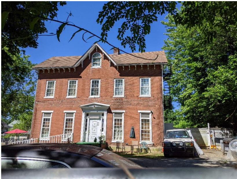
33 of 36: MD_BaltimoreCity_ParkHeightsHD_0124.tif 2900 Boarman Avenue, camera facing southwest
