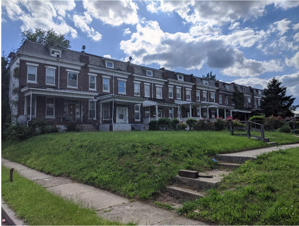
21 of 36: MD_BaltimoreCity_ParkHeightsHD_0051.tif 5000-5016 Denmore Avenue, camera facing west
