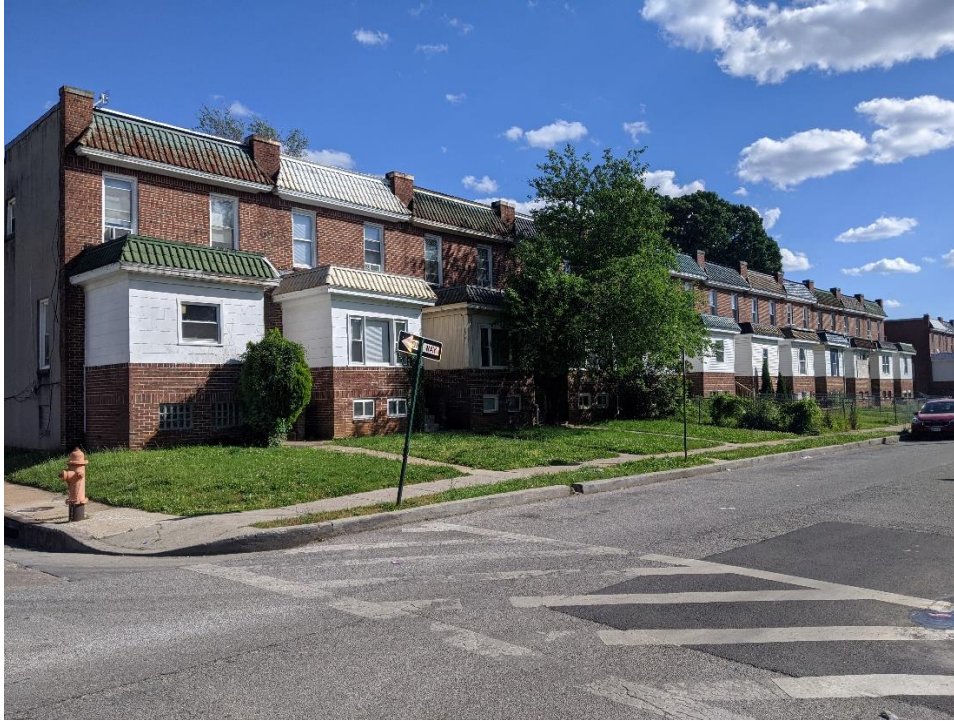
23 of 36: MD_BaltimoreCity_ParkHeightsHD_0059.tif 3901-3923 W. Garrison Avenue, camera facing south
