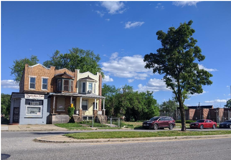
24 of 36: MD_BaltimoreCity_ParkHeightsHD_0066.tif 3701-3705 W. Belvedere Avenue, camera facing south
