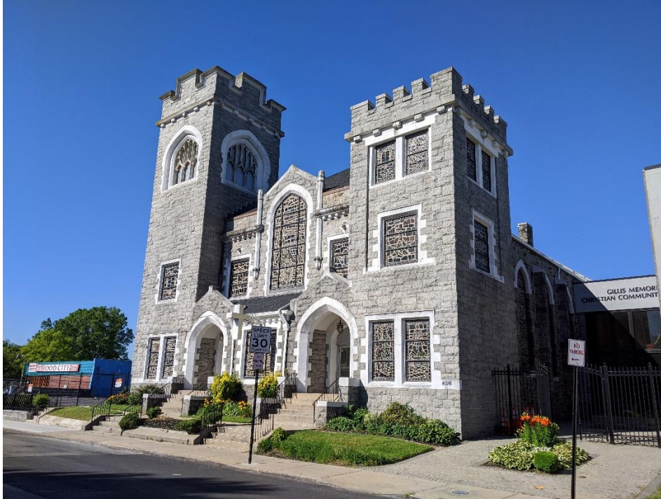
27 of 36: MD_BaltimoreCity_ParkHeightsHD_0092.tif 4016 Park Heights Avenue, camera facing south
