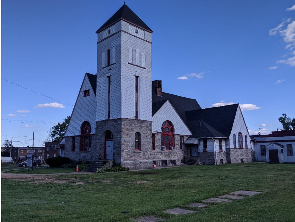
25 of 36: MD_BaltimoreCity_ParkHeightsHD_0069.tif 4820 Reisterstown Road, camera facing southeast
