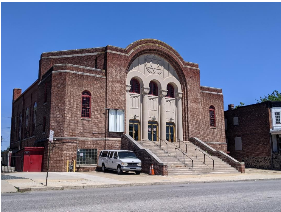
28 of 36: MD_BaltimoreCity_ParkHeightsHD_0095.tif 4239 Park Heights Avenue, camera facing east
