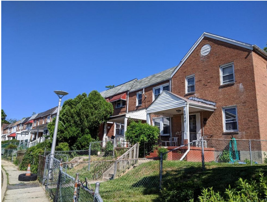
31 of 36: MD_BaltimoreCity_ParkHeightsHD_0109.tif 2900-2930 Oakford Avenue, camera facing northwest
