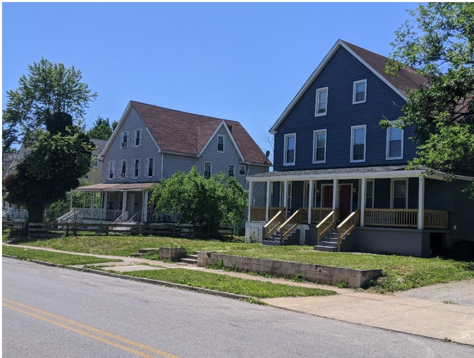
36 of 36: MD_BaltimoreCity_ParkHeightsHD_0161.tif 3514-3520 Hayward Avenue, camera facing west
