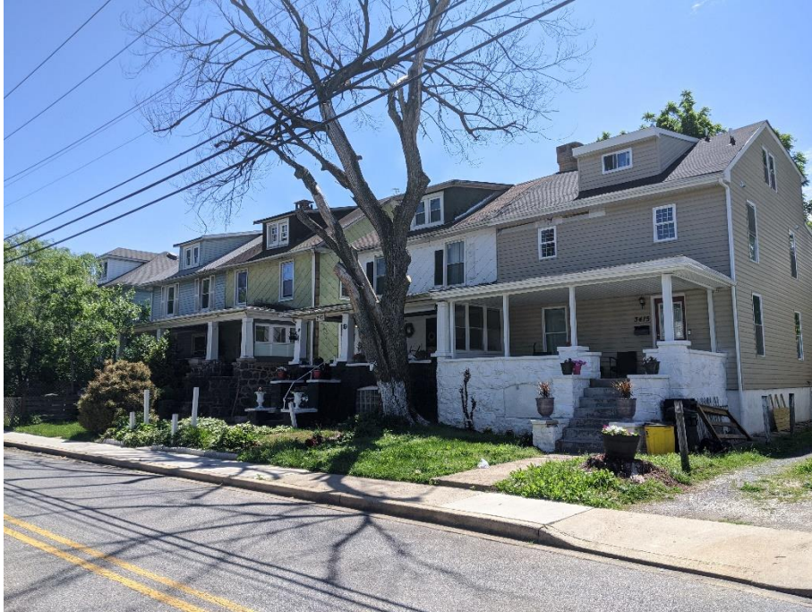
3 of 36: MD_BaltimoreCity_ParkHeightsHD_0004.tif 3409-3415 W. Rogers Avenue, camera facing east
