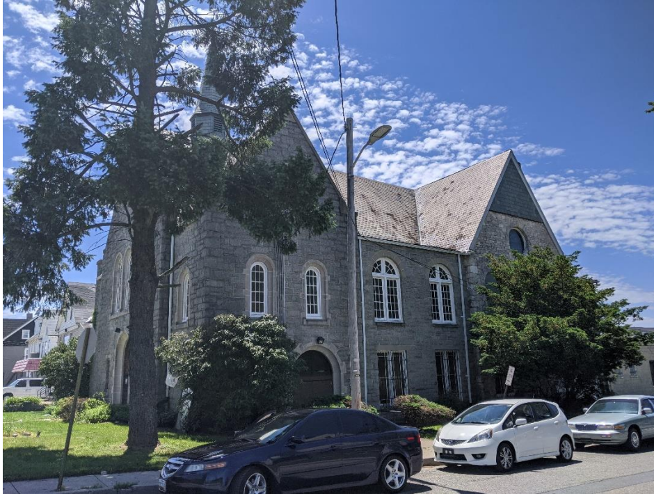
9 of 36: MD_BaltimoreCity_ParkHeightsHD_0021.tif 5260 Reisterstown Road, Arlington Methodist Church, view from McKendree Place
