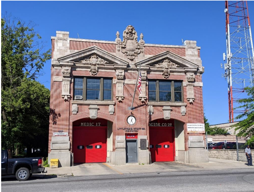
29 of 36: MD_BaltimoreCity_ParkHeightsHD_0096.tif 4312 Park Heights Avenue, camera facing west
