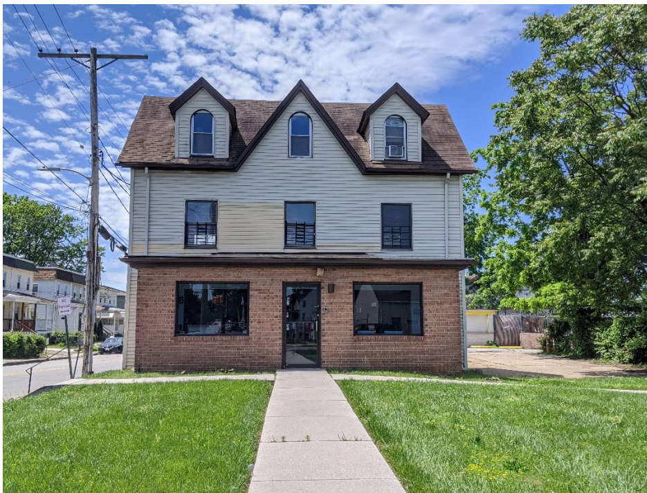
8 of 36: MD_BaltimoreCity_ParkHeightsHD_0018.tif 5300 Reisterstown Road, westside sunporch
