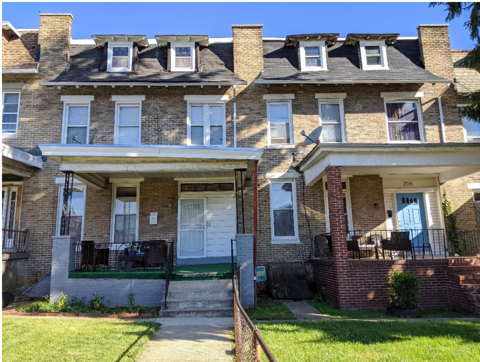
26 of 36: MD_BaltimoreCity_ParkHeightsHD_0082.tif 2506-2508 Keyworth Avenue, camera facing northwest
