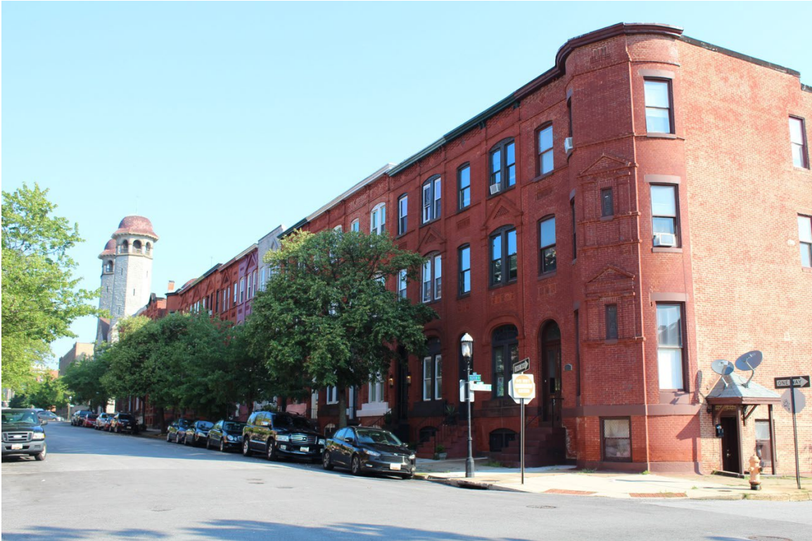
Photo 3 of 10 MD_BaltimoreCity_CivilRightsMPS_ParrenMitchellHouse_0003.tif 1800 block of Madison Avenue, southwest elevations, facing northeast
