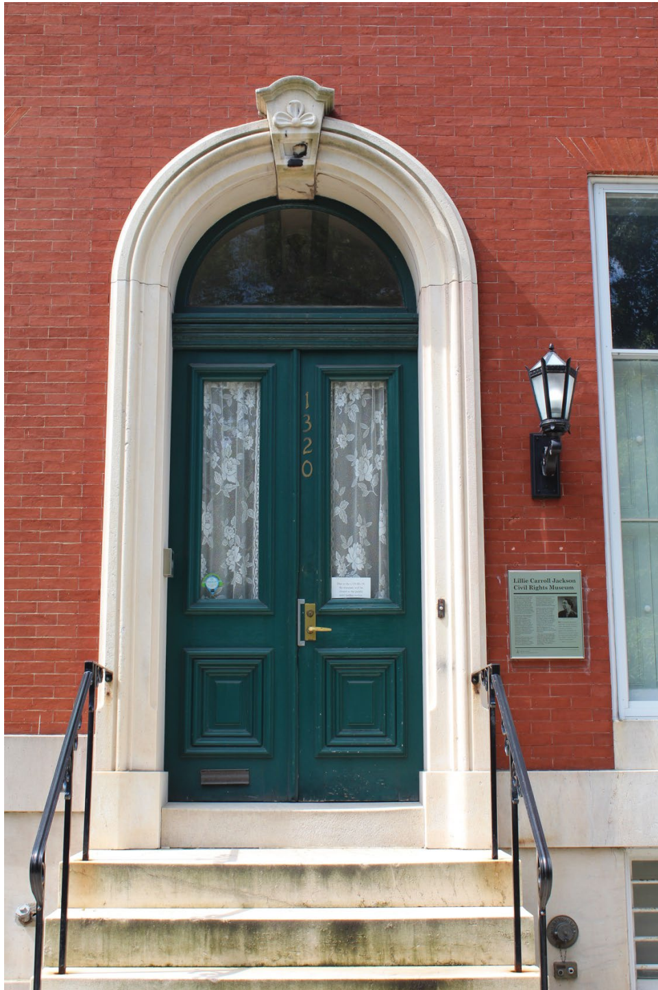
Photo 2 of 20 Detail of front entrance, facing northwest
