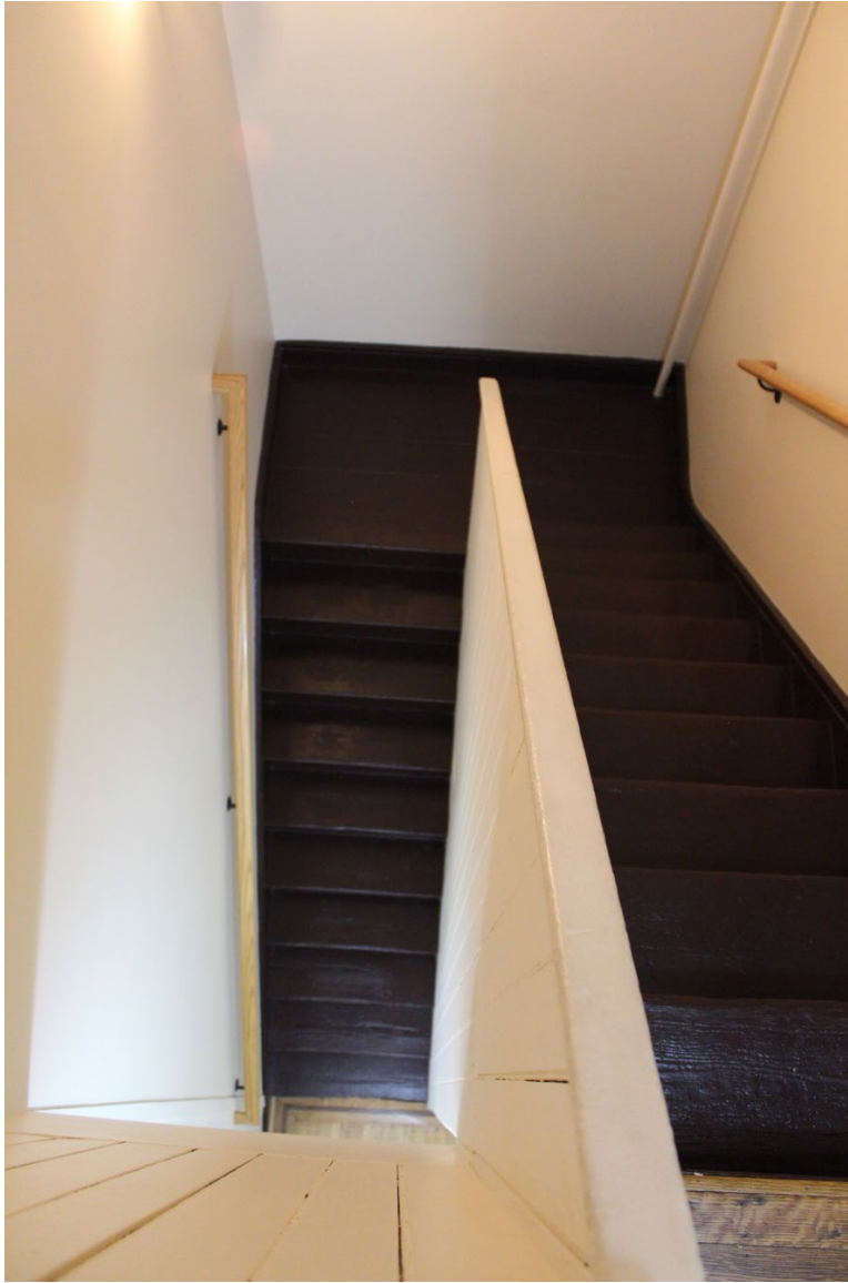
Photo 20 of 20 Servants' stair, looking down from third story to second story.
