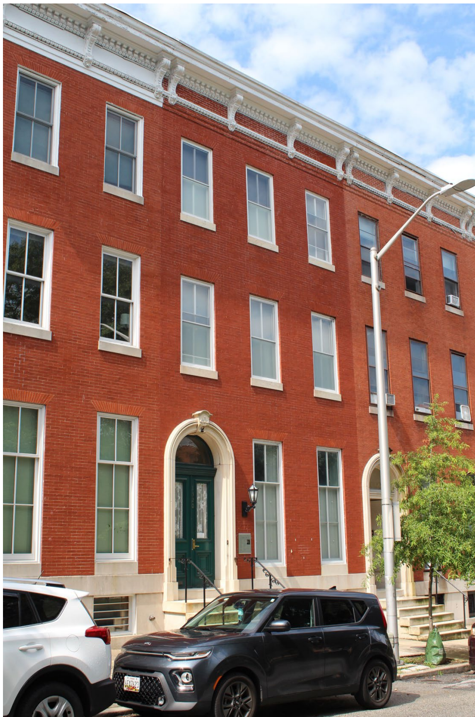
Photo 1 of 20 Northeast façade, facing northwest.
