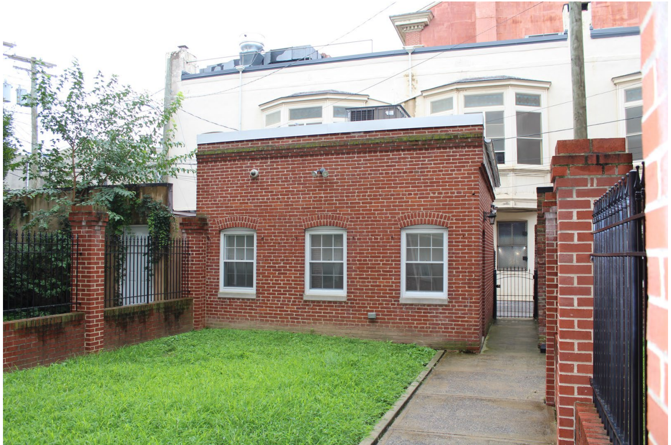
Photo 4 of 20 Northeast elevation of garage, looking southwest
