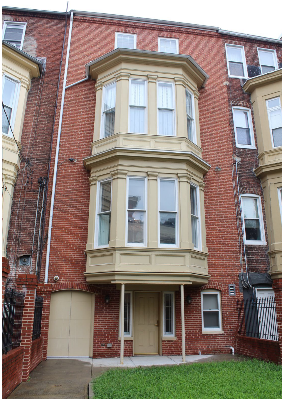
Photo 3 of 20 Southwest elevation, looking northeast
