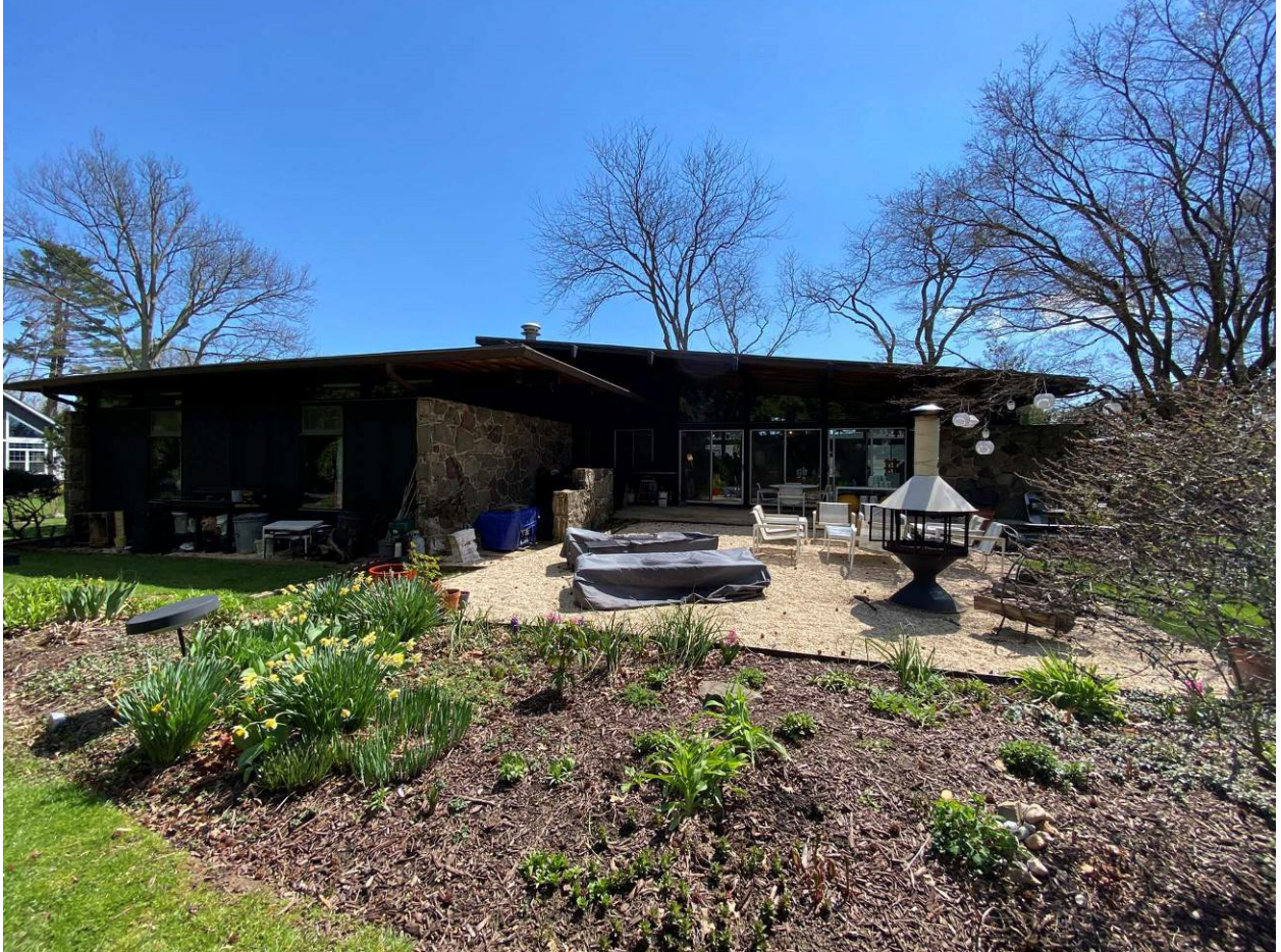
Photo #6 MD_Harford County_Hirsch Residence_0006 north elevation, looking south
