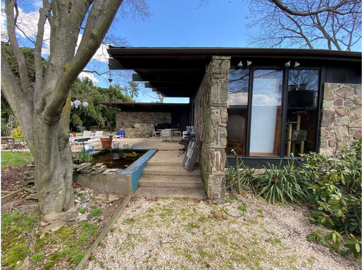
Photo #8 MD_Harford County_Hirsch Residence_0008 west elevation, looking east
