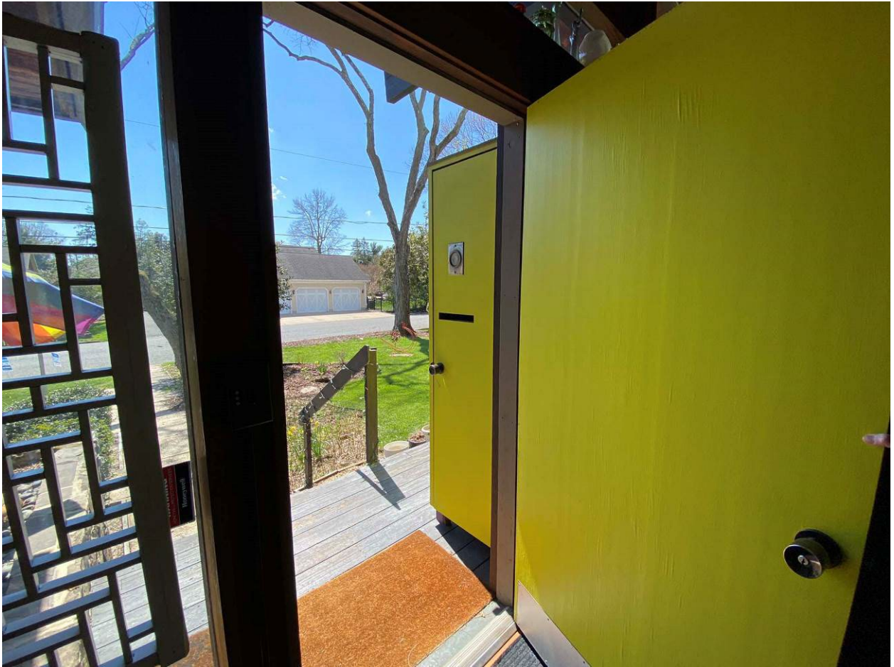
Photo #11 MD_Harford County_Hirsch Residence_0011 inside front entrance, looking southwest
