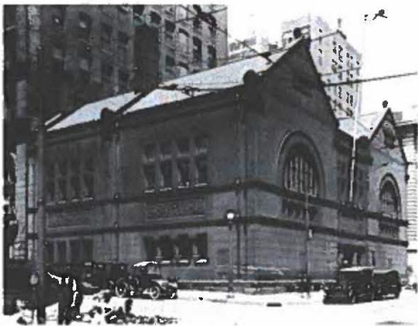
Fig. 6A – Wyatt & Sperry’s Mercantile Trust in Baltimore In 1886 was one of the finest examples of the Richardsonian Romanesque.
