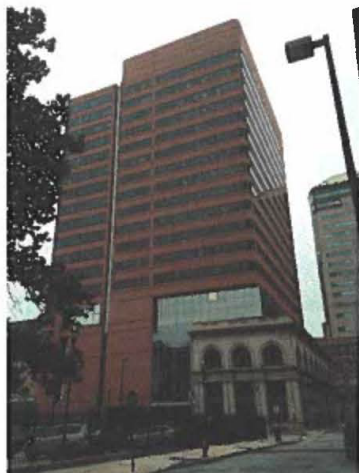
Fig. 25 – The thrift changed its name once more when it hit the $1 billion mark in 1979, and decided to build a new headquarters at East Lombard, Water, South, and Commerce Streets in 1983. This time the thrift chose the modern for its $30 million building but in a historic gesture, incorporated the 1894 Merchants’ National Building designed by Baldwin & Pennington. The cost of the new building played a role in the downfall of the thrift.
