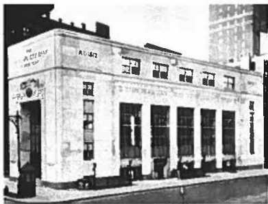
Fig. 13A – Beginning in the late 1920s, stripped or modern classicism replaced the classical Roman temple, Walker & Gillette’s National City Bank branch on Canal St. was the catalyst for the bank style that lasted up to World War II. The design elements would be repeated on National City’s branches to give the bank a brand identity.
