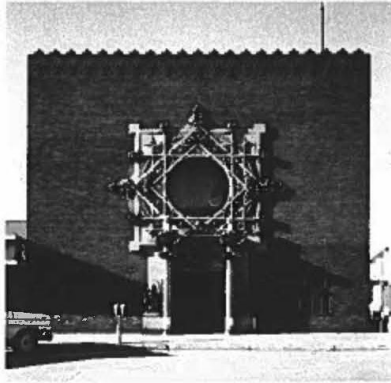
Fig. 10A – For sheer originality, Louis Sullivan may have been the most creative of all bank designers. Merchant’s National in Grinnell, Iowa in 1914 was one of 8 banks he did.
