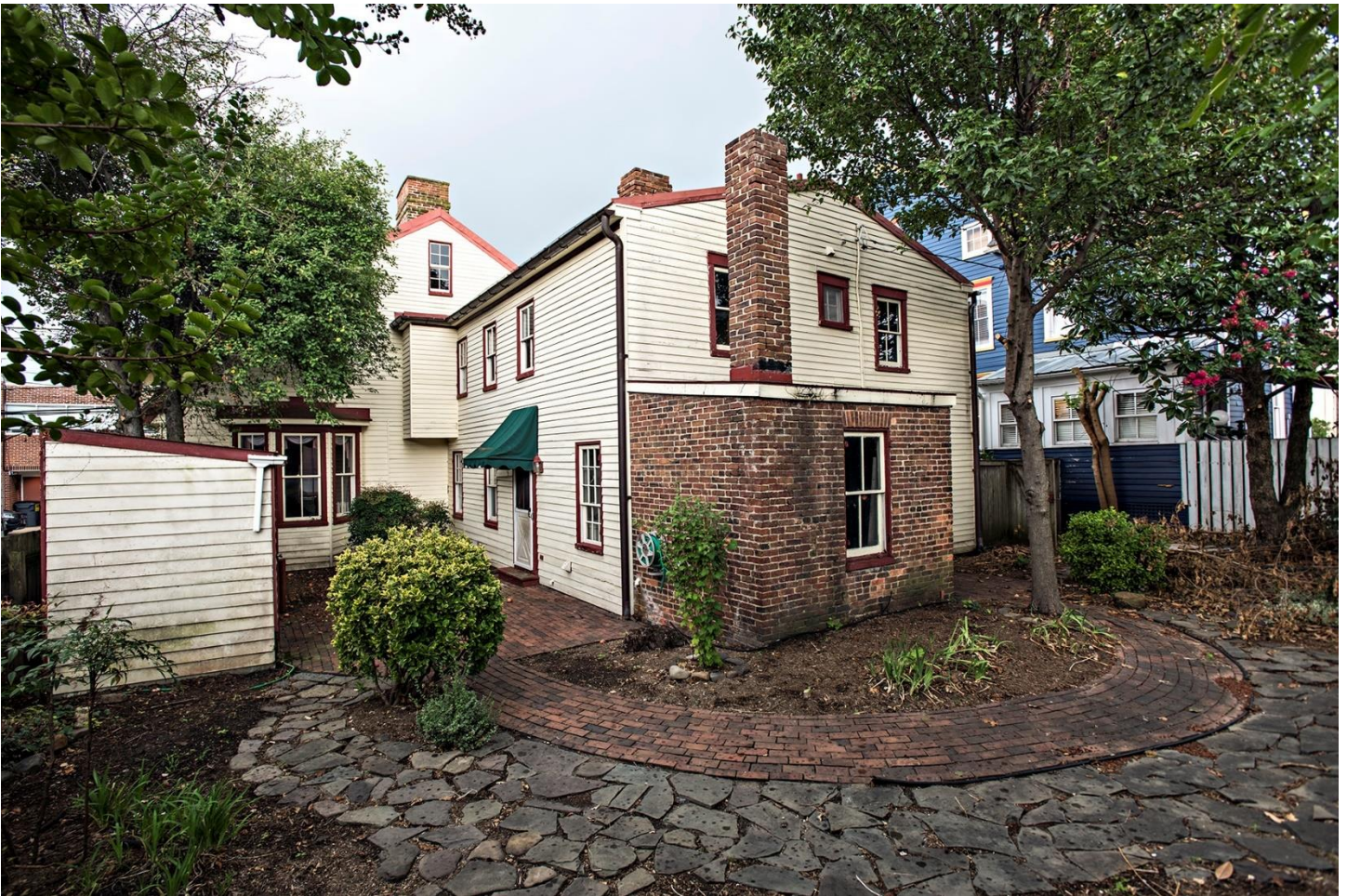
MD_AnneArundelCounty_SandsJohnHouse_0005.tif View from east
