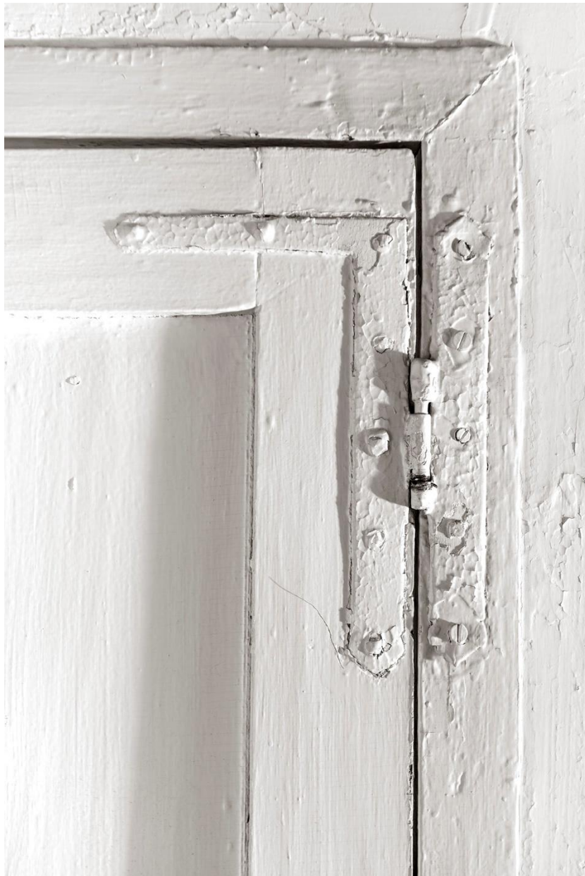
MD_AnneArundelCounty_SandsJohnHouse_0009.tif Handwrought hinge
