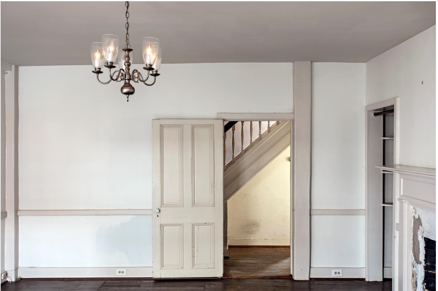
MD_AnneArundelCounty_SandsJohnHouse_0007.tif Showing articulated frame—exposed posts
