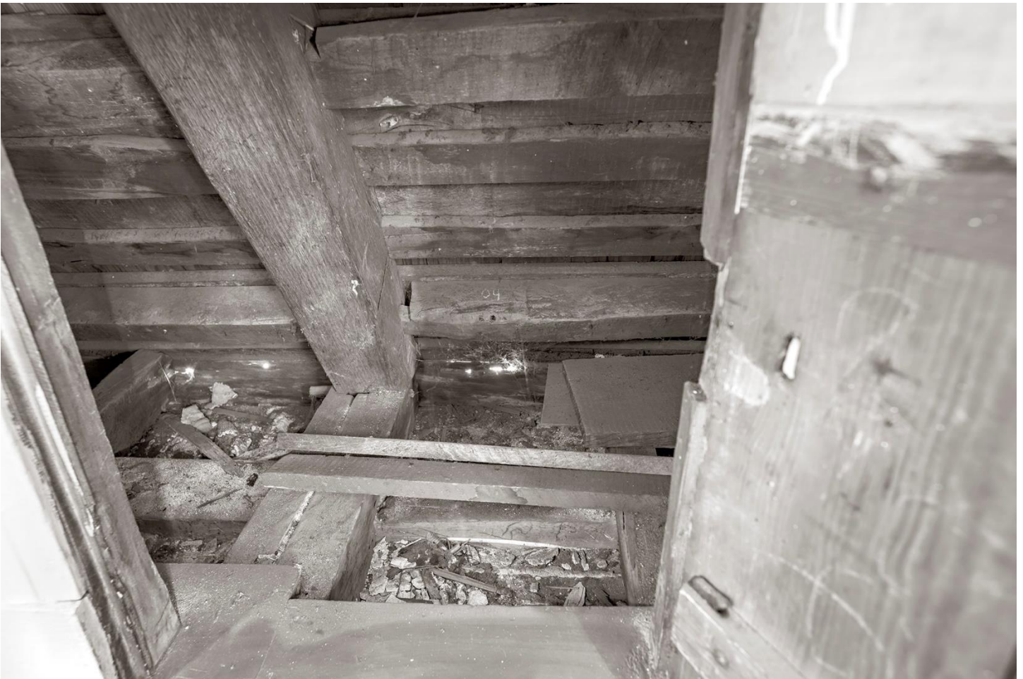
MD_AnneArundelCounty_SandsJohnHouse_0010.tif Foot of principal rafter showing complex joinery
