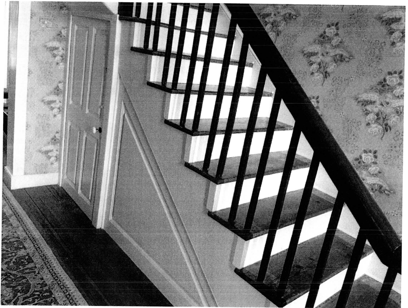
Photograph 4. Detail of staircase showing spandrel paneling, door to basement staircase, and steps looking toward second floor.
