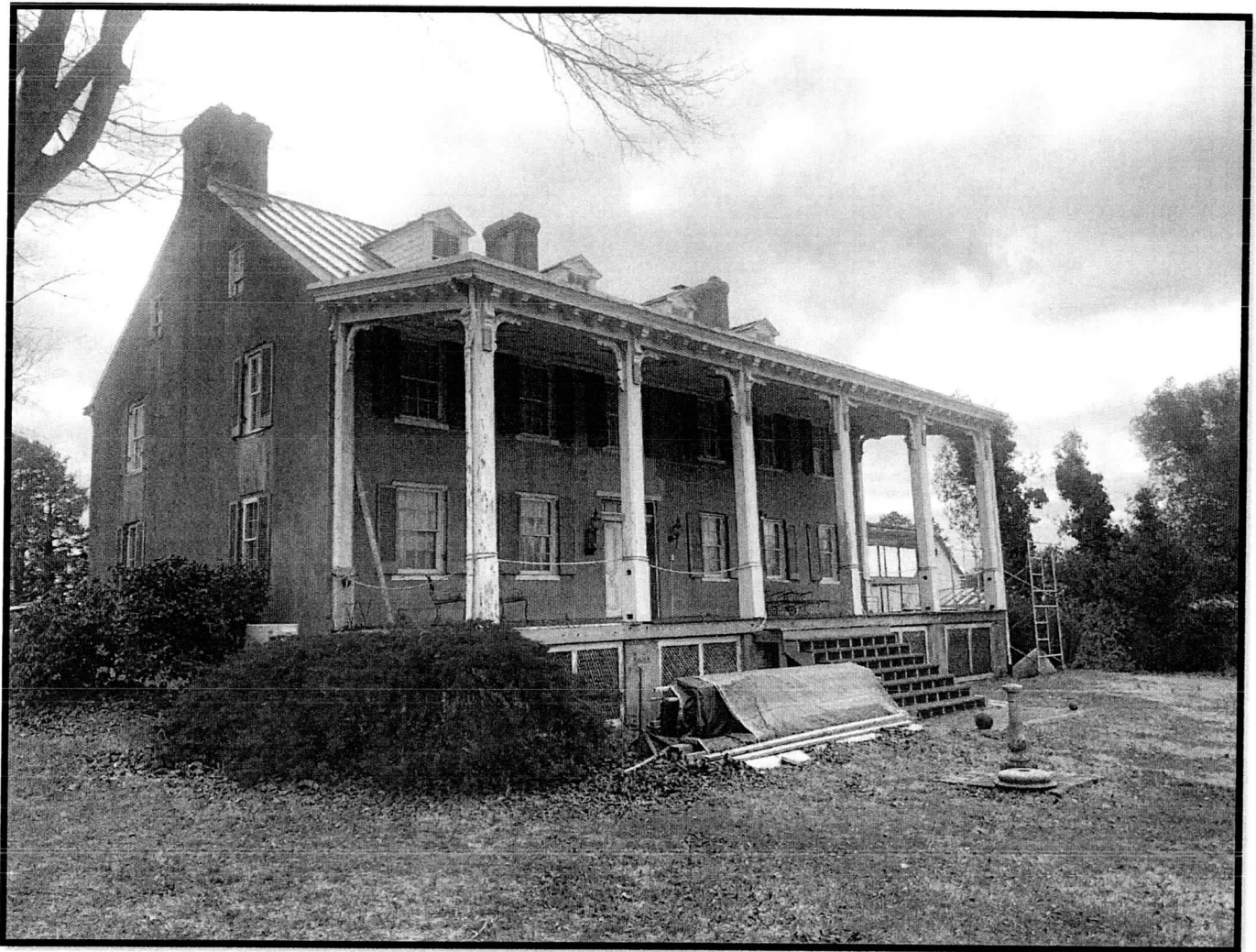
Photograph 1. North (river front) and east elevation looking southwesterly.
