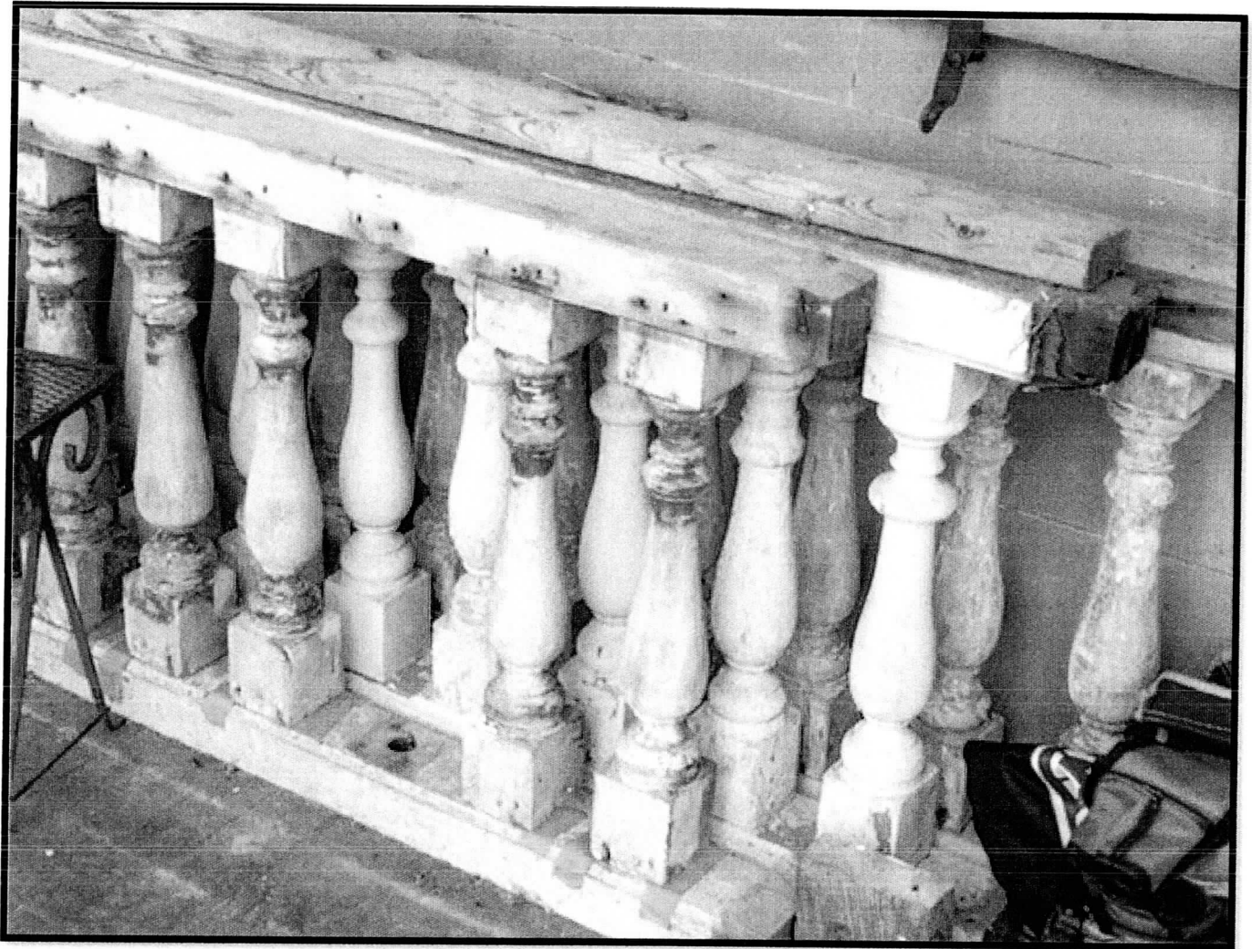
Photograph 16. Original portico balustrade sections being conserved and then reinstalled.
