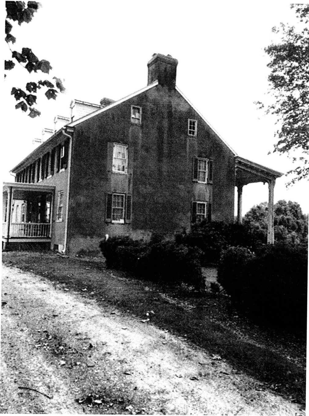
Photograph 2. East elevation looking westerly.
