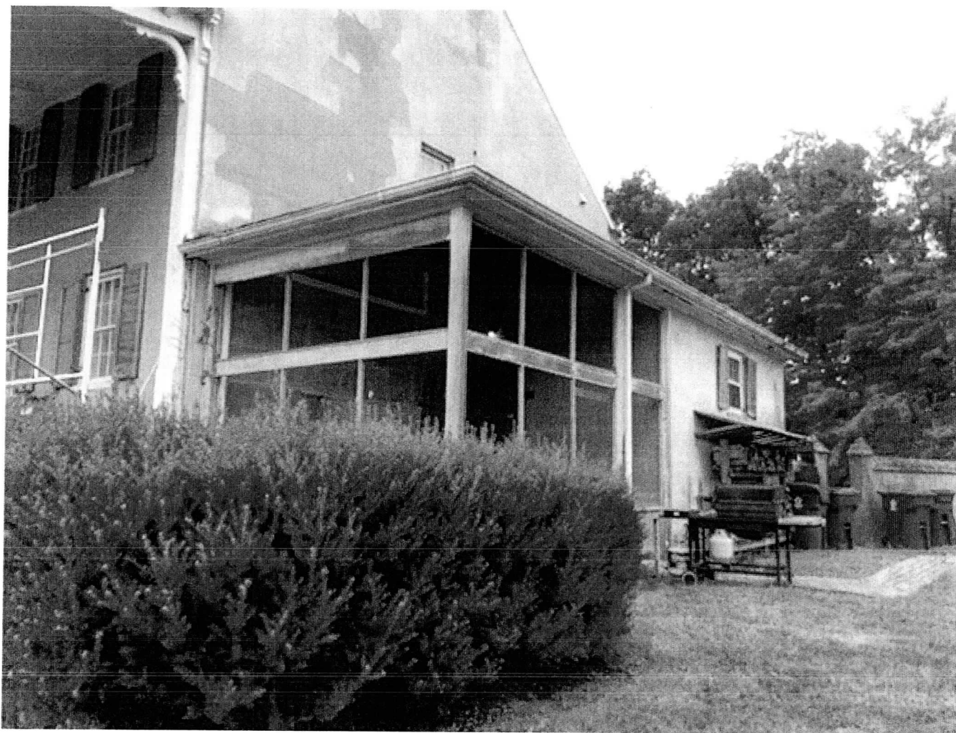
Photograph 11. 1951 breakfast room and porch addition to west side. Looking southeasterly.
