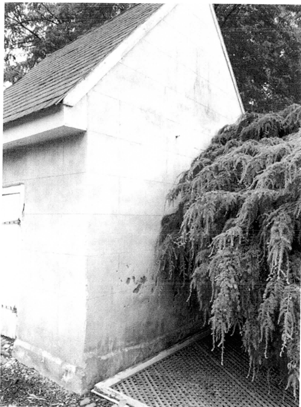
Photograph 12. Northwest corner of smokehouse looking southeasterly.
