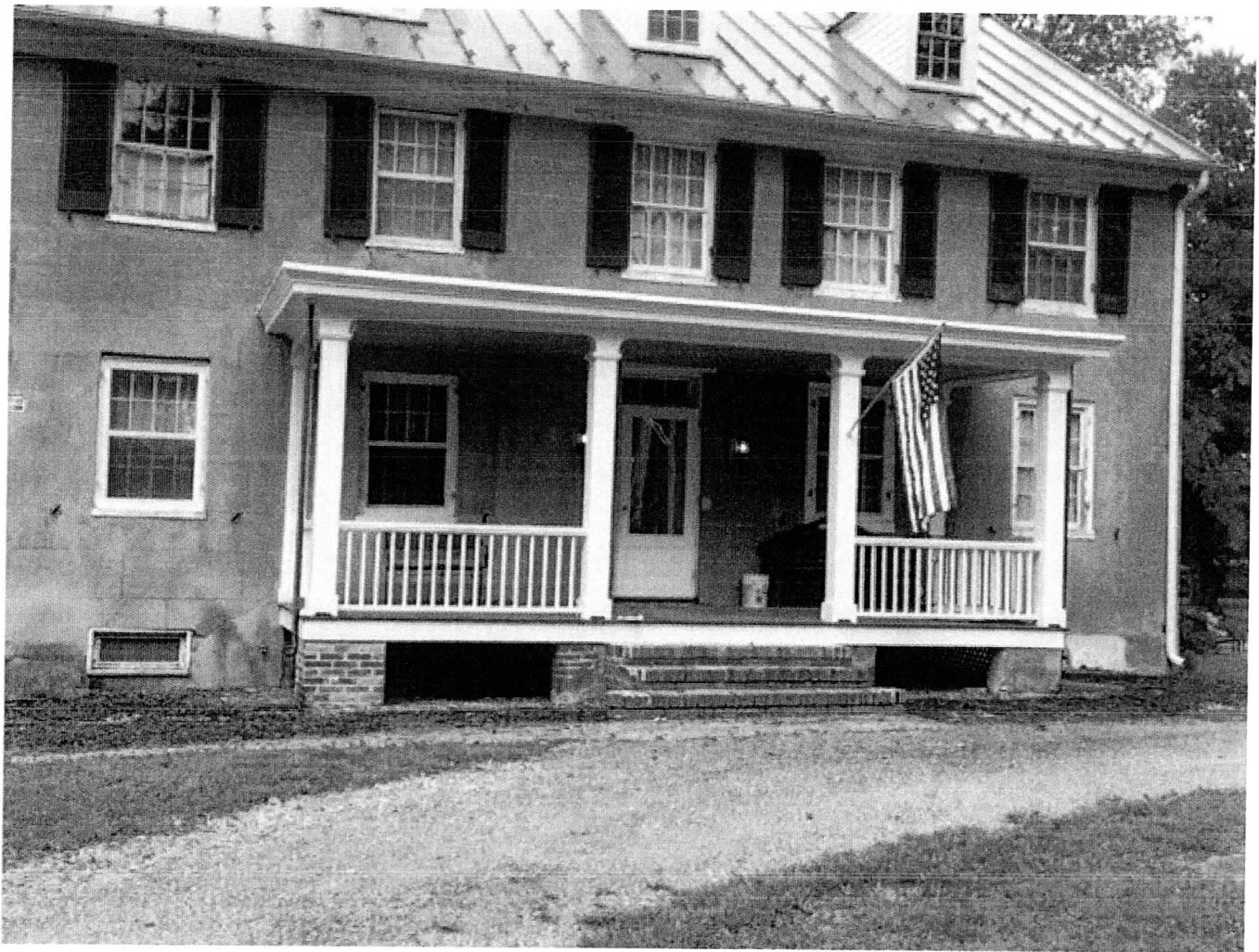
Photograph 10. 1864 porch on southerly elevation. Three bays to right are ca. 1773 section.
