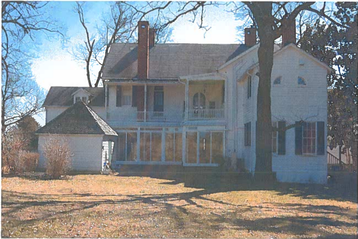
MD_FrederickCounty_Oakland_0002.tif Rear of house, camera facing south
