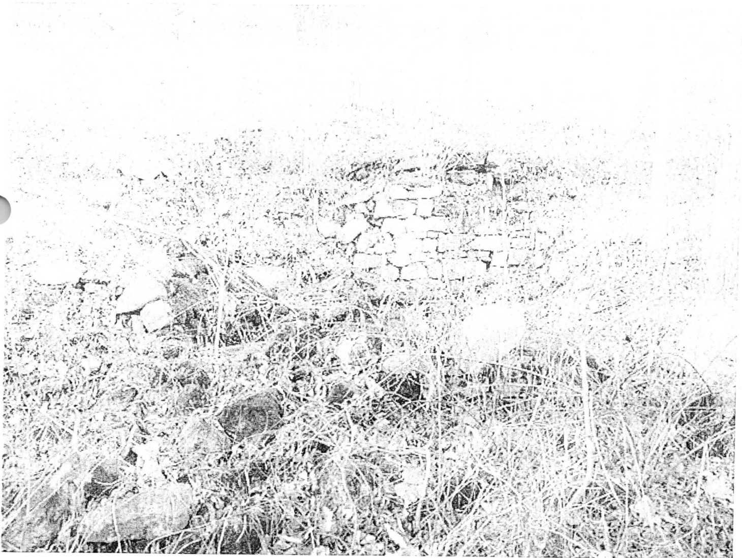
MD_WASHINGTONCOUNTY_COOLHOLLOWHOUSE_0007.TIF Mill site stone foundation, west.
