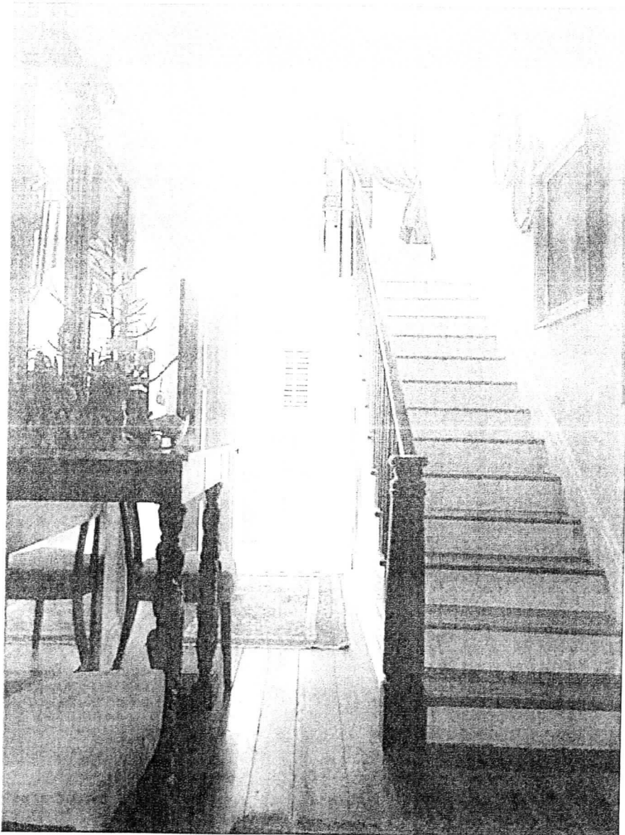
MD_WASHINGTONCOUNTY_COOLHOLLOWHOUSE_00018.TIF First floor stair and entrance hall, West.
