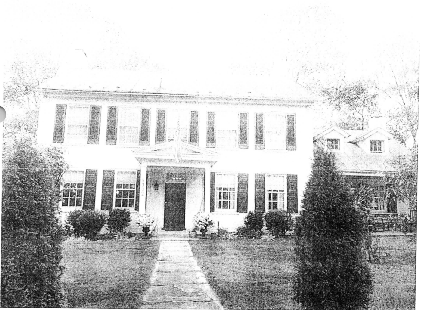
MD_WASHINGTONCOUNTY_COOLHOLLOWHOUSE_0001.TIF West View, East elevation facing the National Road
