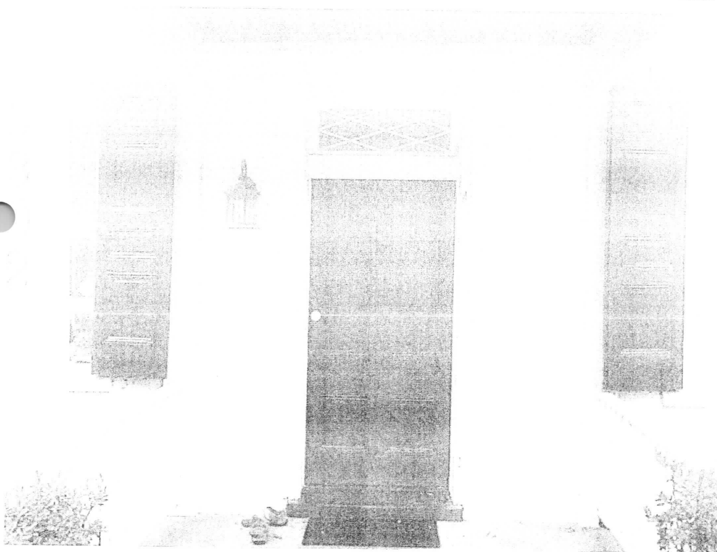
MD_WASHINGTONCOUNTY_COOLHOLLOWHOUSE_00017.TIF Front door, west view, east elevation.
