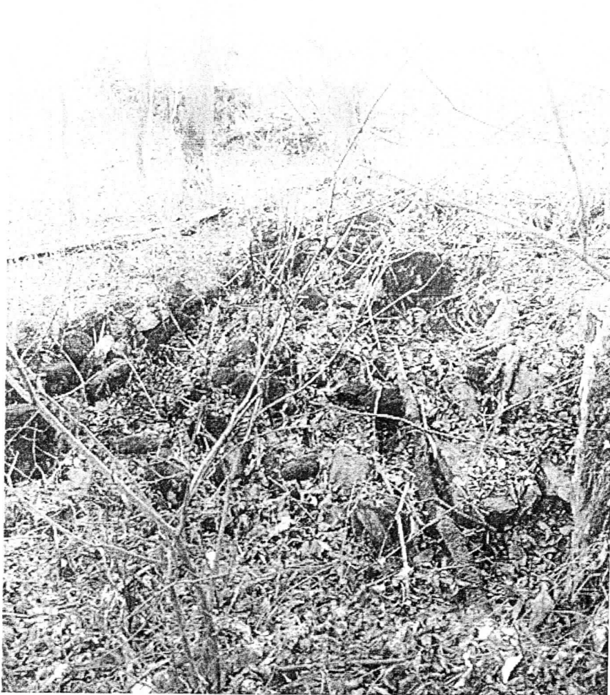
MD_WASHINGTONCOUNTY_COOLHOLLOWHOUSE_0008.TIF Mill site, stone foundation and wall, east.
