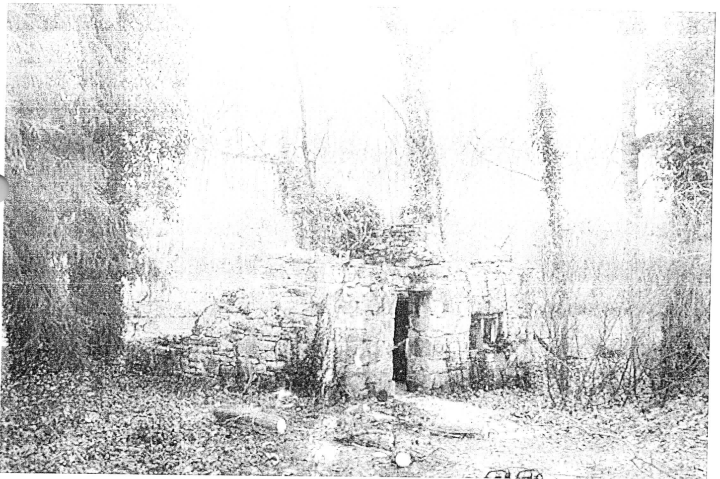
MD_WASHINGTONCOUNTY_COOLHOLLOWHOUSE_00011.TIF 18 th Century stone forge, northwest from lawn.
