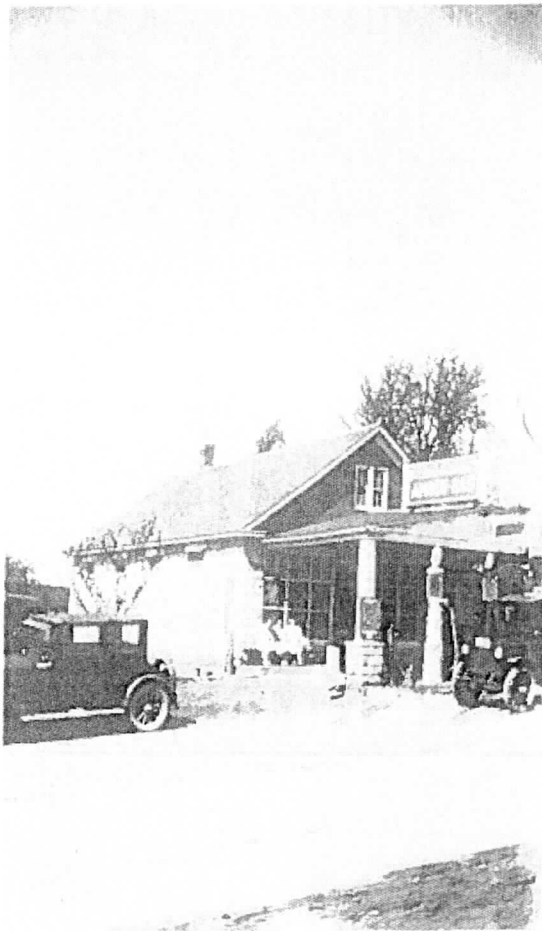
MD_FrederickCounty_Cockey'sHouseandStore_0046.tif Store (Hendrickson's Store) c. 1920-1930's, south (front) façade with Amoco gasoline pumps in front
