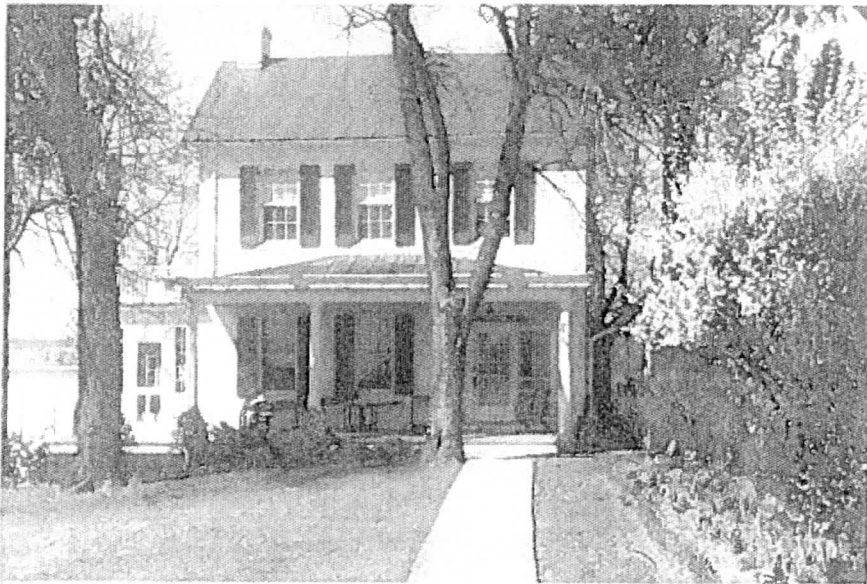
MD_FrederickCounty_Cockey'sHouseandStore_0041.tif Cockey Jamison/Hendrickson House (Hendrickson home) c.1940-1950's, south (front) elevation
