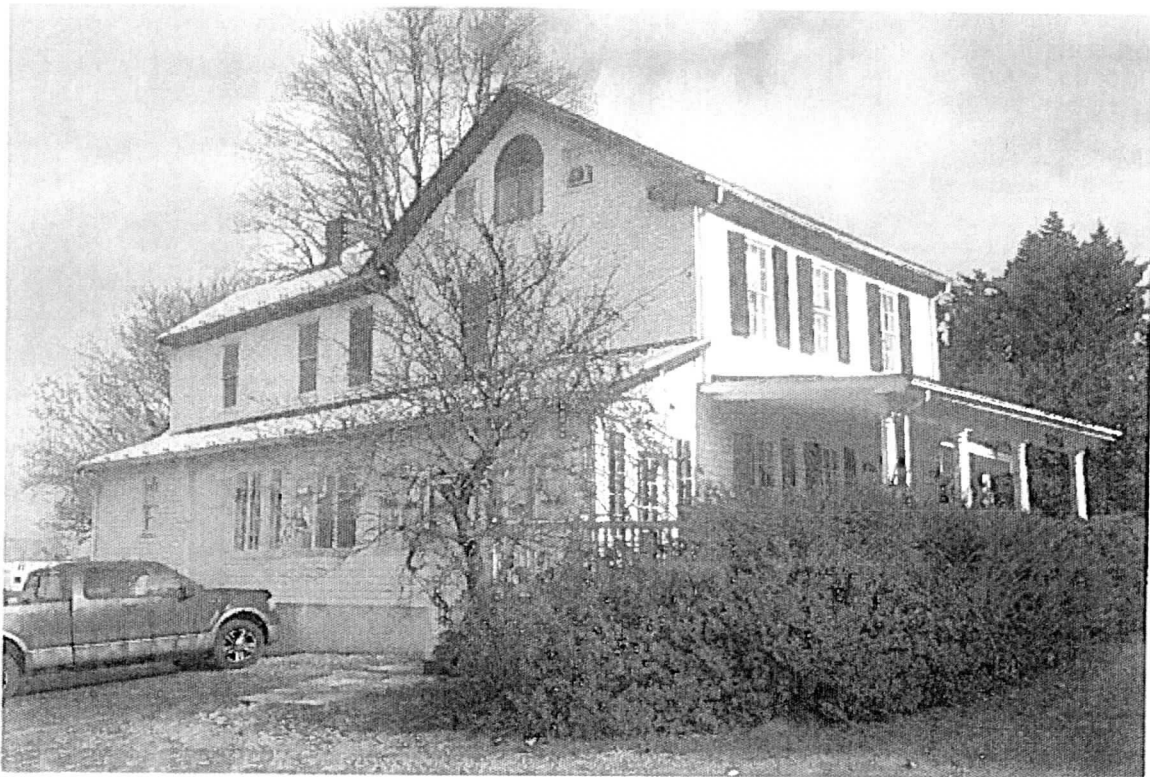
MD FrederickCounty_Cockey'sHouseandStore_0003.tif Cockey/Jamison/Hendrickson House, west side elevation
