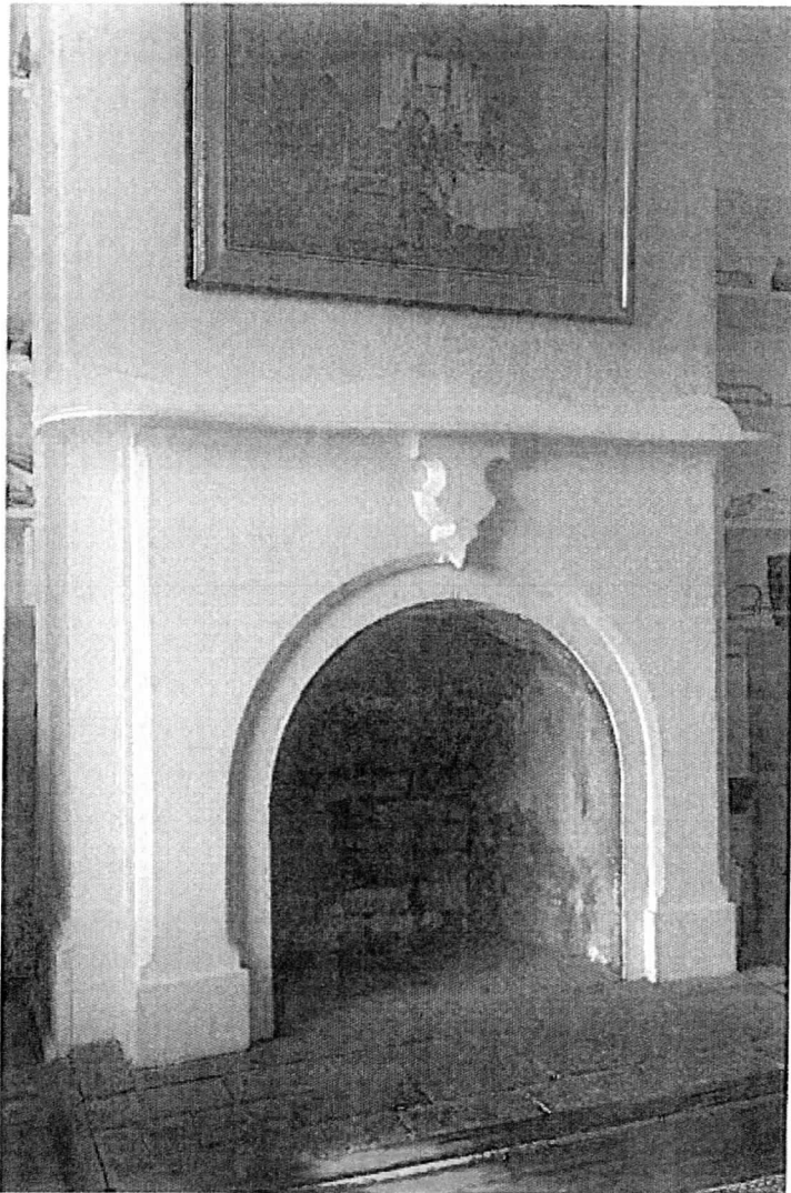
MD_FrederickCounty_Cockey'sHouseandStore_0021.tif Cockey/Jamison/Hendrickson House interior, front parlor, original fireplace and mantel
