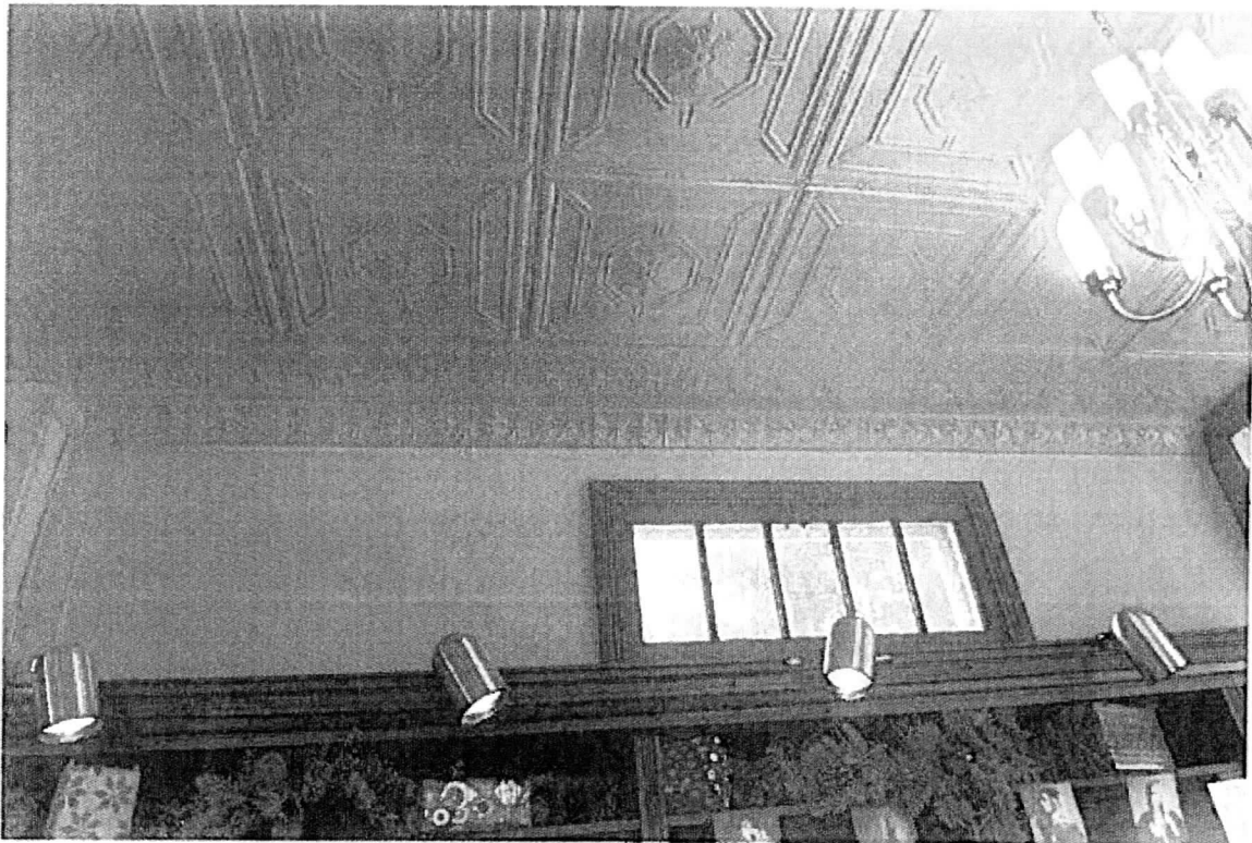
MD FrederickCounty_Cockey'sHouseandStore_0033.tif Store interior, original pressed metal ceiling
