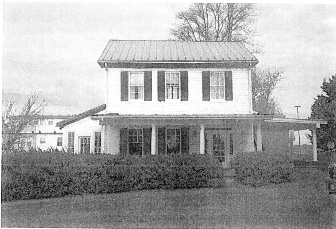
MD_FrederickCounty_Cockey'sHouseandStore_0002.tif Cockey/Jamison/Hendrickson House, south front elevation
