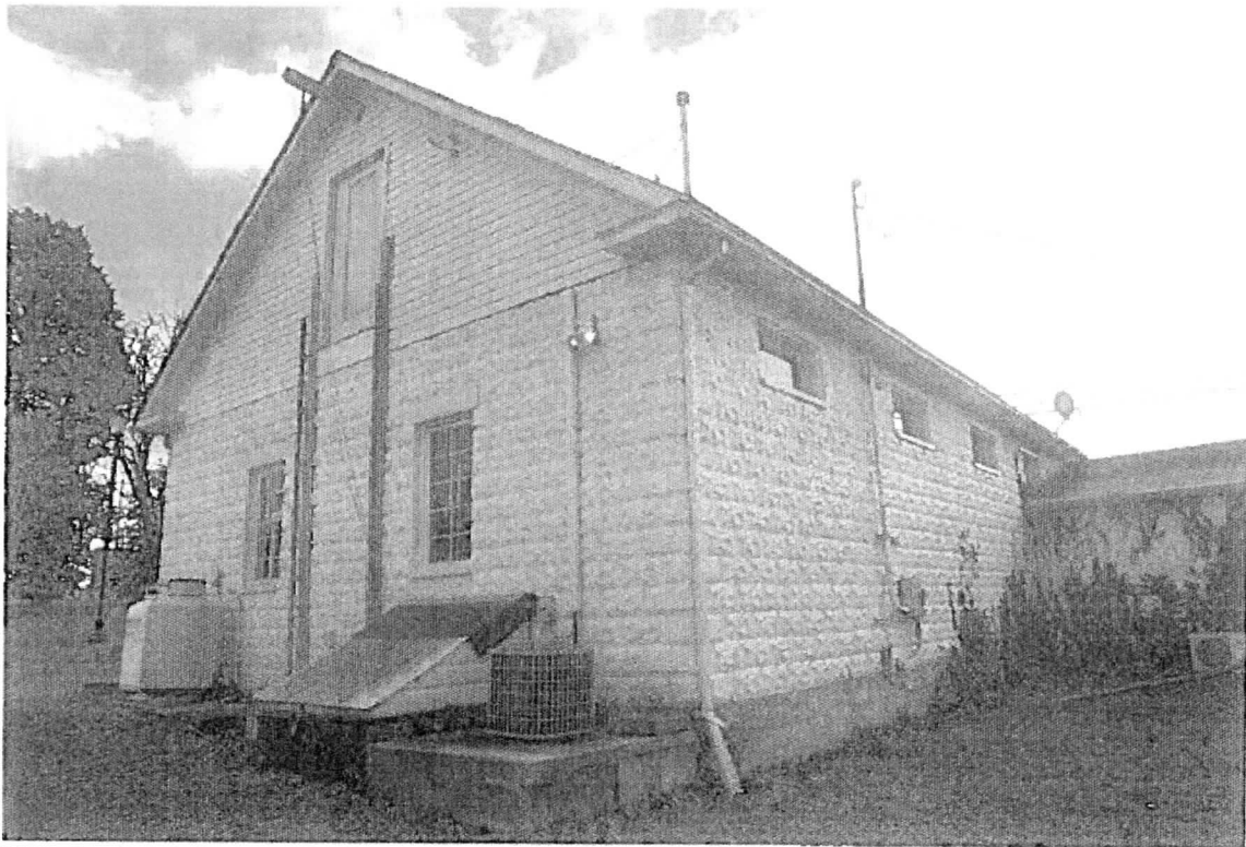
MD FrederickCounty Cockey'sHouseandStore_0012.tif Store, northwest corner of north and west facades
