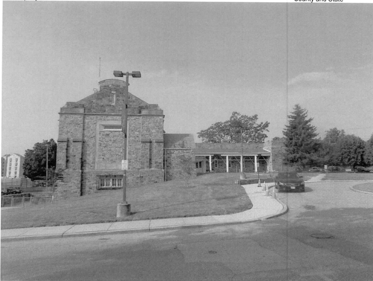
MD_BaltimoreCity_MSUMemorialChapel_0002.tif North Elevation, 06/29/2012 2 of _7_.
