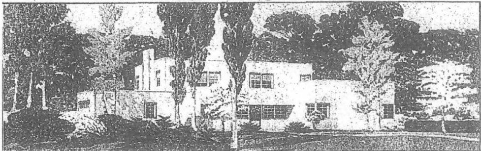
The first pre-fabricated motohome to be built in the Washington area is under construction on Brookside drive, in Kenwood, Chevy Chase, Md., for Lee D. Butler, prominent Washington automobile distributor. The house is built of prefabricated steel into which are set fireproof panels of compressed asbestos and cement, said to be indestructible. The house contains 12 rooms, 3 baths and a 2-car garage. A moto-unit, a mechanism no larger than a pantry, operates the air-conditioning, heating and hot water units. The above sketch is an artist's conception of what Mr. Butler's new home will look like when completed.
