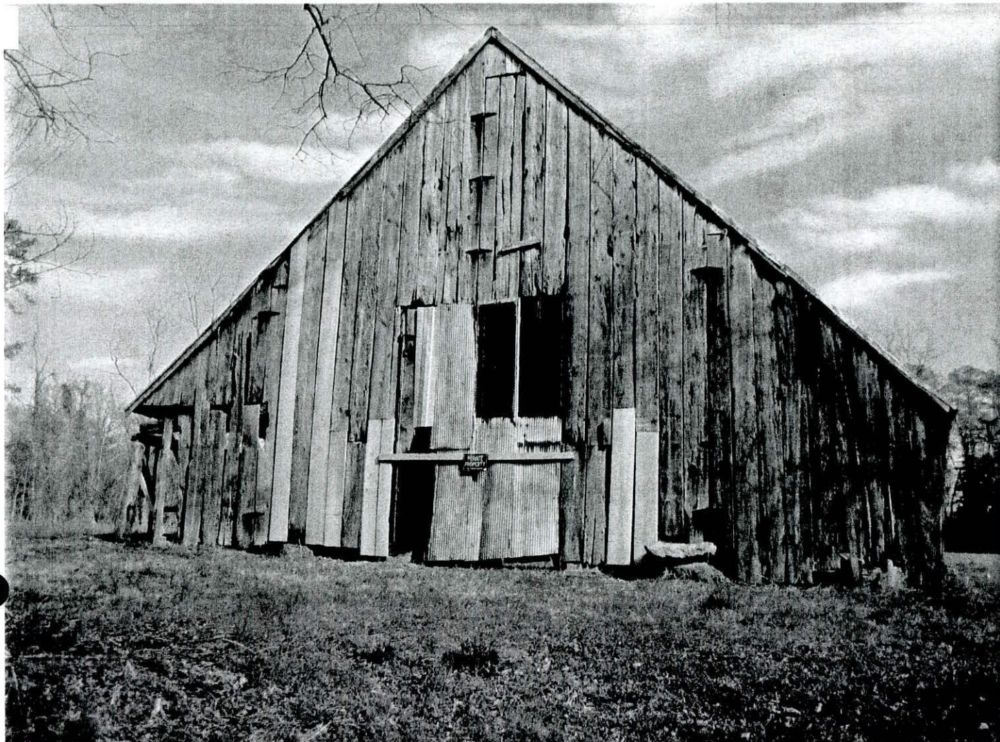
Barn exterior, view from west, 4/5/2014
