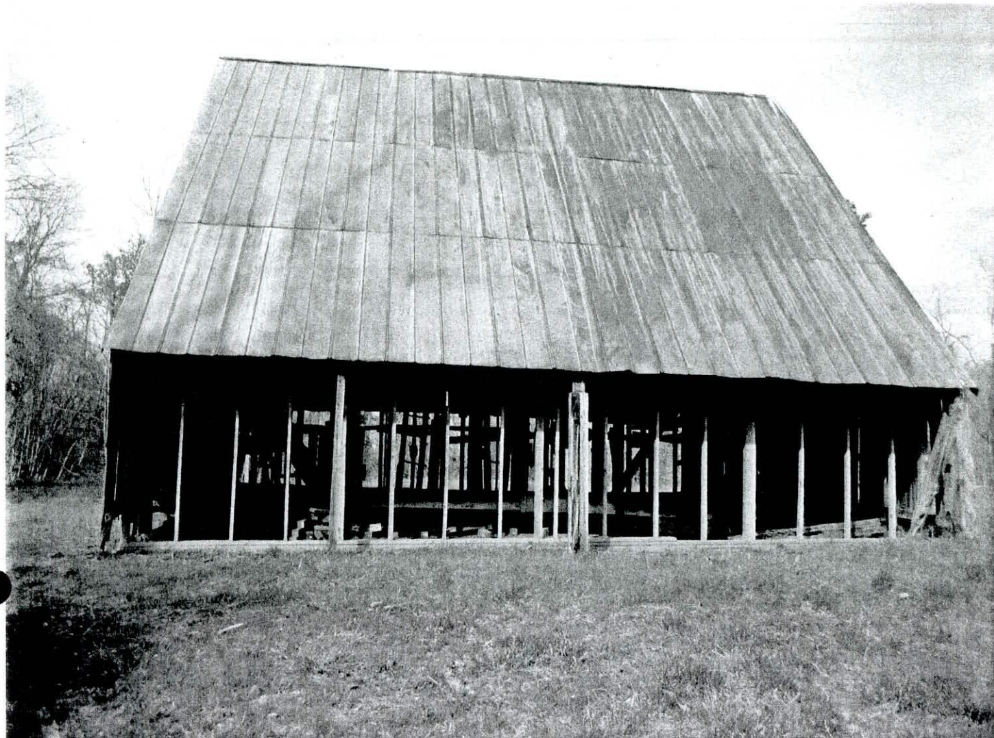
Barn exterior, view from south, 4/5/2014. Siding repair in progress.
