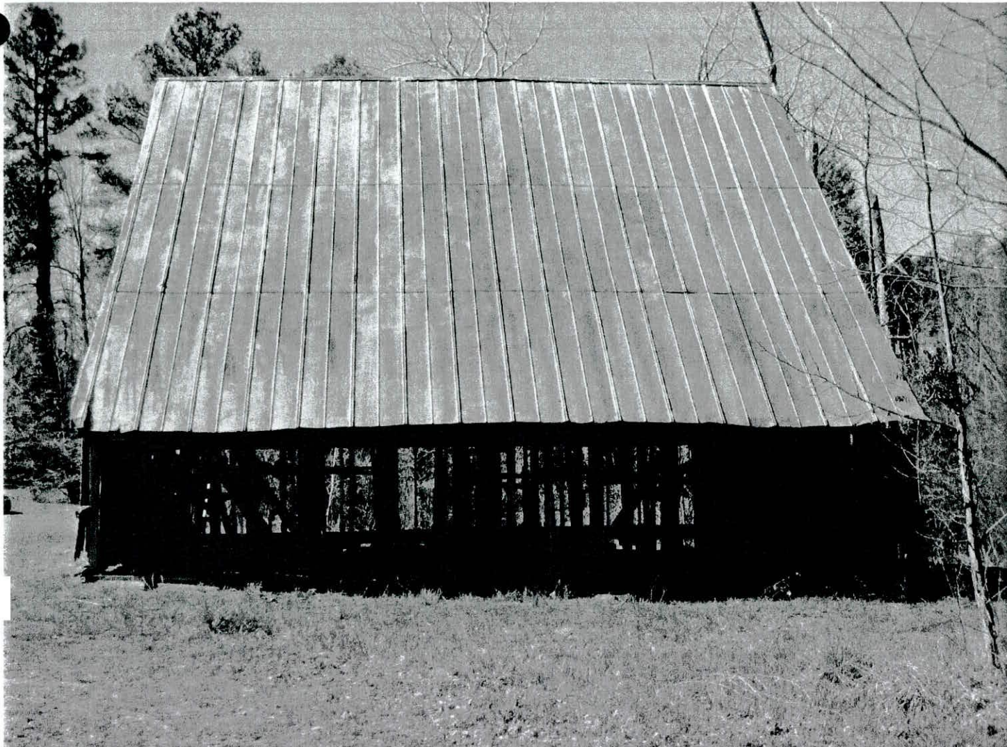
Barn exterior, view from north, 4/5/2014. Siding repair in progress.
