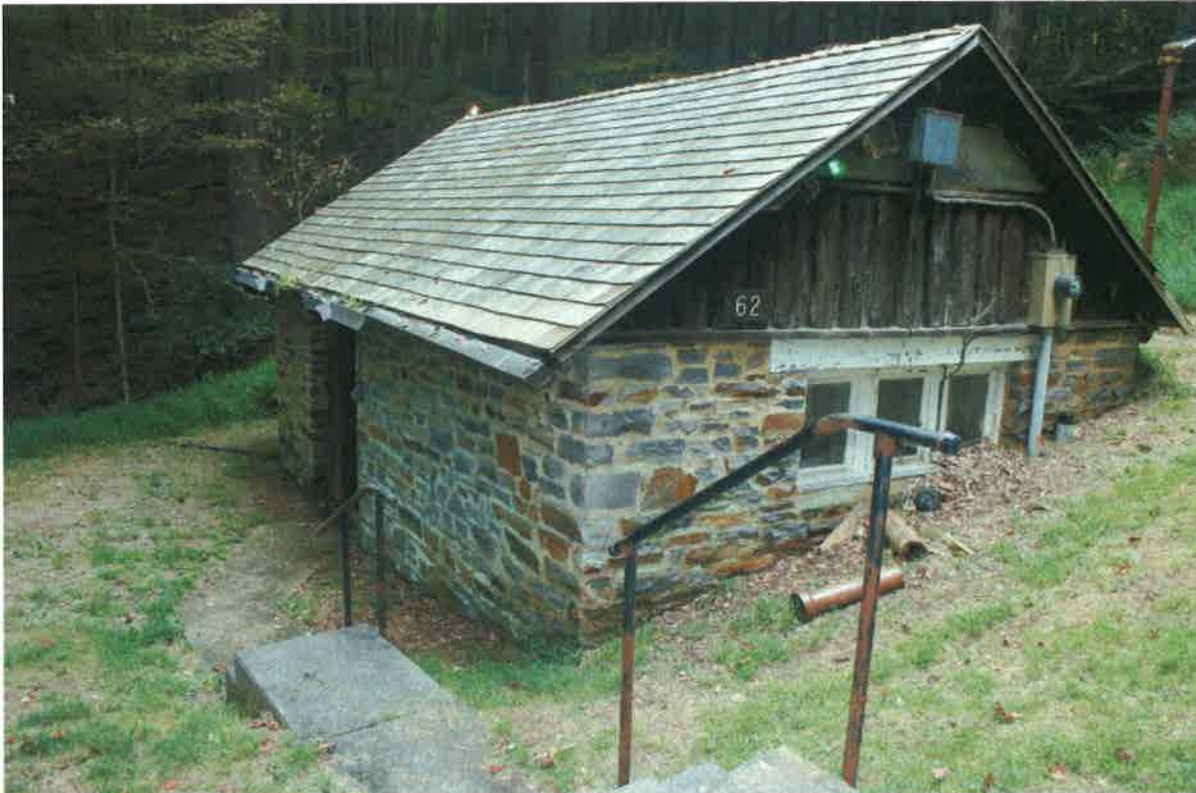
Photo 18 of 33 (MD_FrederickCounty_CatoctinMountainParkHD_0018)* Ike Smith Pumphouse (Bld 62, LCS# 231878) looking northeast.
