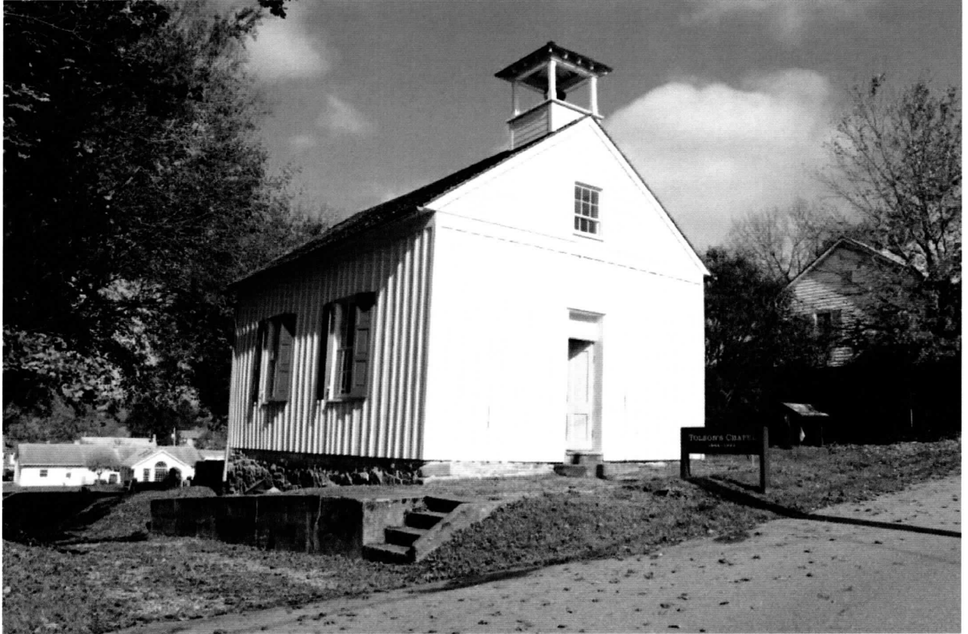
1 of 10 South and west elevations of church/school, looking northeast, showing west alley.
