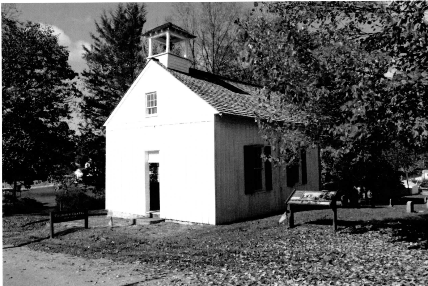
2 of 10 South and east elevations of church/school, looking northwest, showing southeast corner of cemetery.
