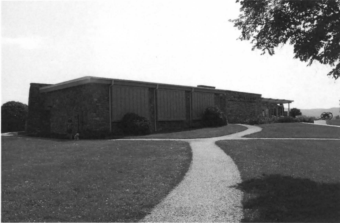
Photo 3 of 28. Visitor Center, West Elevation, Looking Southeast (8/4/2017)
