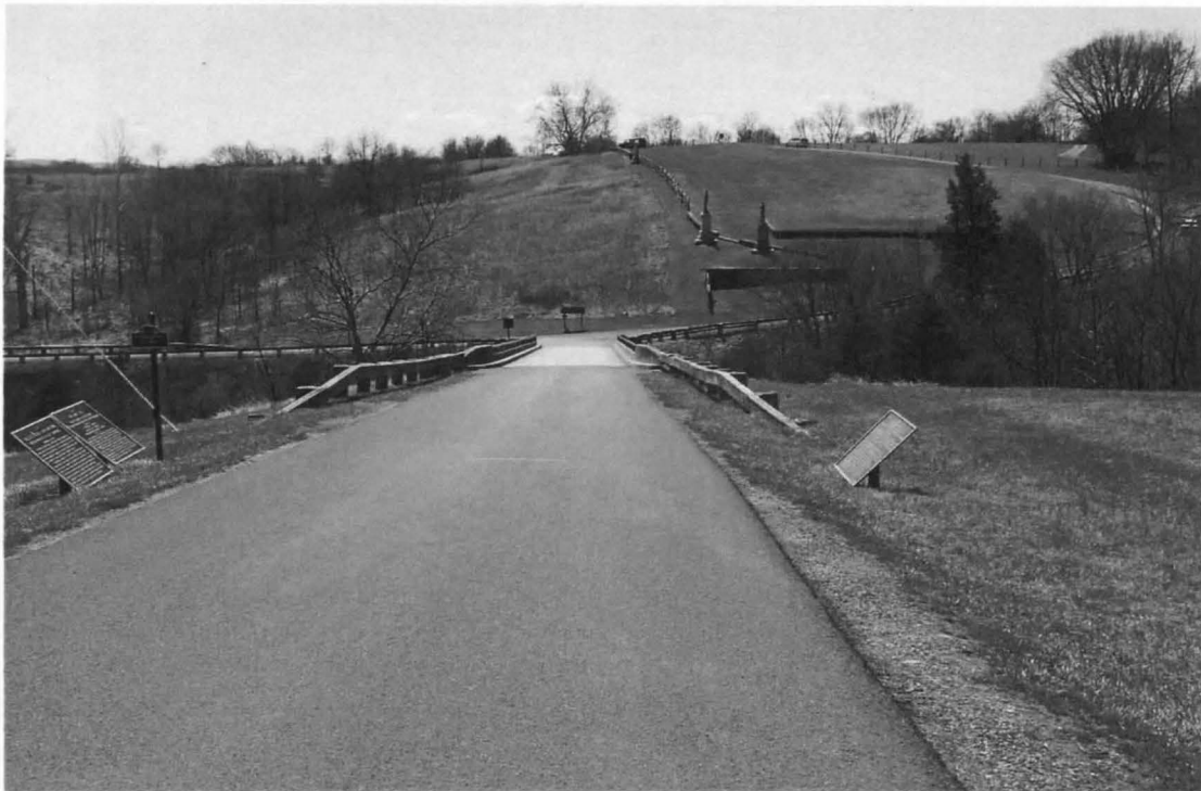
Photo 21 of 28. Rodman Avenue Bridge, Branch Avenue in Distance, Looking South (3/29/2017)
