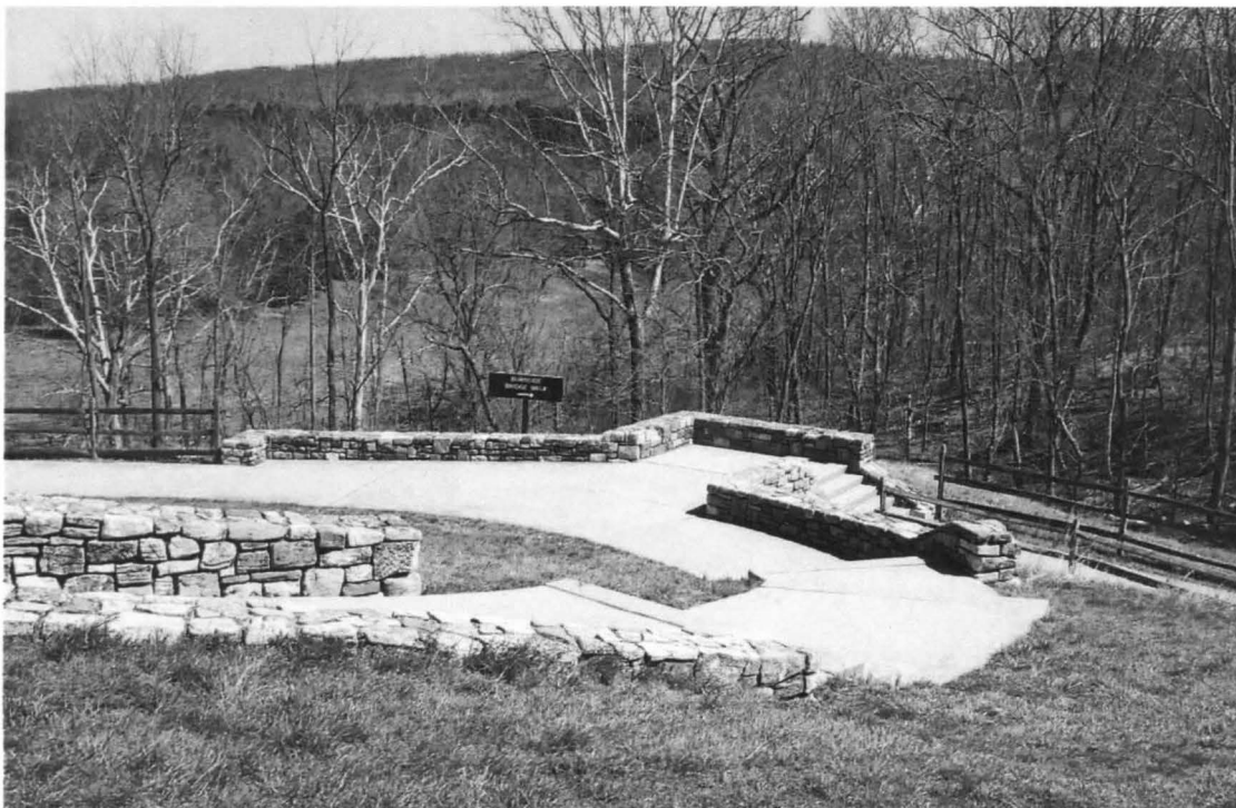
Photo 24 of 28. Burnside Bridge Overlook, Looking Northeast (3/29/2017)
