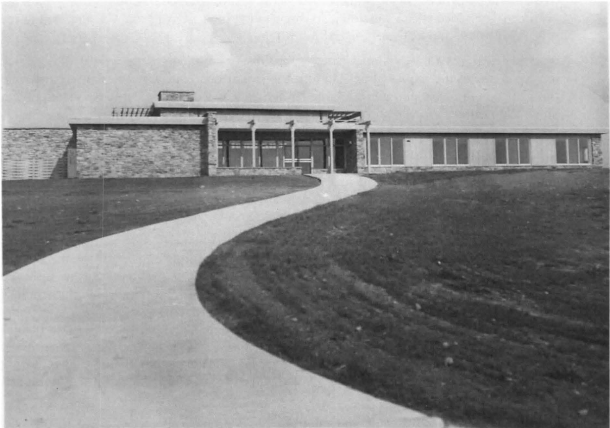
Figure 9. Completed Visitor Center in 1962. Source: Superintendent's Monthly Report, 9 November 1962. Source: Record Group 79, Entry 11, Box 122, National Archives, College Park, Maryland.
