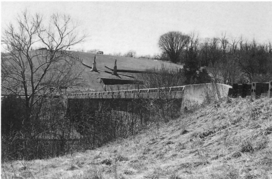
Photo 22 of 28. Rodman Avenue Bridge, Looking Southwest (3/29/2017)
