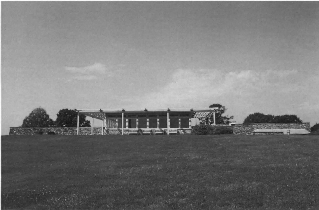
Photo 6 of 28. Visitor Center, East Elevation (Observation Room), Looking Southwest (8/4/2017)
