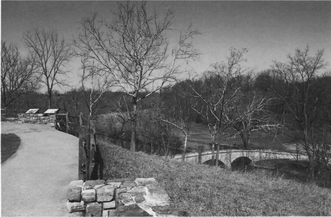
Photo 25 of 28. Burnside Bridge Overlook, Looking Northeast (3/29/2017)
