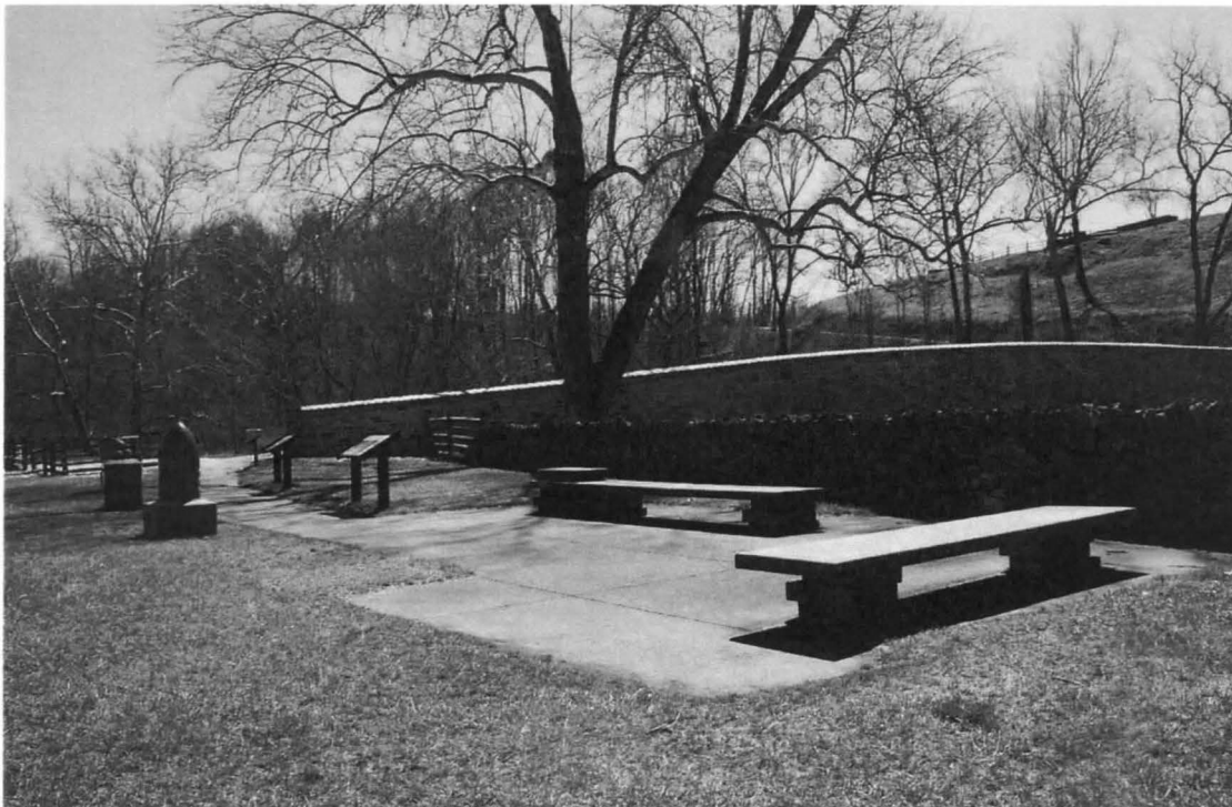
Photo 28 of 28. Burnside Bridge, Lower Terrace and Stone Wall, Looking Southeast (3/29/2017)
