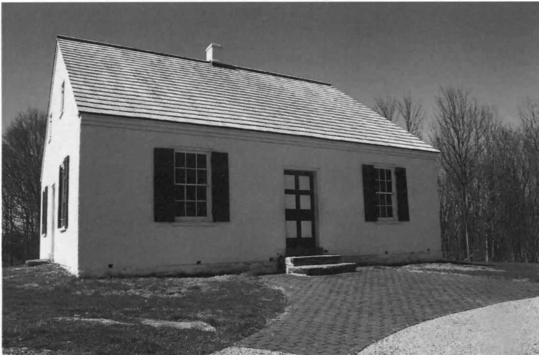
Photo 10 of 28. Dunker Church, East Elevation, Looking Northwest (8/4/2017)
