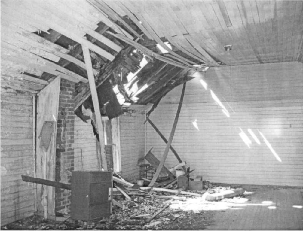
Second floor interior, facing southwest.
