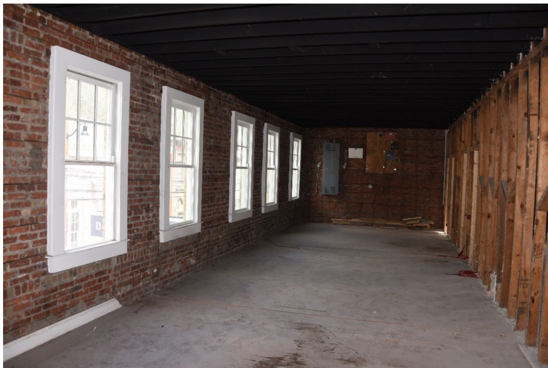
Photo 6 of 15: Second story northern half, view east. 4/15/2021
