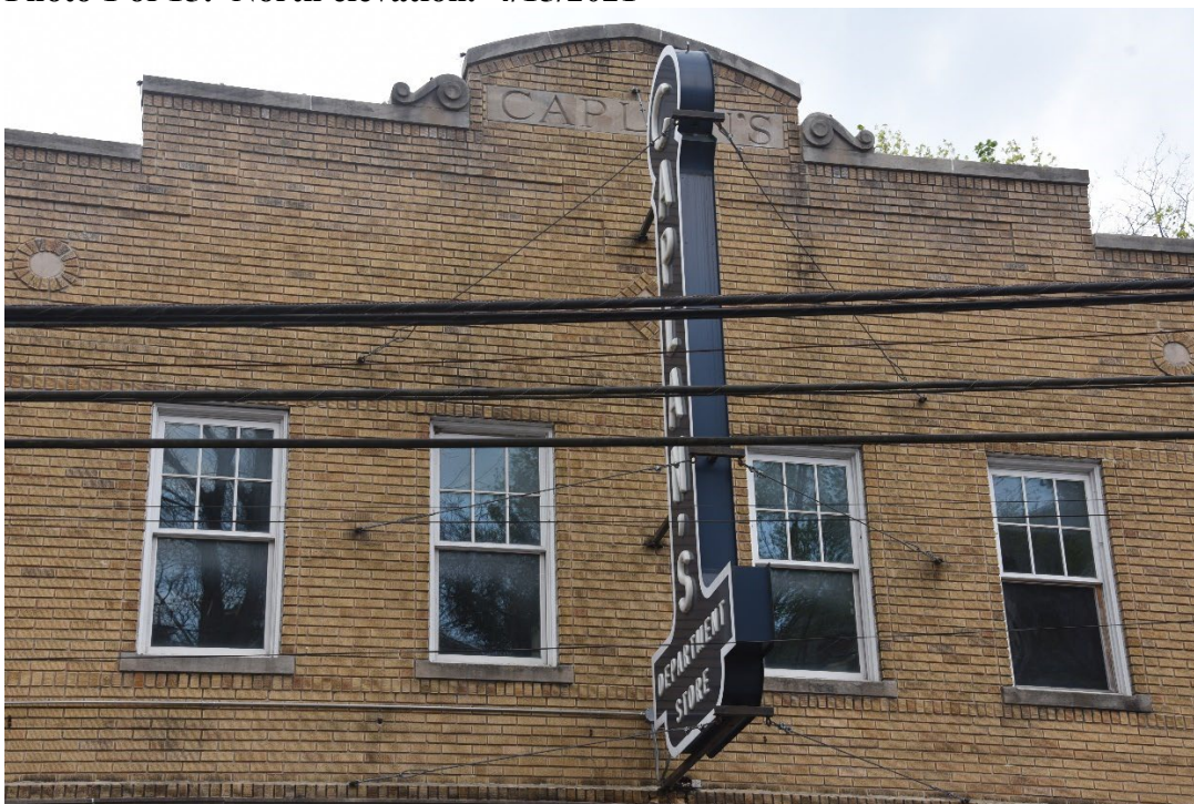
Photo 2 of 15: North elevation, pediment detail. 4/15/2021
