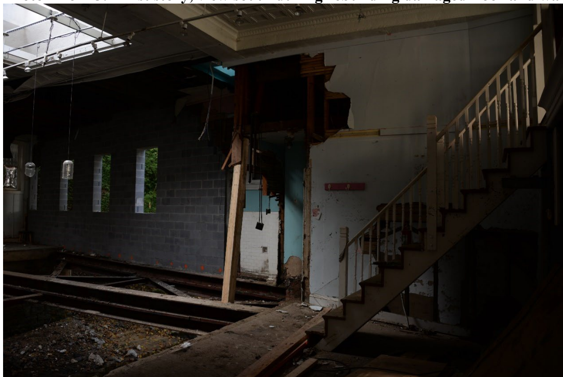
Photo 13 of 15: First story, view west during rebuilding damaged floor and wall. 10/20/2016
