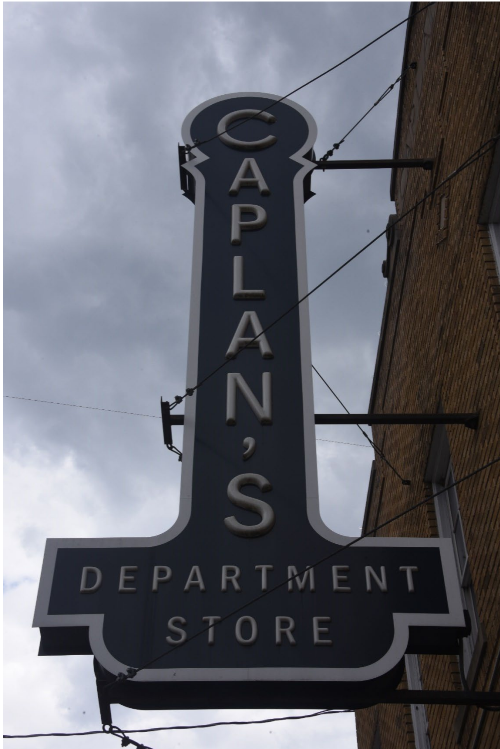
Photo 3 of 15: North elevation, store sign. 4/15/2021
