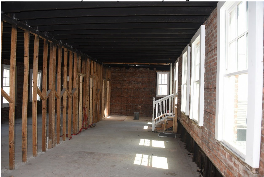
Photo 5 of 15: Second story southern half, view east. 4/15/2021
