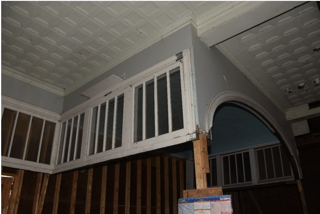
Photo 4 of 15: First story center bay/entrance bay ceiling & transoms. 4/15/2021
