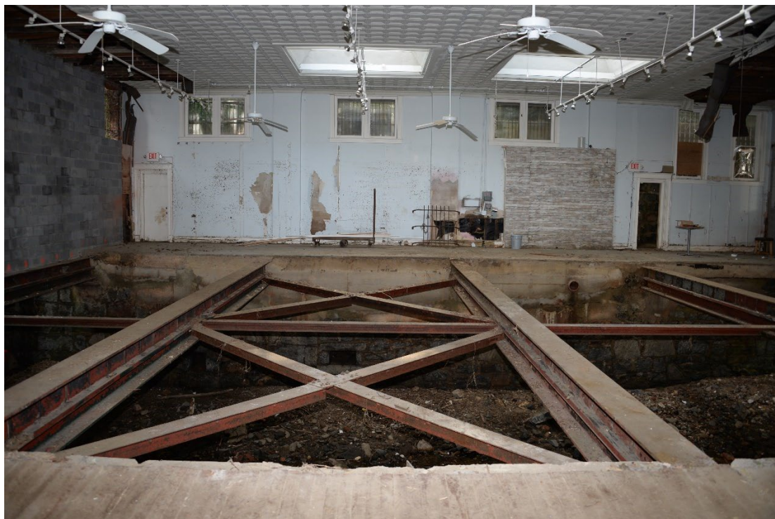
Photo 12 of 15: First story, view south during rebuilding damaged floor and wall. 10/20/2016
