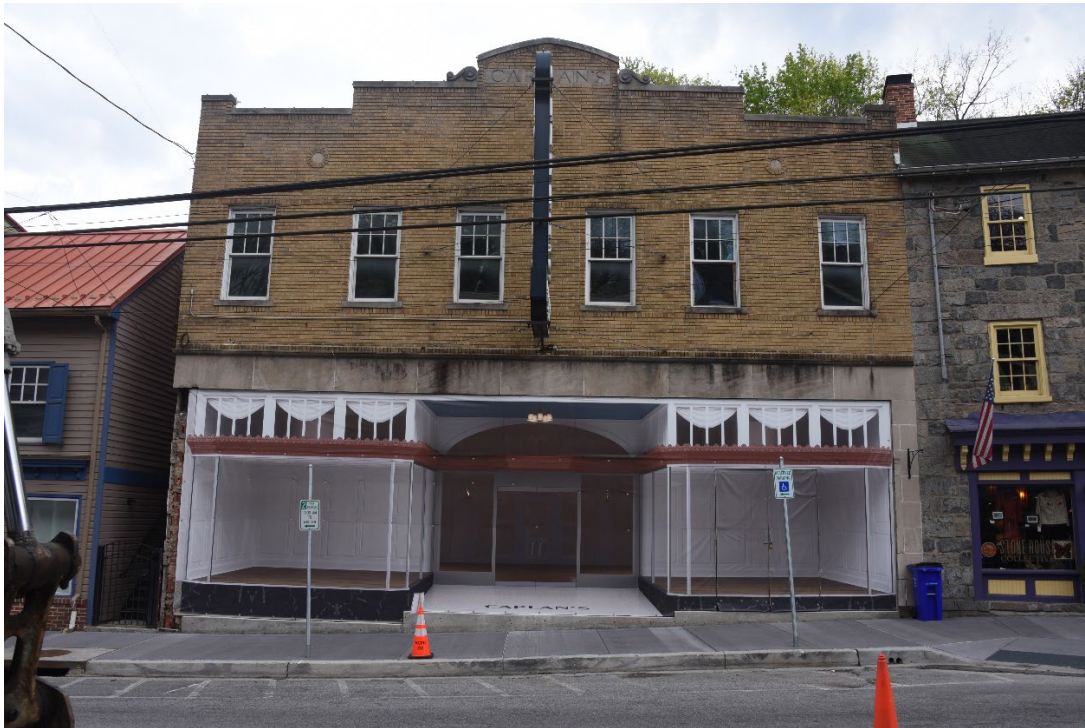
Photo 1 of 15: North elevation. 4/15/2021
