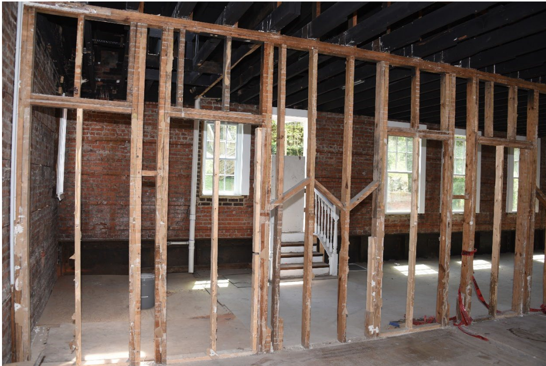
Photo 8 of 15: Second story partition wall at east end, view south. 4/15/2021
