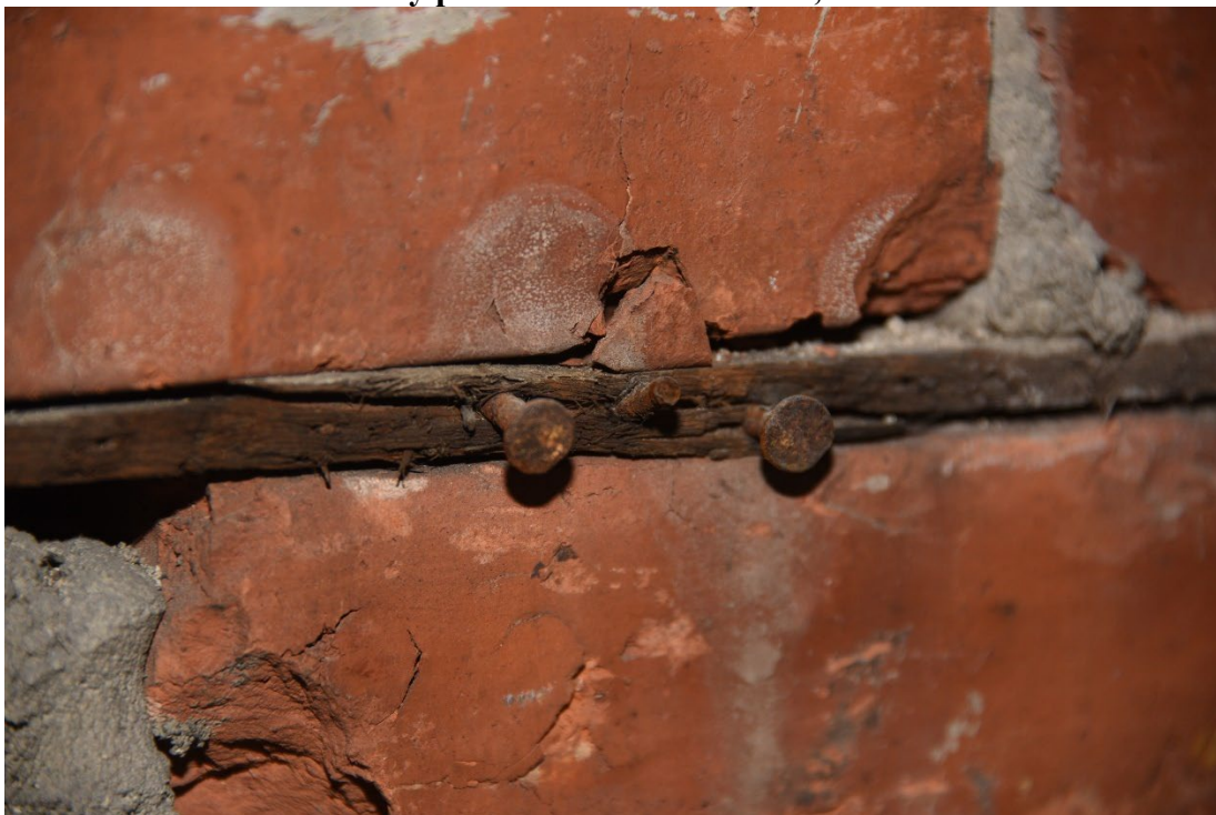
Photo 9 of 15: Wood nailing strip in mortar joint, with lath nails. 4/15/2021
