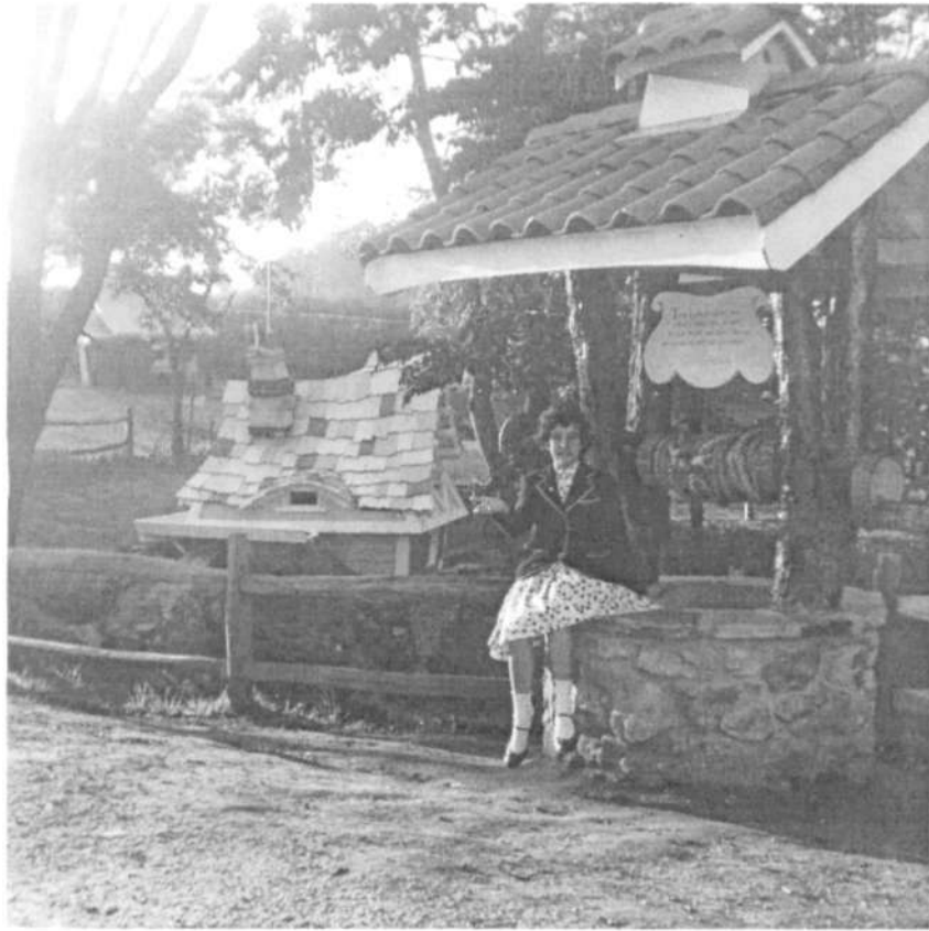
HO-767, Enchanted Forest, Howard County, Maryland. Photographer unknown, January 1956. Wishing Well and Merry Miller's House in the background. Digital image courtesy of the Howard County Historical Society.
