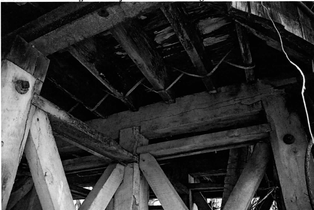
Photo 6 of 11: Framing underneath with joists and cross-bracing.
