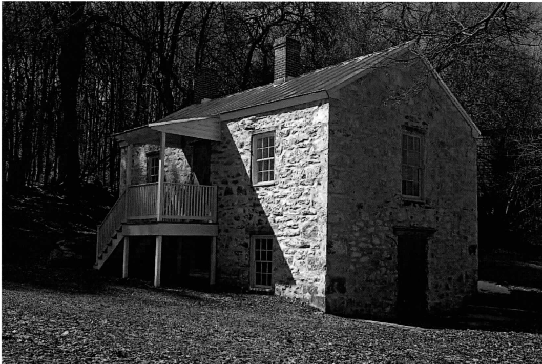
Photo 10 of 11: House, south and east elevations.
