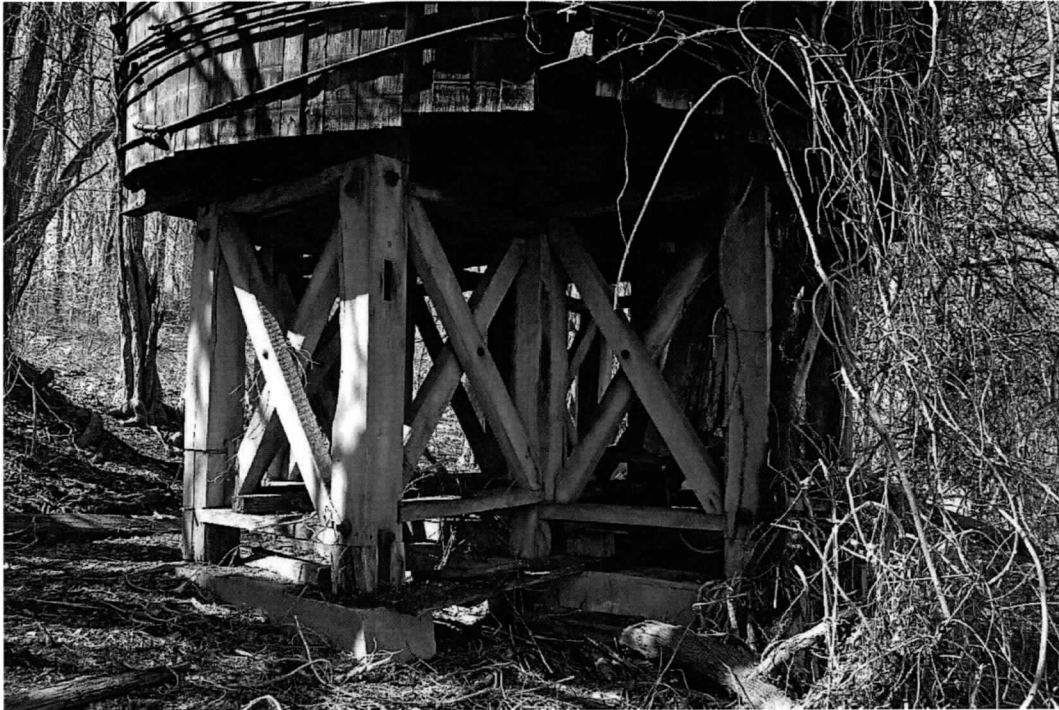
Photo 3 of 11: Base of tower from southeast.
