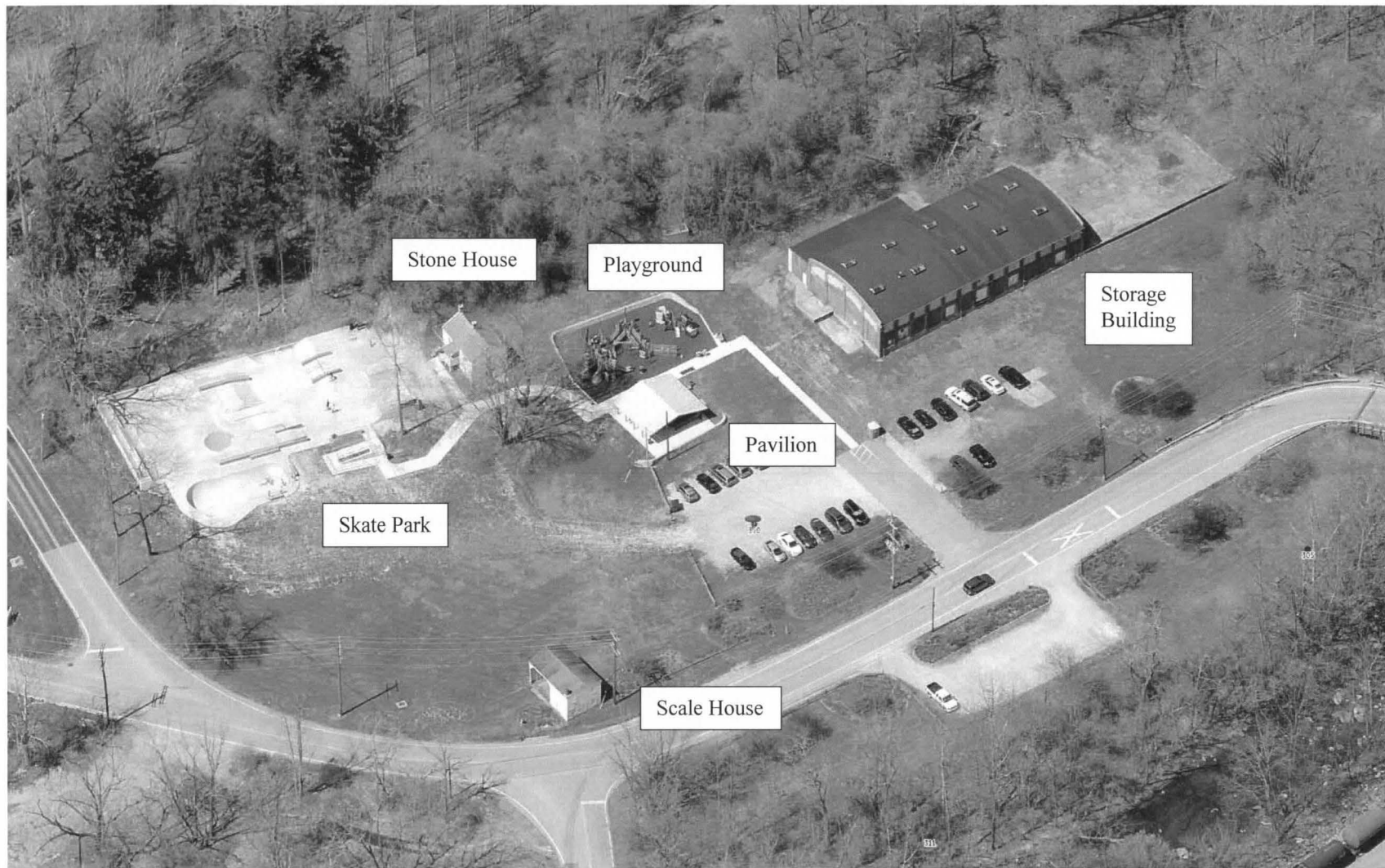
HO-751 Howard Cotton Factory/B. F. Shriver Cannery 350 Route 32 Pictometry bird's-eye view of site looking west, 2017.
