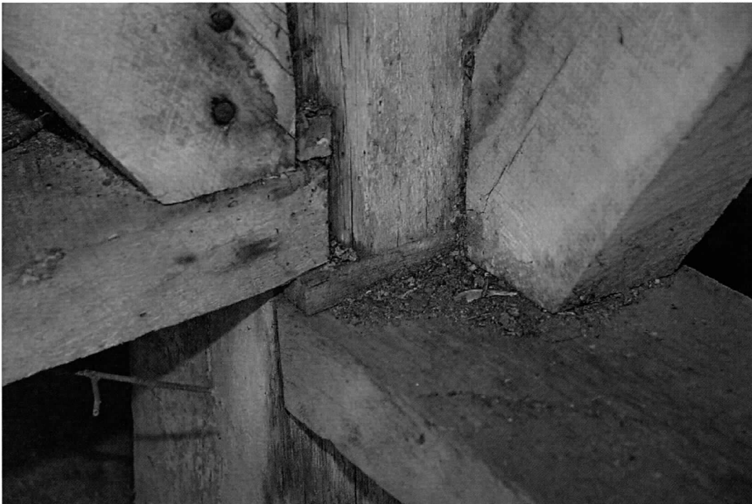
Photo 5 of 11: Post/girt/brace joint detail with wedges.
