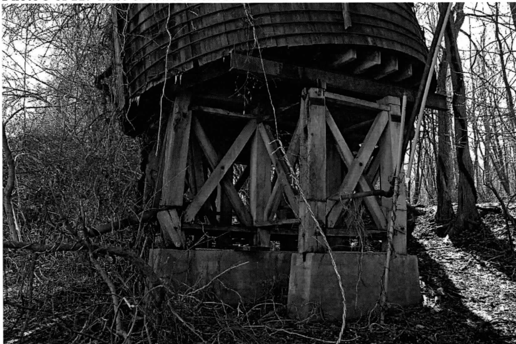
Photo 4 of 11: Base of tower from northeast.
