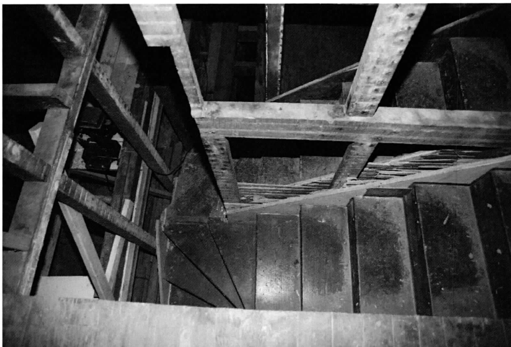
Photo 9 of 15: House, interior, view of back-to-back stairs looking down from attic. 1/2/2020
