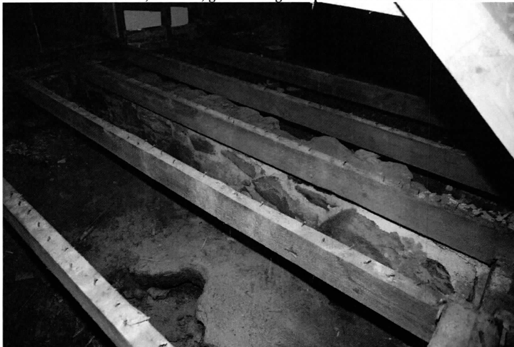
Photo 14 of 15: House, interior, retaining wall under west addition, view northwest. 3/6/2020
