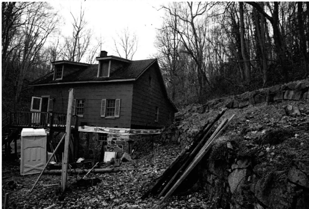
Photo 2 of 15: House, east & north elevations, with retaining walls. 1/2/2020
