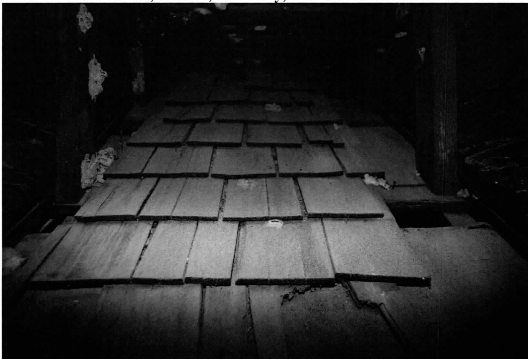
Photo 12 of 15: House, interior, attic story, shingles on east captured under dormer. 1/2/2020
