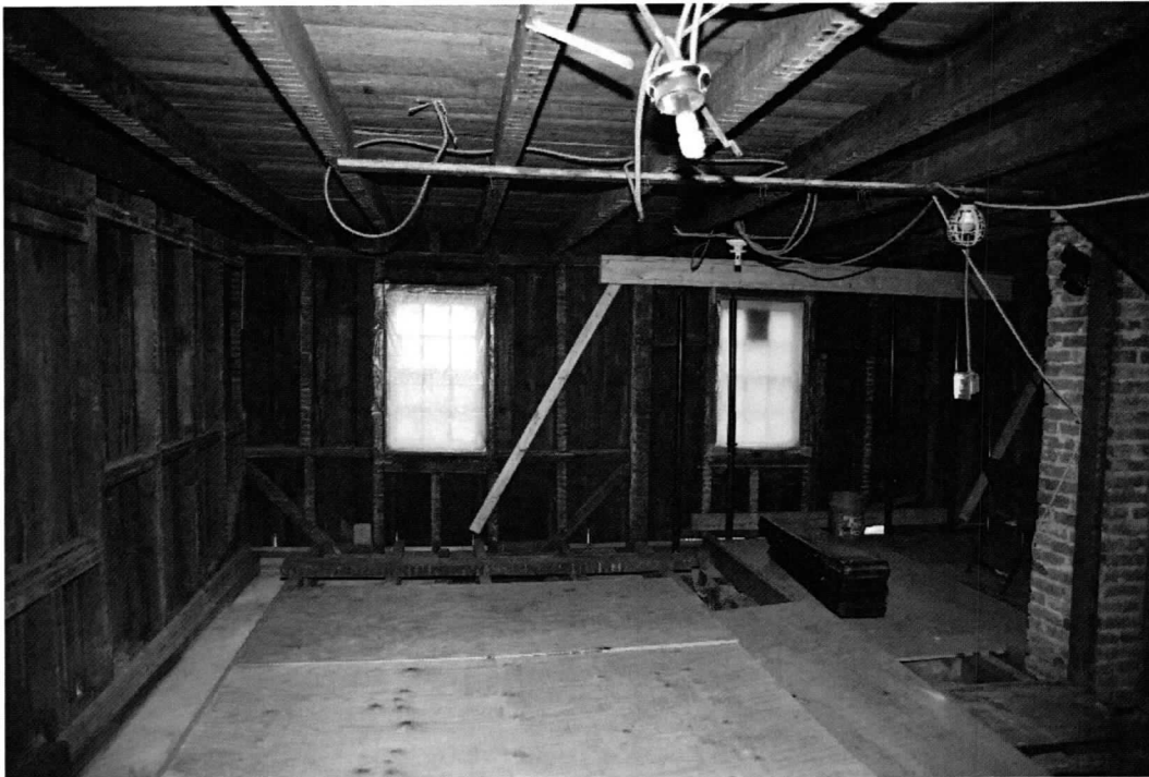
Photo 7 of 15: House, interior, first story, east elevation of north addition. 1/2/2020
