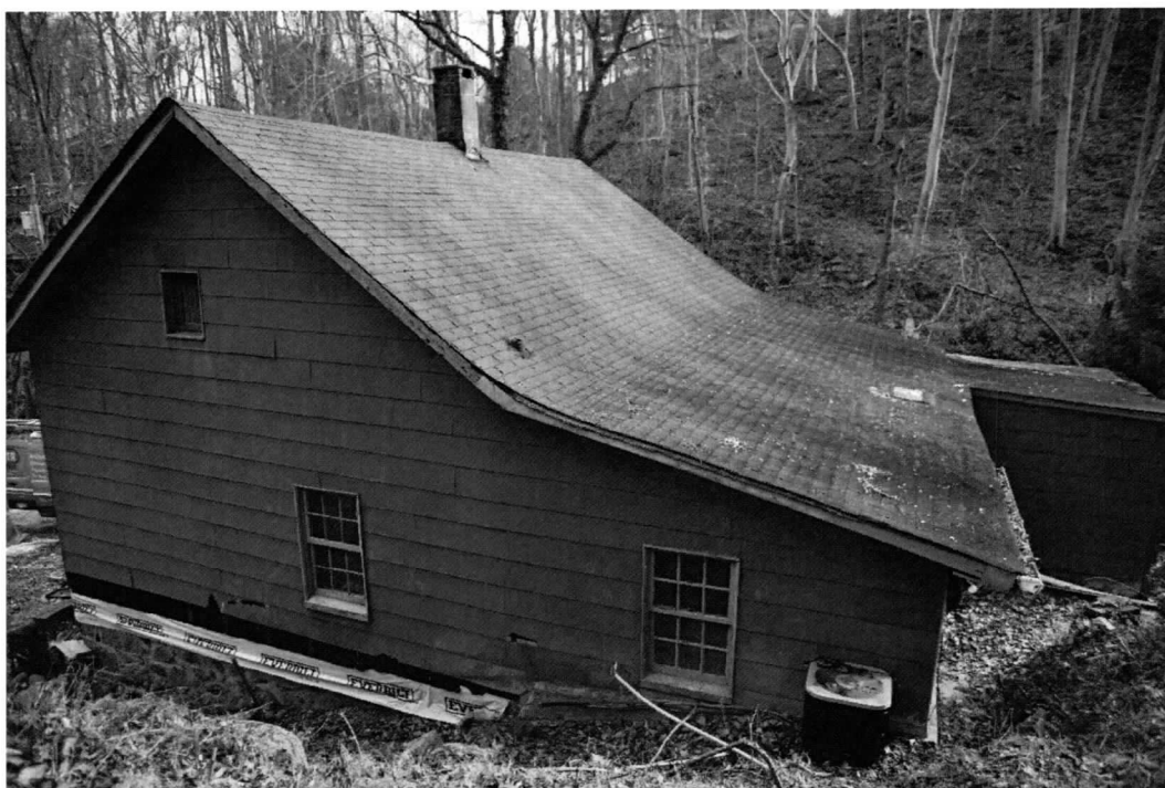
Photo 3 of 15: House, north elevation from northwest. 1/2/2020
