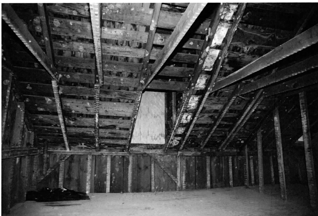
Photo 11 of 15: House, interior, attic story, view east of north addition. 1/2/2020
