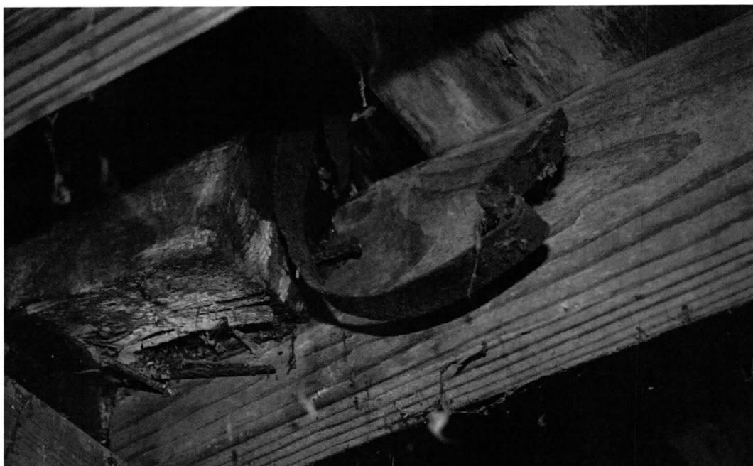
Photo 13 of 15: House, interior, gutter hanger captured in later addition. 1/30/2020
