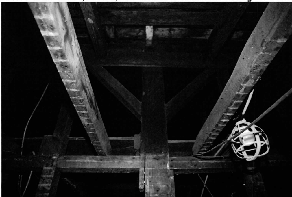
Photo 10 of 15: House, interior, view of original braced frame with inserted studs, ledger boards and joists. West wall, view from east side. 1/2/2020
