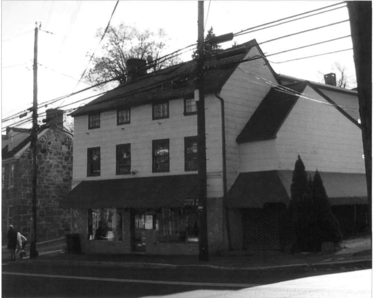
HO-573 The Judge's Bench (Buzz Suter Building) 8385 Main Street (MD 144), Ellicott City Photo by Jennifer K. Cosham, 11/28/2012 North elevation
