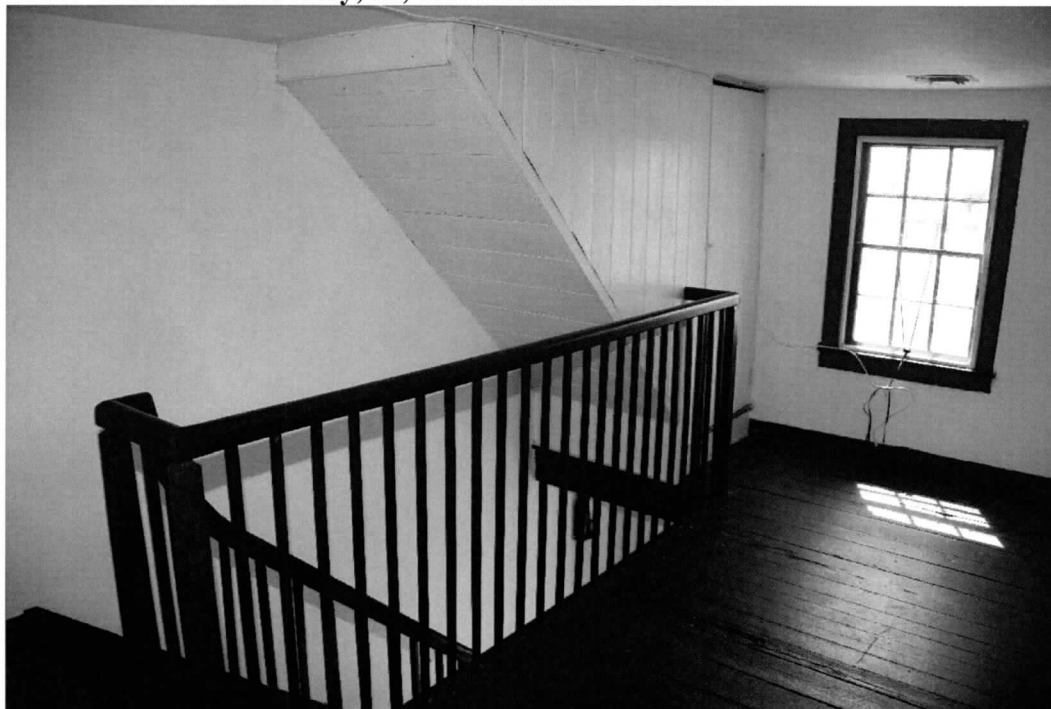
Photo 13 of 16: Second-story passage, view southeast. 4/10/2017
