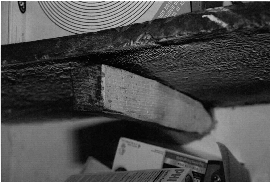
Photo 6 of 16: First-story closet shelf support under stairs. 4/10/2017
