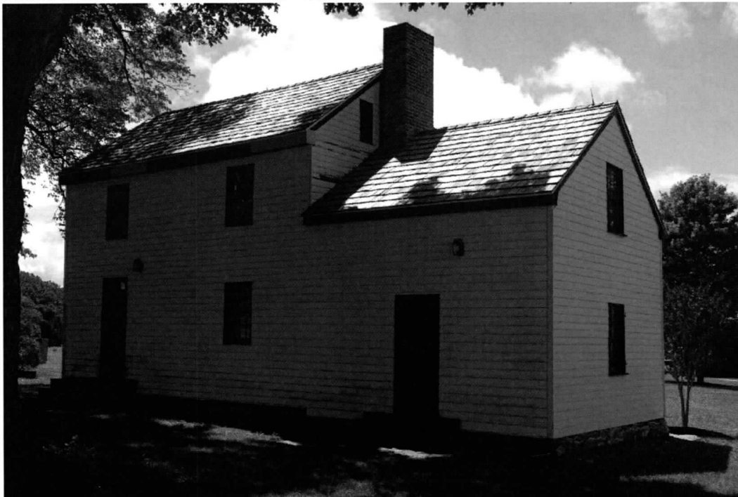
Photo 2 of 22: North & west elevations. 7/7/2017
