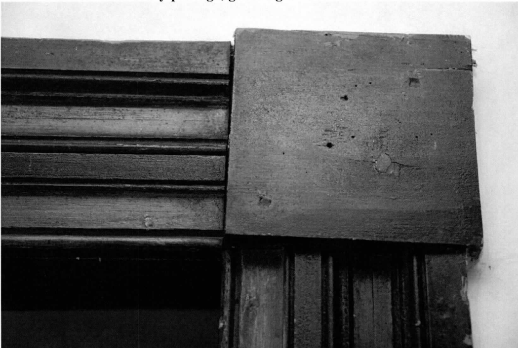
Photo 5 of 16: First-story passage, front door architrave with decorative paint. 4/10/2017
