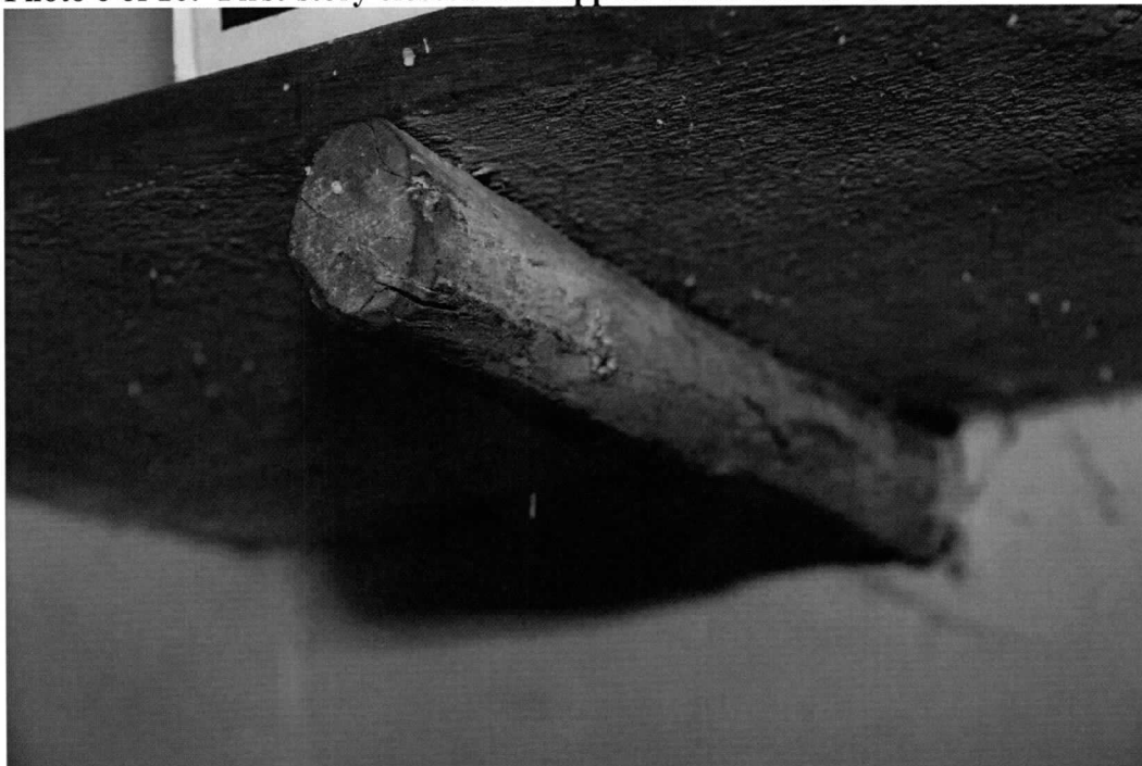
Photo 7 of 16: First-story closet shelf support under stairs. 4/10/2017
