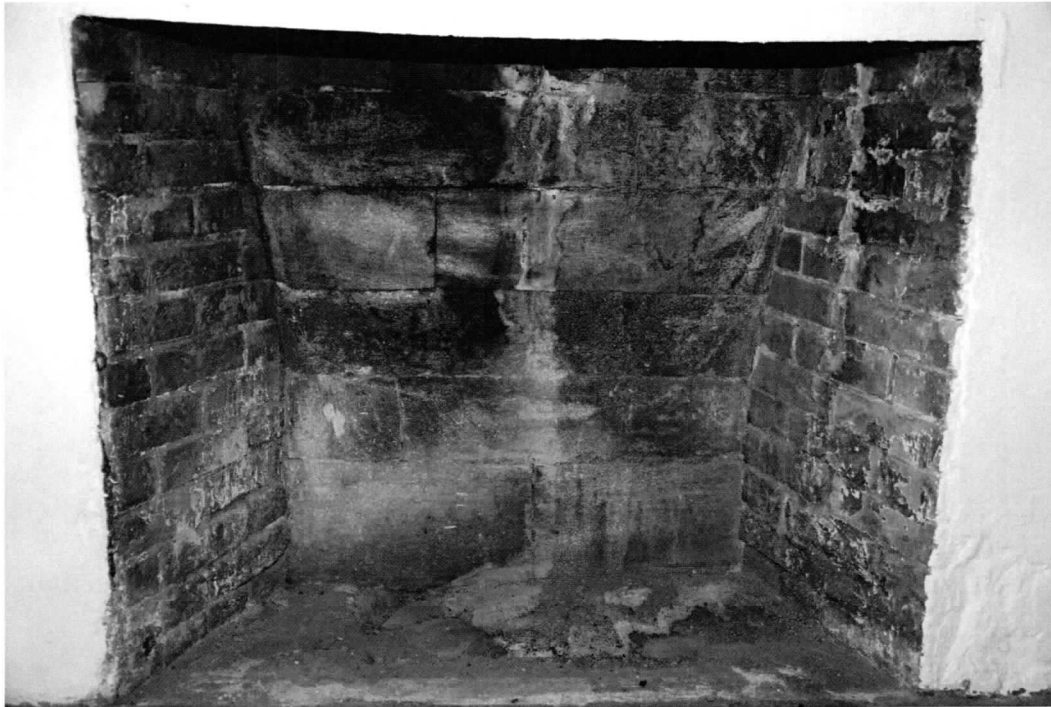
Photo 10 of 16: First story, main block room, firebox detail. 4/10/2017
