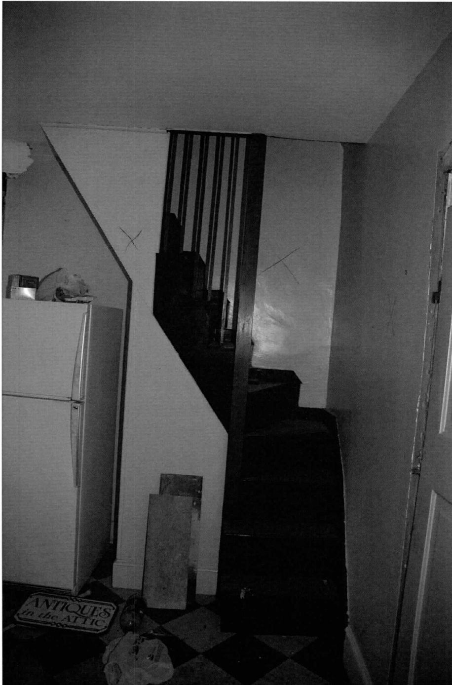
Photo 16 of 24: Northwest room stairway, view west.
