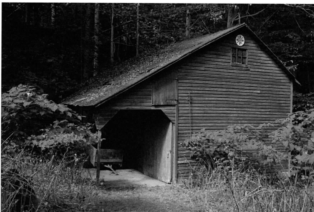
Photo 23 of 24: Stable, south & east elevations.
