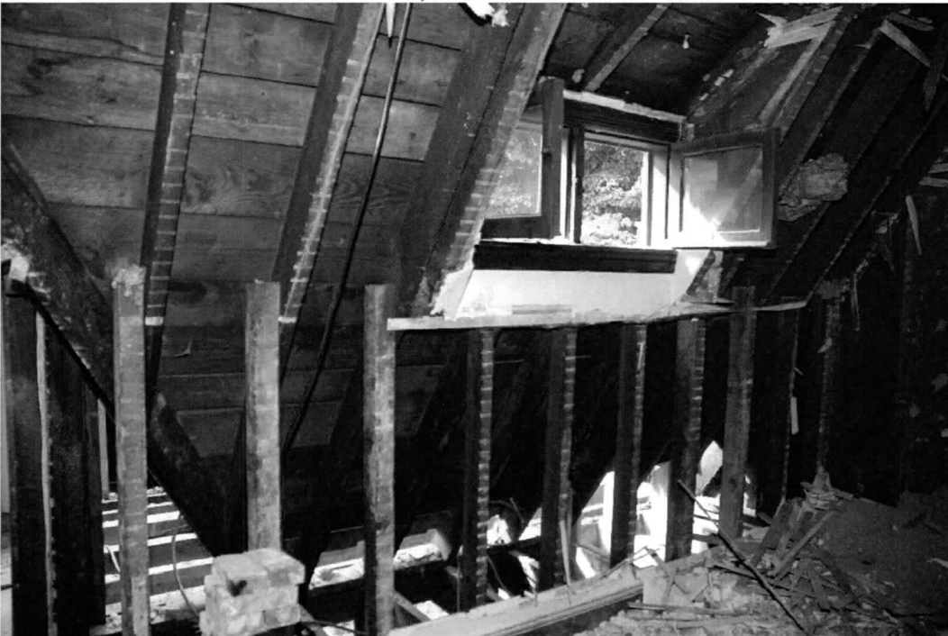
Photo 19 of 24: Attic, west wall.
