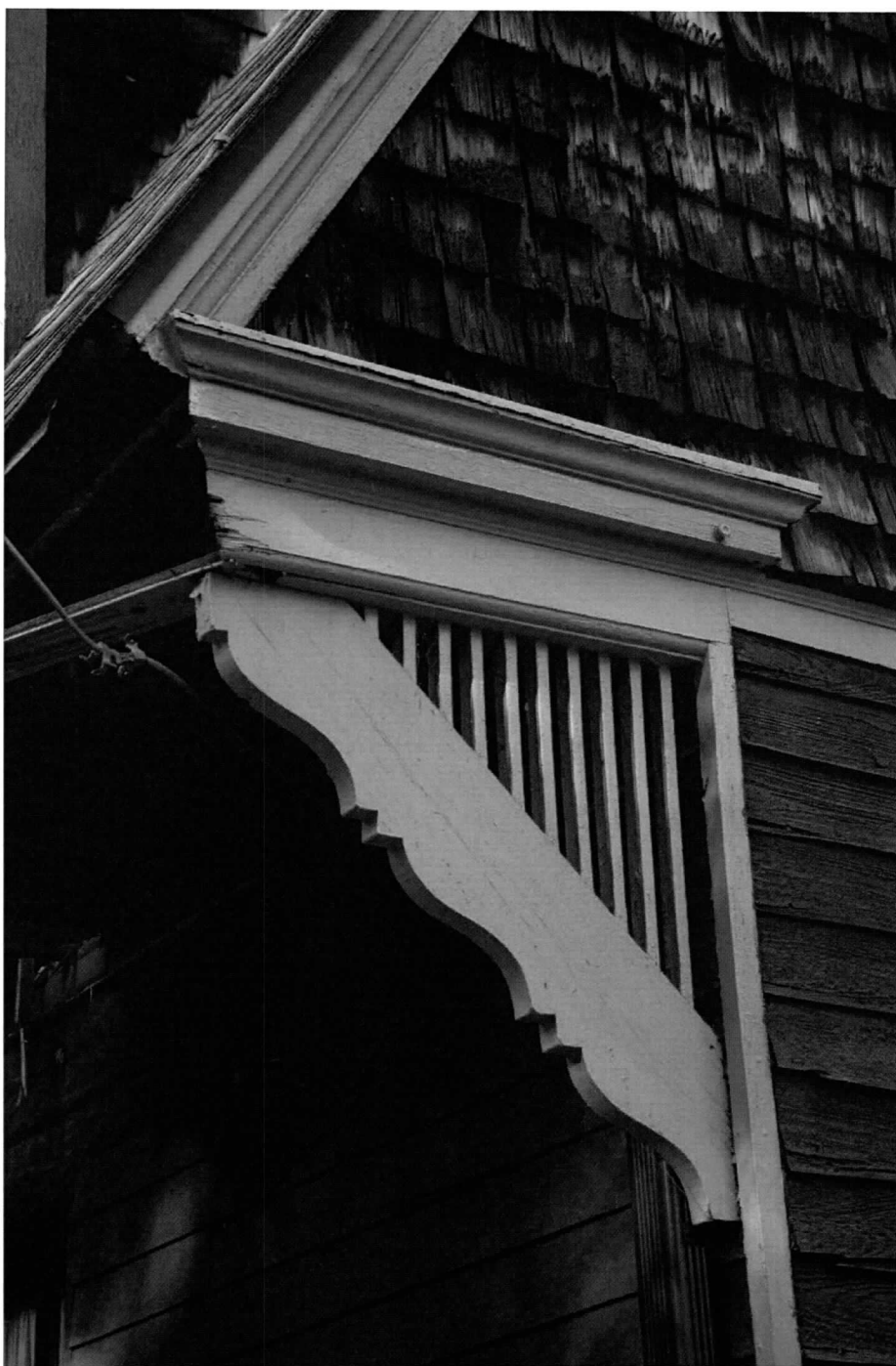
Photo 5 of 24: Southwest corner roof bracket.
