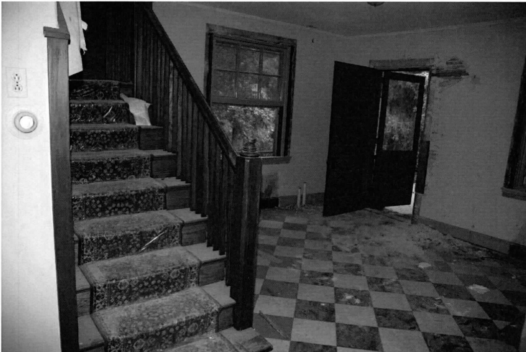
Photo 10 of 24: Northeast room, view northeast.
