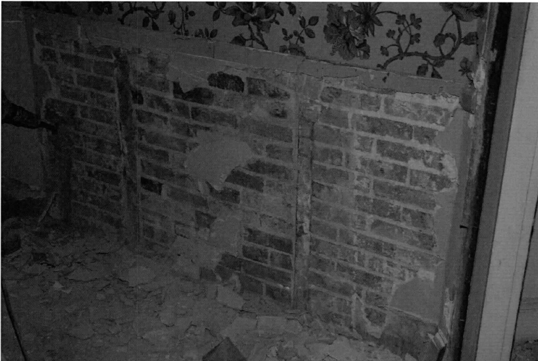
Photo 14 of 24: Southwest room, fireplace in northwest corner exposed during demolition.
