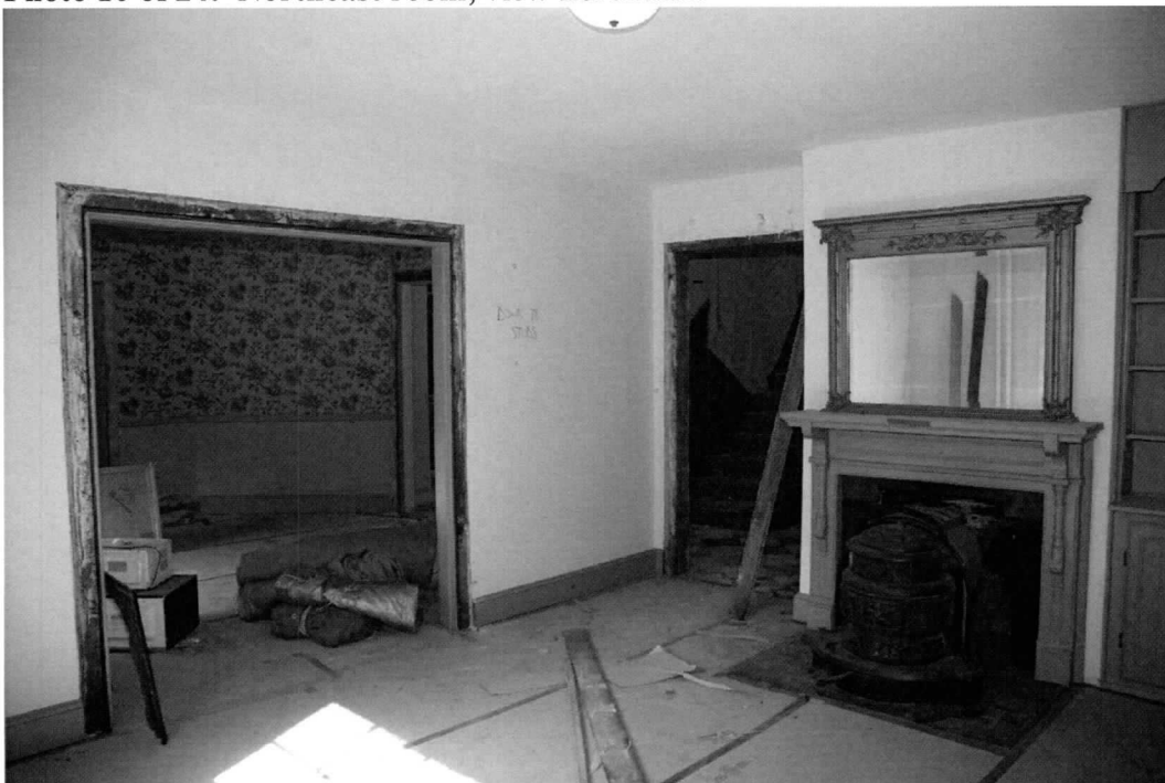
Photo 11 of 24: Southeast room, view northwest.
