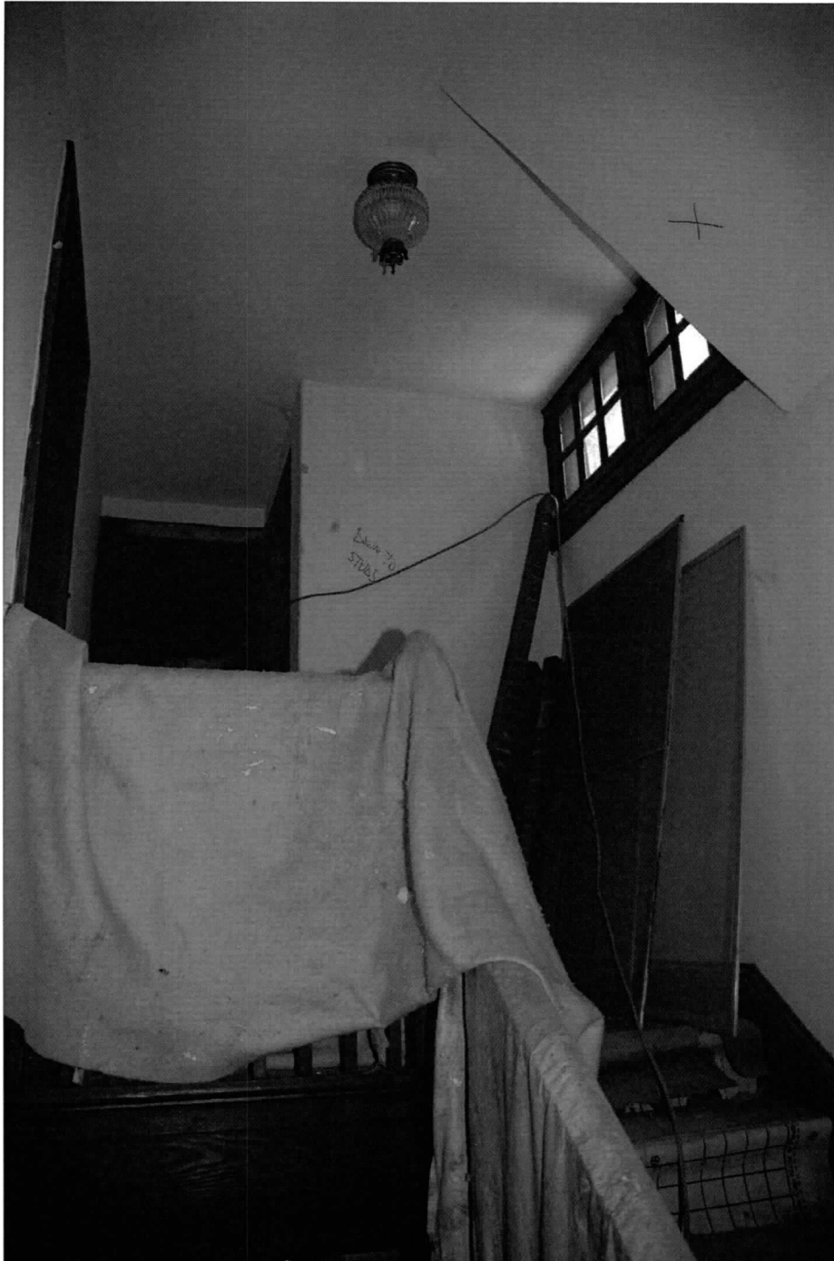
Photo 17 of 24: Stairway to second story.
