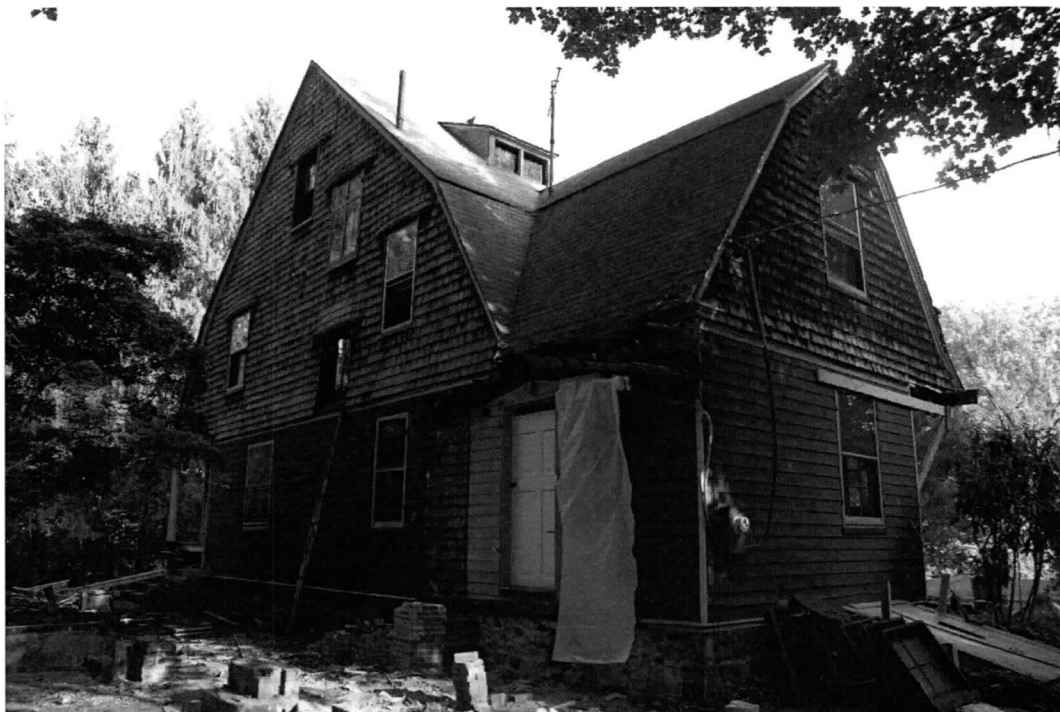
Photo 6 of 24: North & west elevations.
