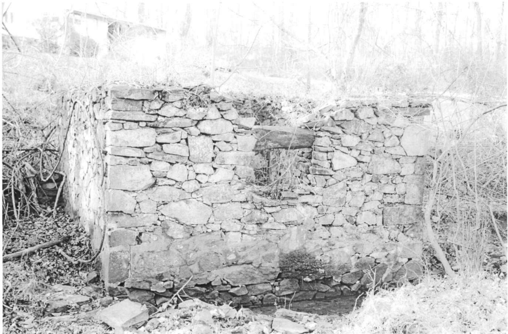
HO-451 Hoogewerff-Donaldson Cottage 6460 Elibank Drive Springhouse, south elevation Ken Short, December 2006 15/15
