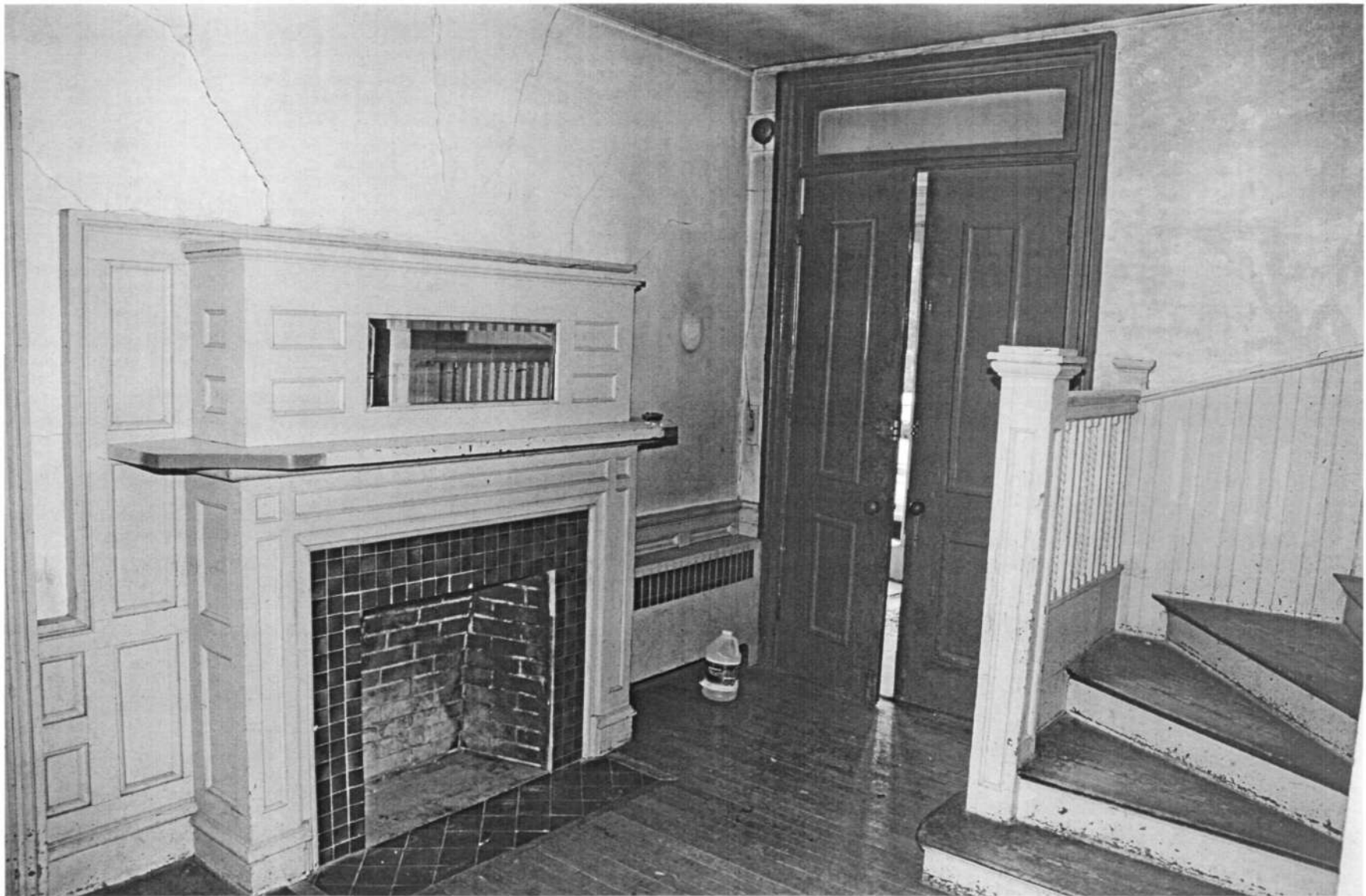
HO-451 Hoogewerff-Donaldson Cottage 6460 Elibank Drive Stair hall, view southwest Ken Short, December 2006 9/15
