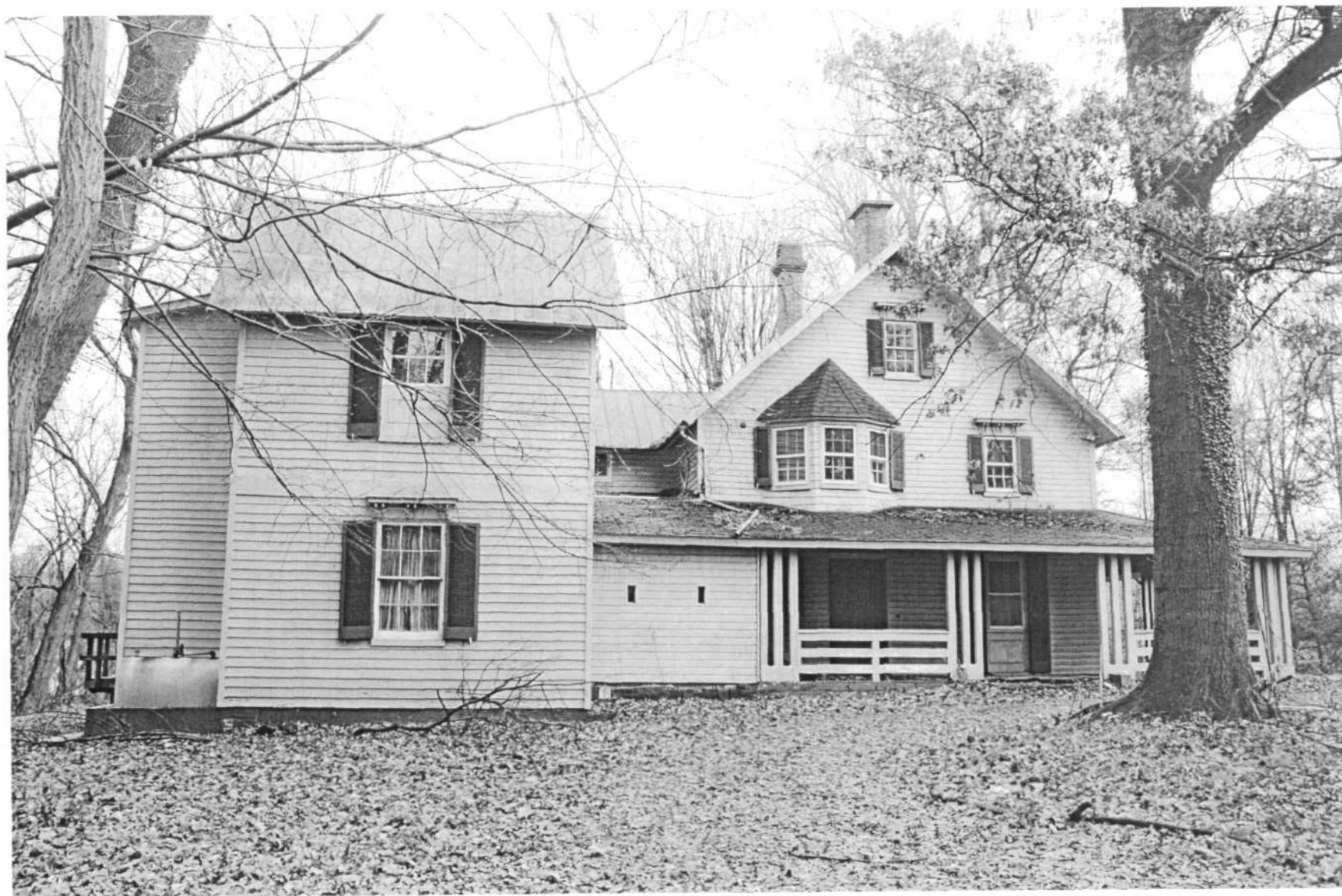
HO-451 Hoogewerff-Donaldson Cottage 6460 Elibank Drive West elevation Ken Short, December 2006 3/15
