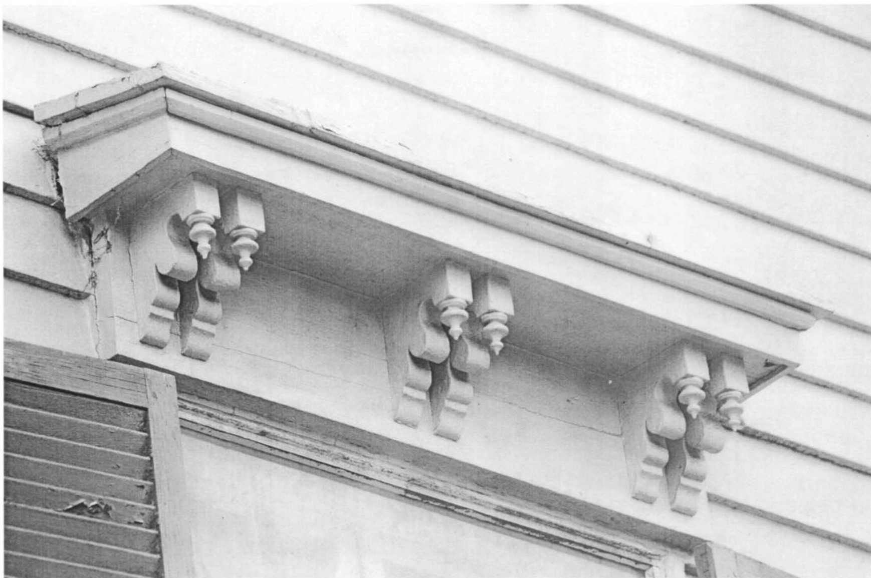
HO-451 Hoogewerff-Donaldson Cottage 6460 Elibank Drive Northwest addition, south elevation window cornice Ken Short, December 2006 7/15
