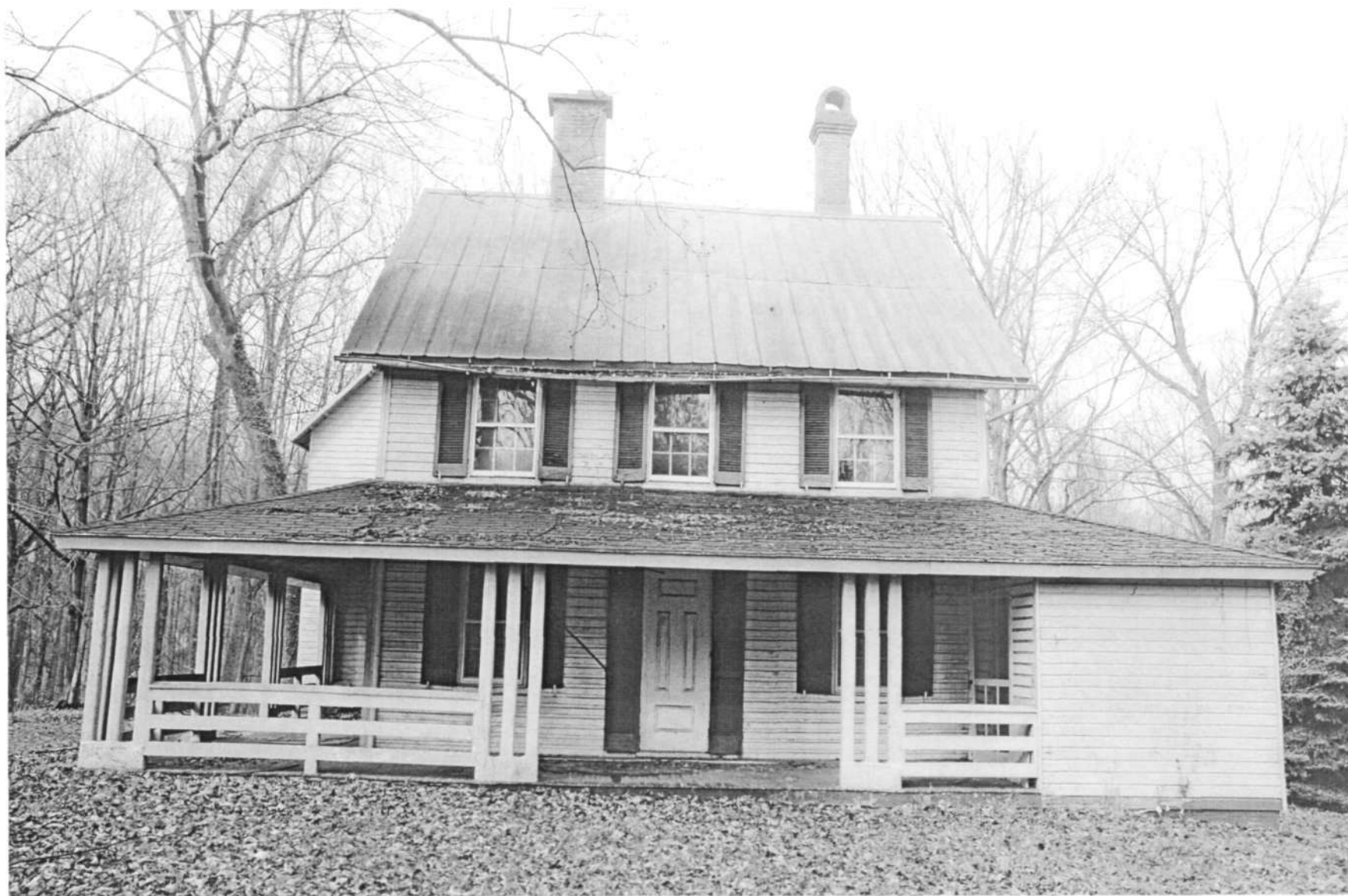
HO-451 Hoogewerff-Donaldson Cottage 6460 Elibank Drive South elevation Ken Short, December 2006 1/15
