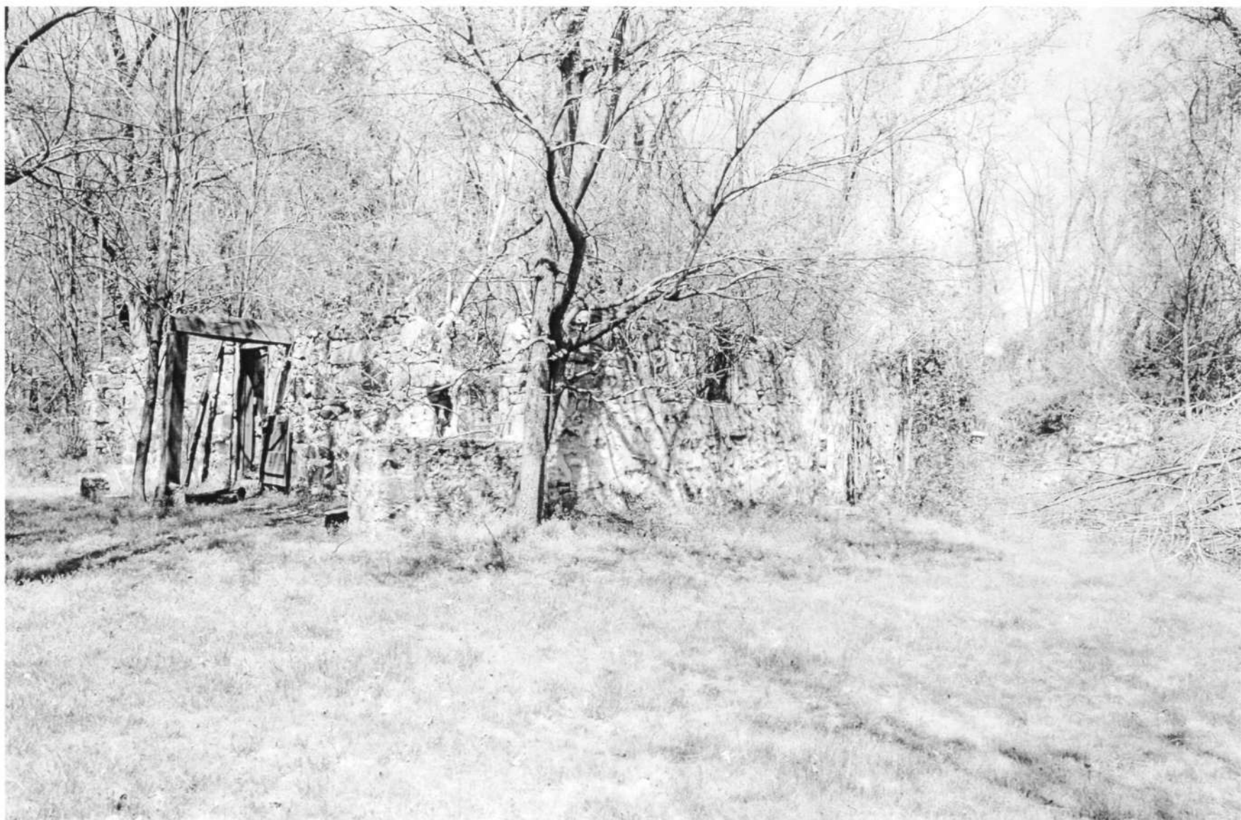
HO-411 Woodlawn Slave Quarter 9254 Old Annapolis Road Barn foundation, view from southwest Ken Short, April 2006 13/14
