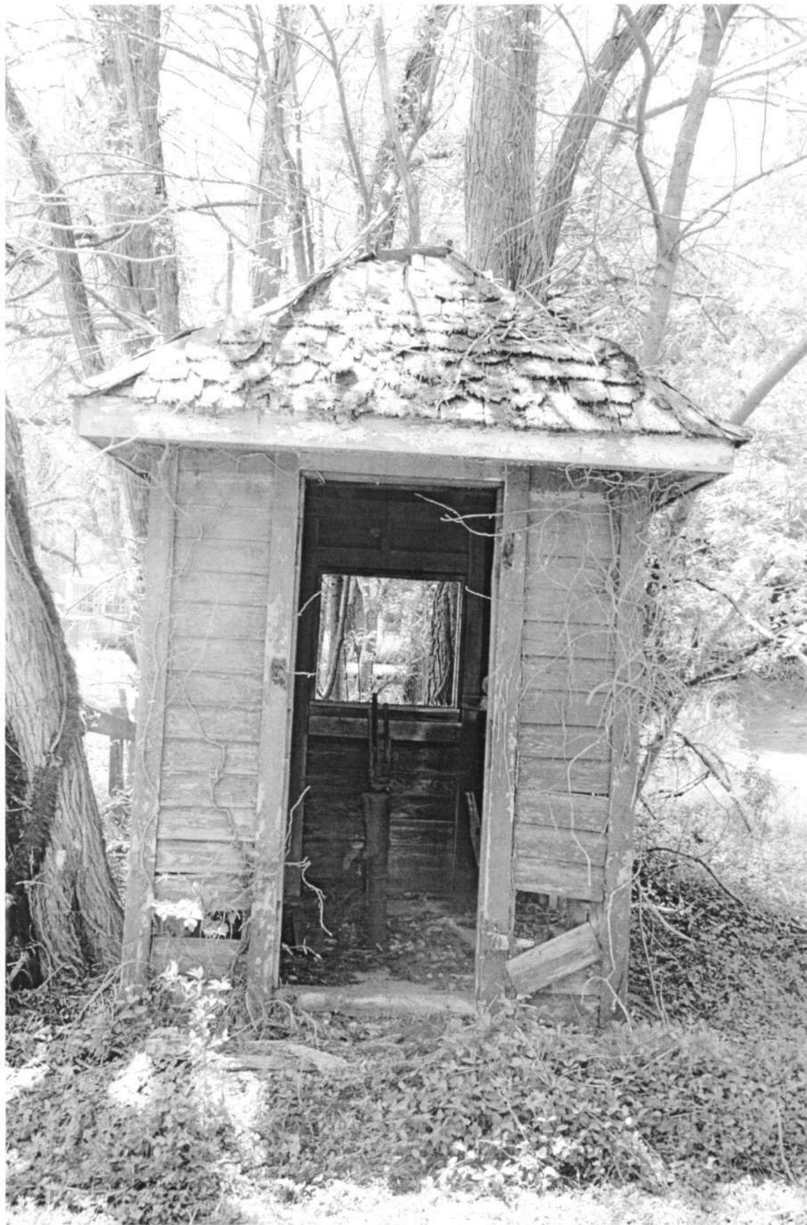
HO-411 Woodlawn Slave Quarter 9254 Old Annapolis Road Well house, east elevation Ken Short, April 2006 14/14
