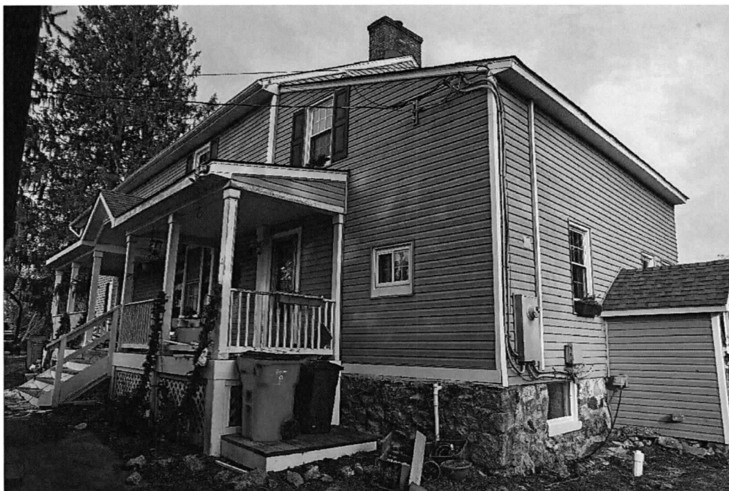
Photo 4 of 20: Northwest and southwest elevations. 1/19/2022
