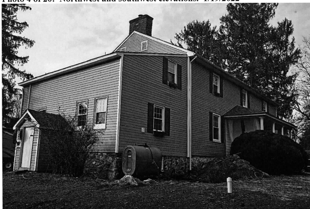
Photo 5 of 20: Southwest & southeast elevations. 1/19/2022
