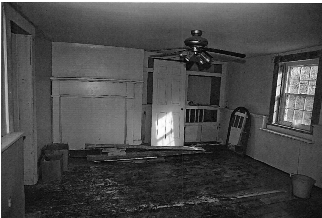
Photo 17 of 20: West chamber, view west. 1/19/2022
