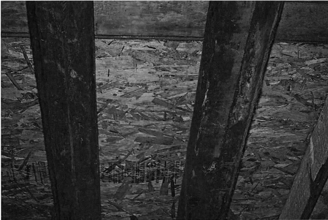
Photo 10 of 20: Northeast room, railroad stringers re-used as second-story joists. 1/19/2022
