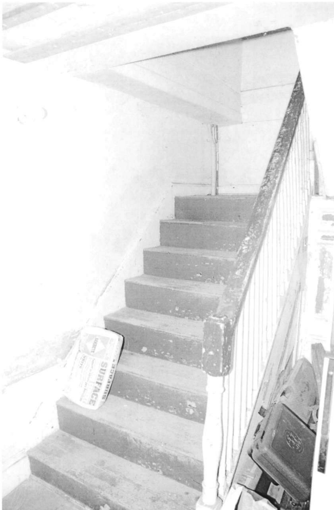
HO-387 "Hockley" 5925 River Road Stair hall, view south Ken Short, October 2006 7/15
