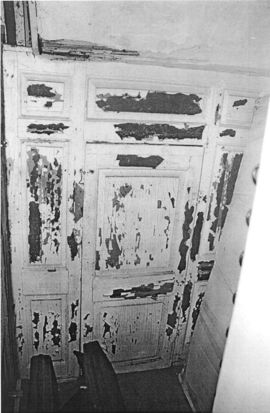
HO-387 "Hockley" 5925 River Road Stair hall, cellar door Ken Short, October 2006 9/15
