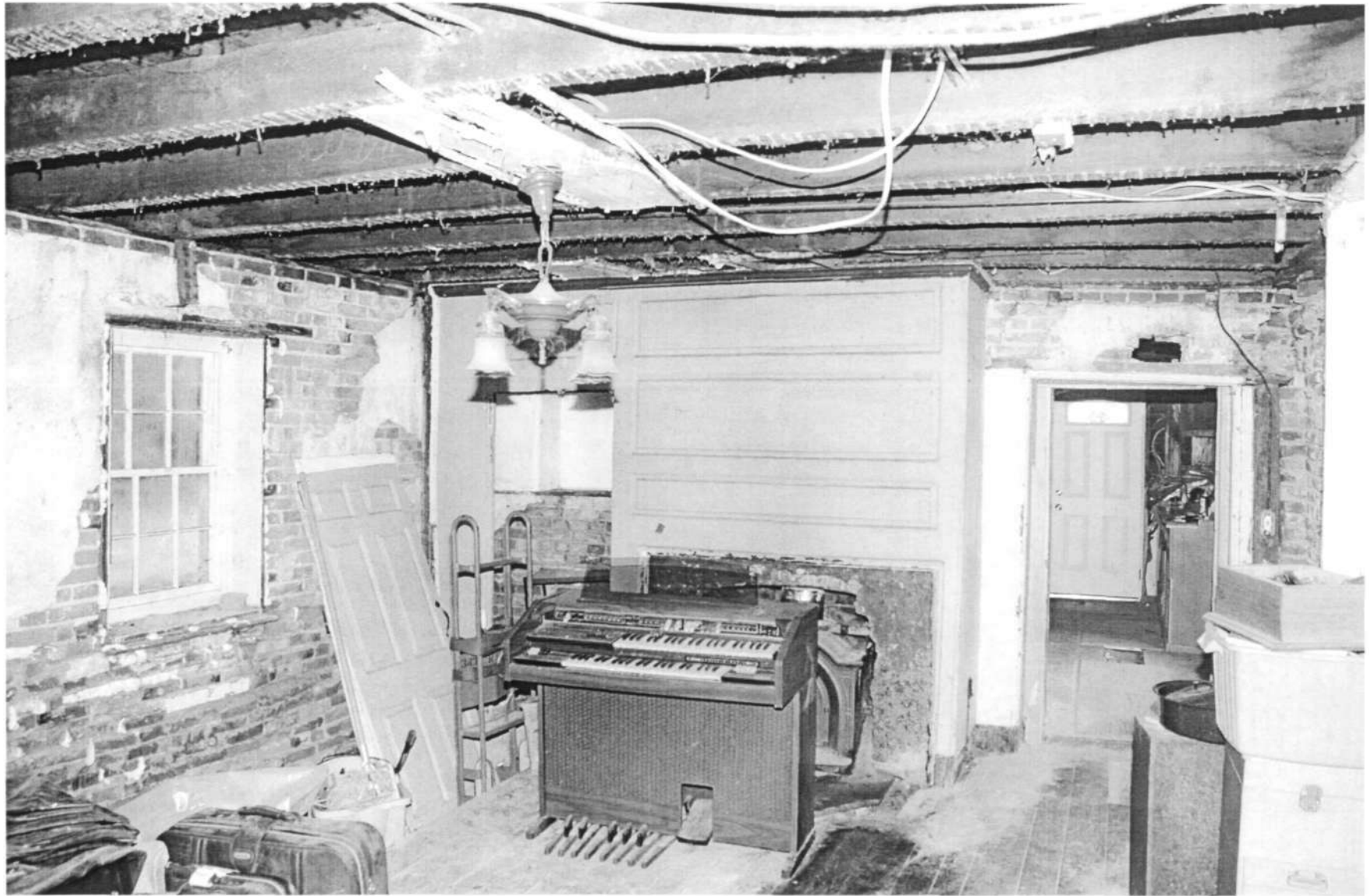
HO-387 "Hockley" 5925 River Road Center room, view west Ken Short, October 2006 10/15
