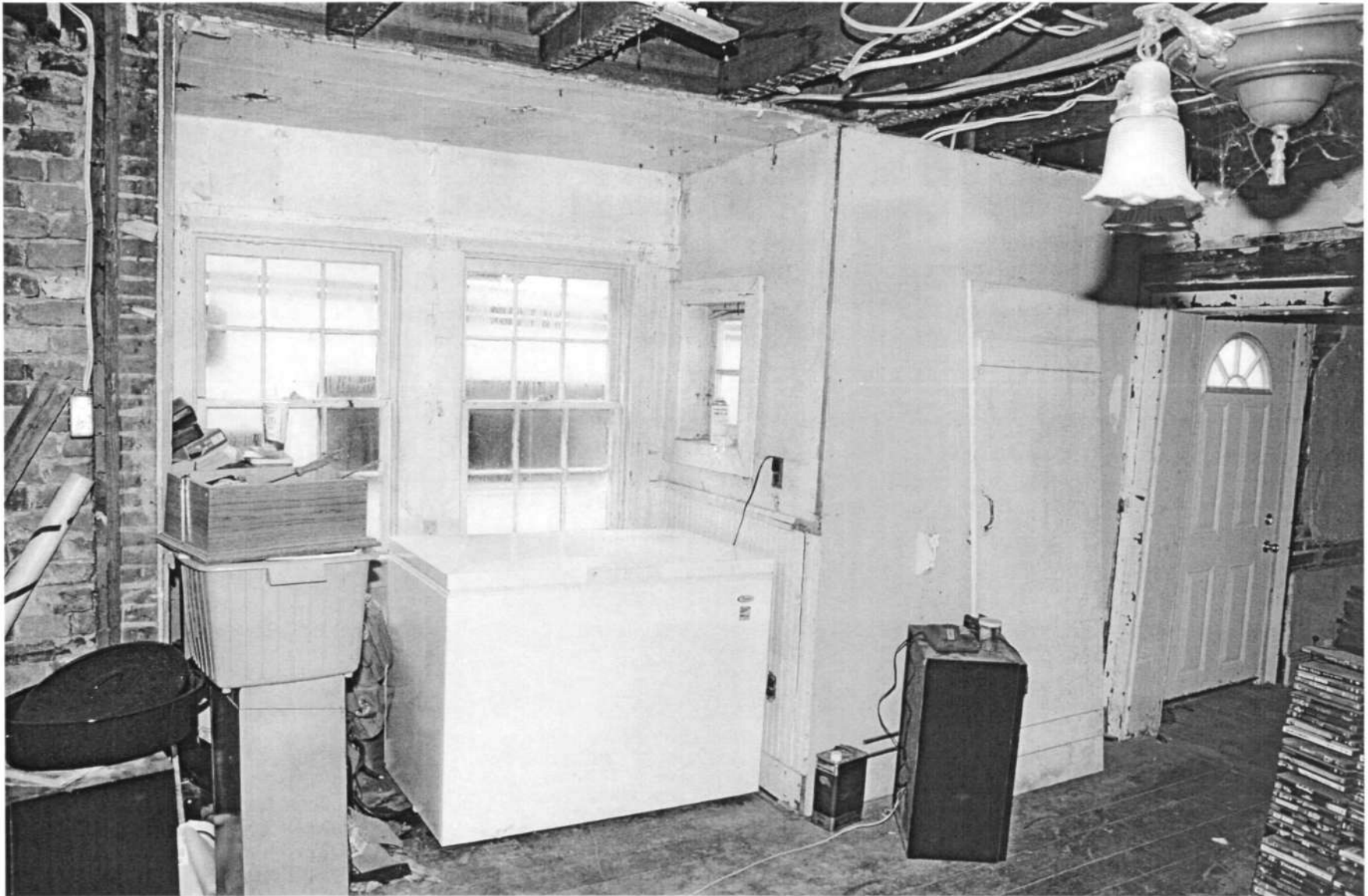
HO-387 "Hockley" 5925 River Road Center room, view south Ken Short, October 2006 12/15
