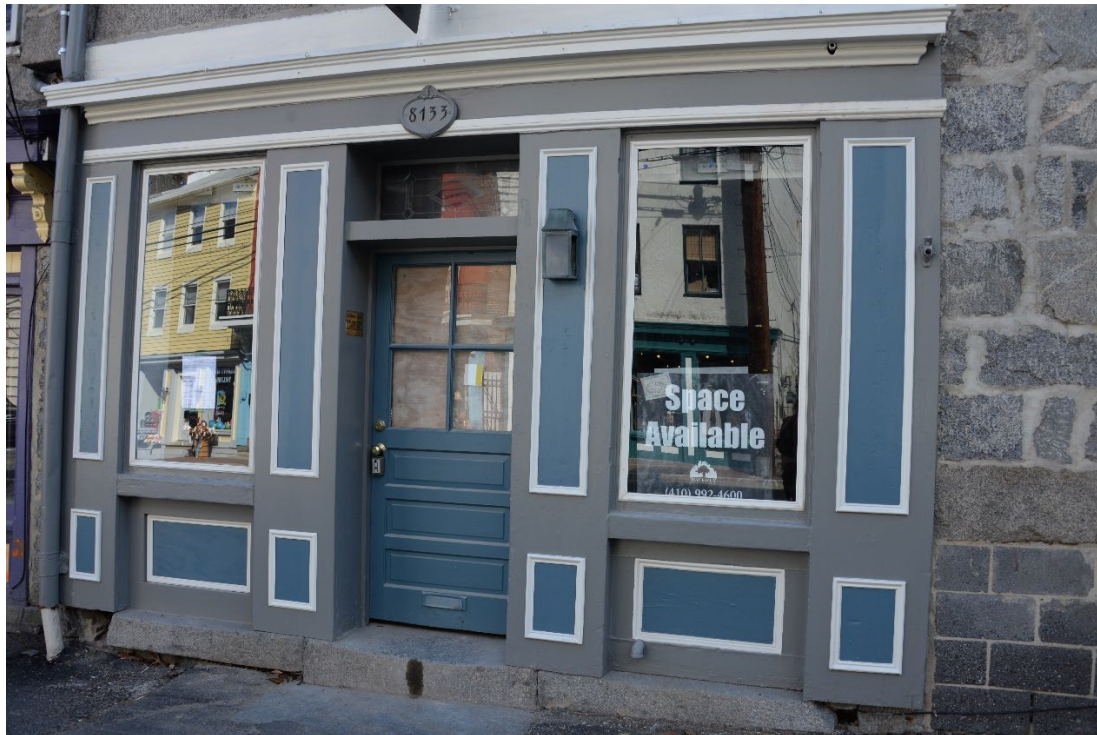
Photo 2 of 19: North elevation, storefront. 3/2/2017
