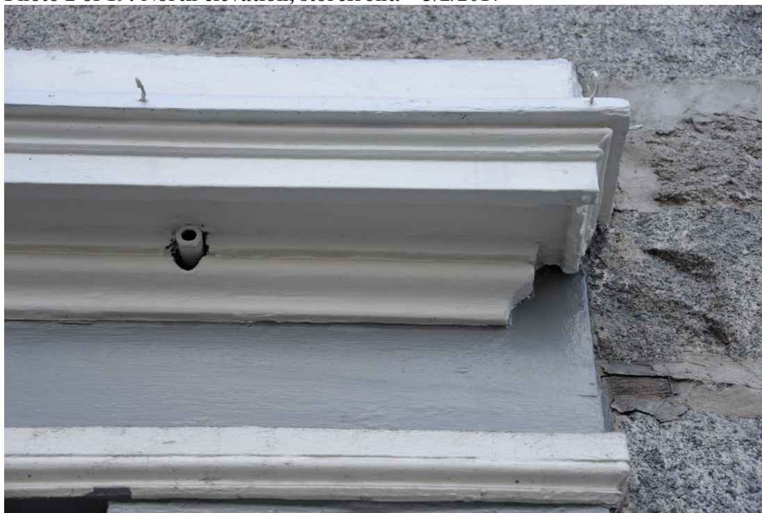
Photo 3 of 19: North elevation, storefront cornice detail. 3/2/2017
