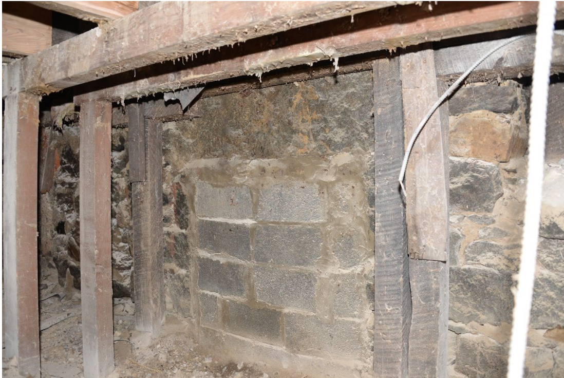
Photo 15 of 19: Basement, main block, fireplace on south wall. 2/24/2017
