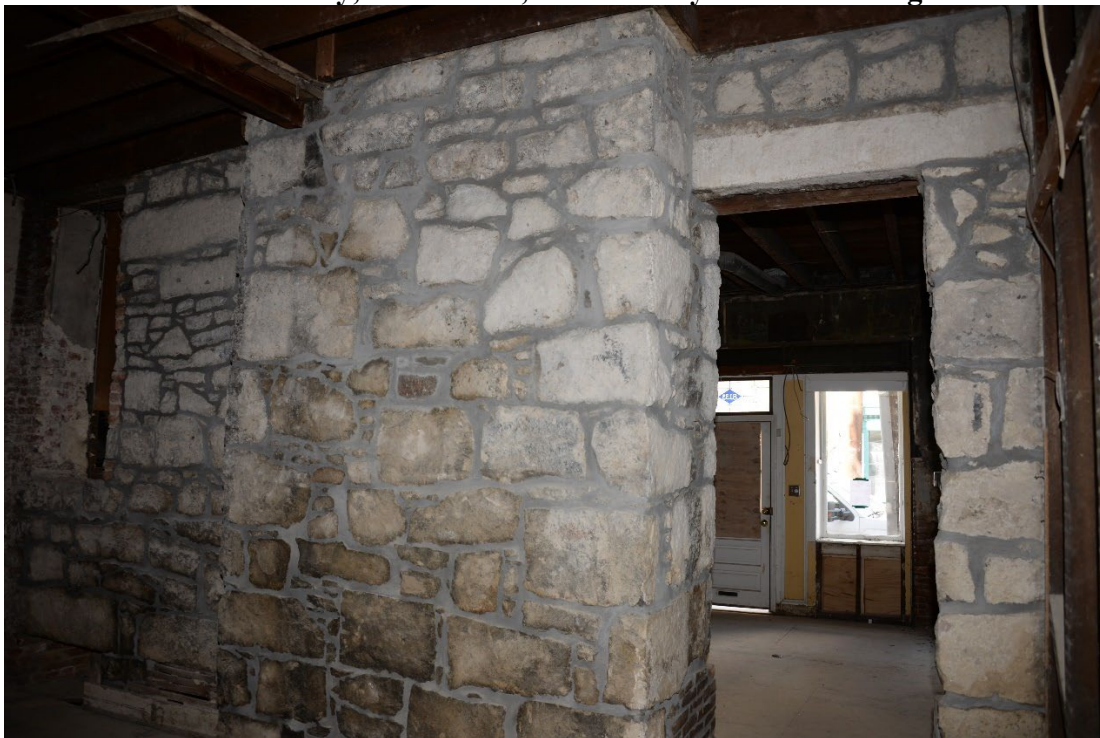
Photo 10 of 19: First story, main block, south elevation captured by addition. 2/15/2017
