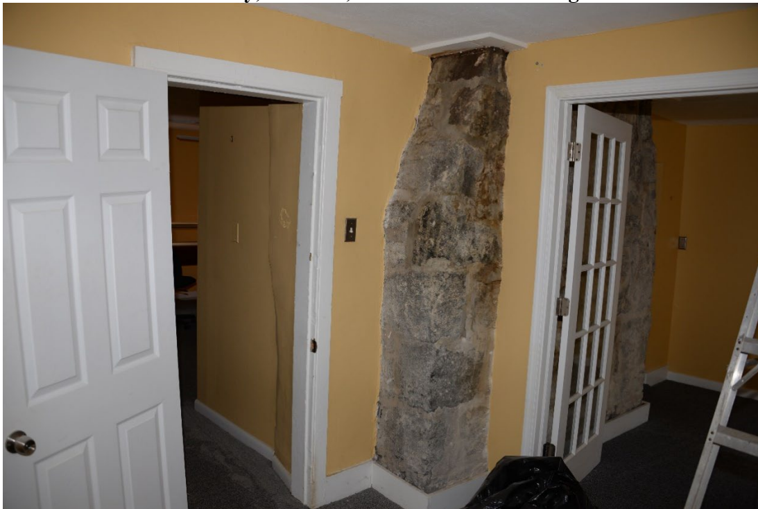
Photo 14 of 19: Second story, south elevation now captured by addition. 2/15/2017
