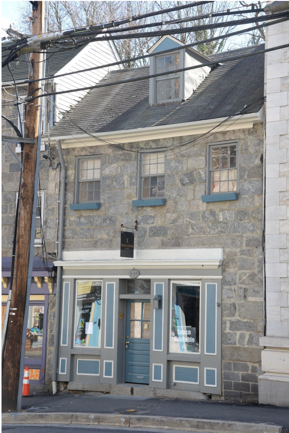
Photo 1 of 19: North elevation. 3/2/2017
