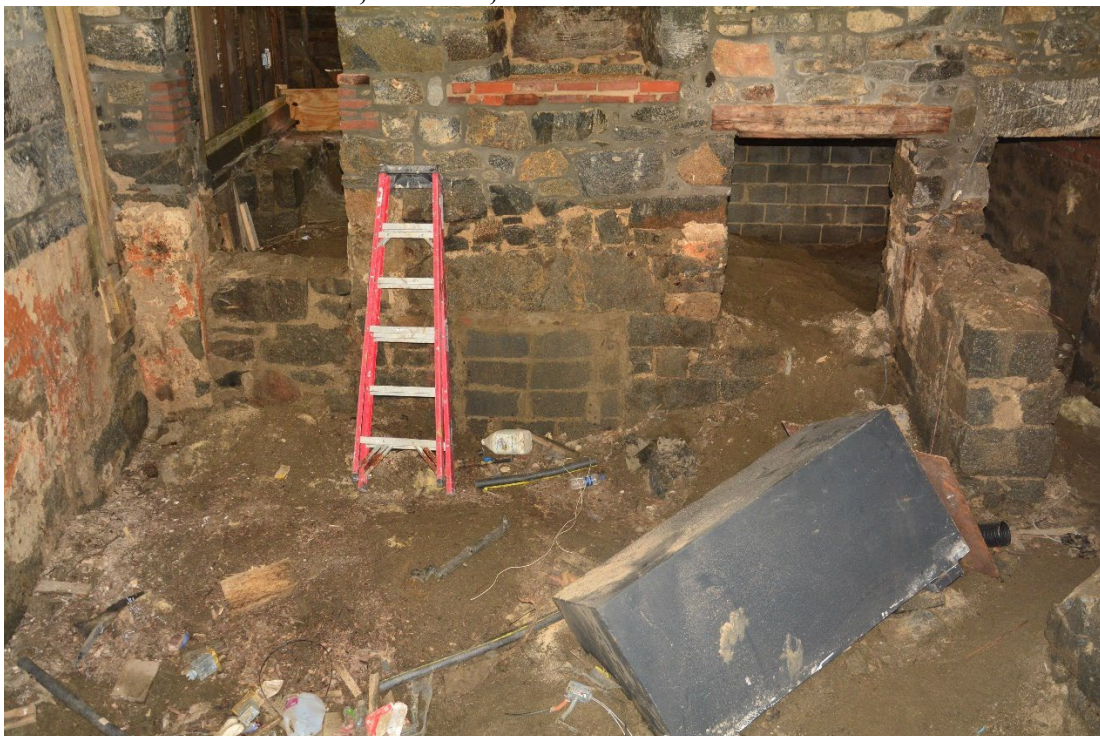
Photo 18 of 19: Basement, main block, view south after floor was removed. 8/18/2018
