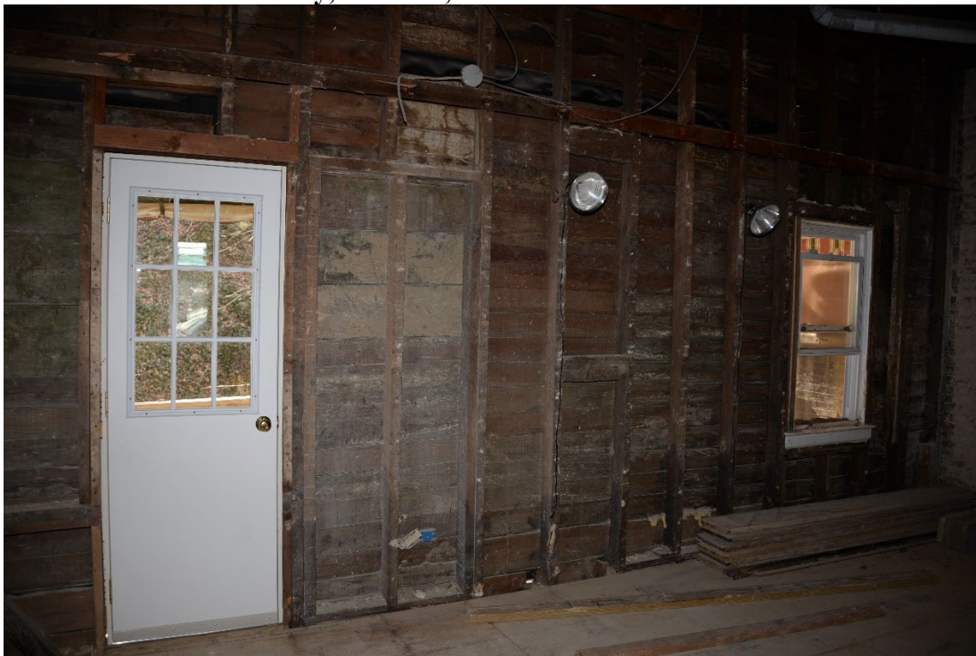
Photo 12 of 19: First story, addition, south wall. 2/15/2017
