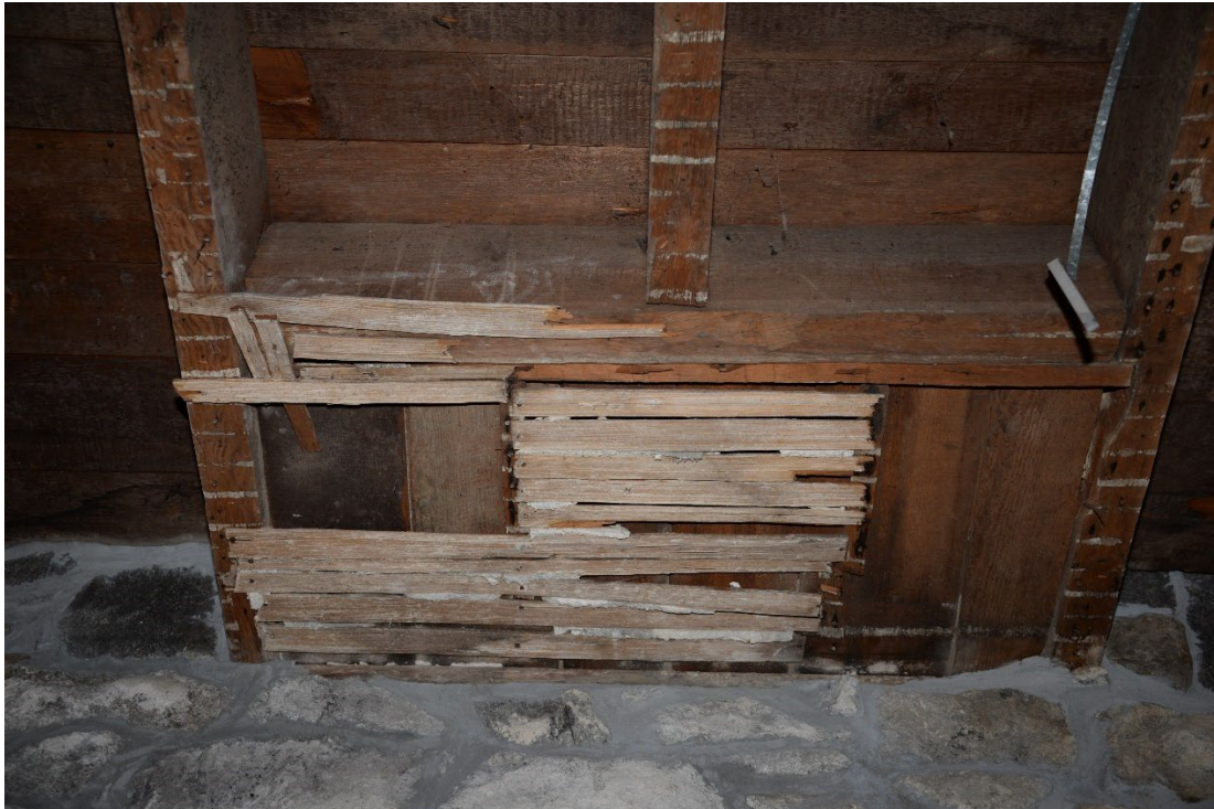
Photo 9 of 19: First story, main block, second story hearth framing. 2/15/2017
