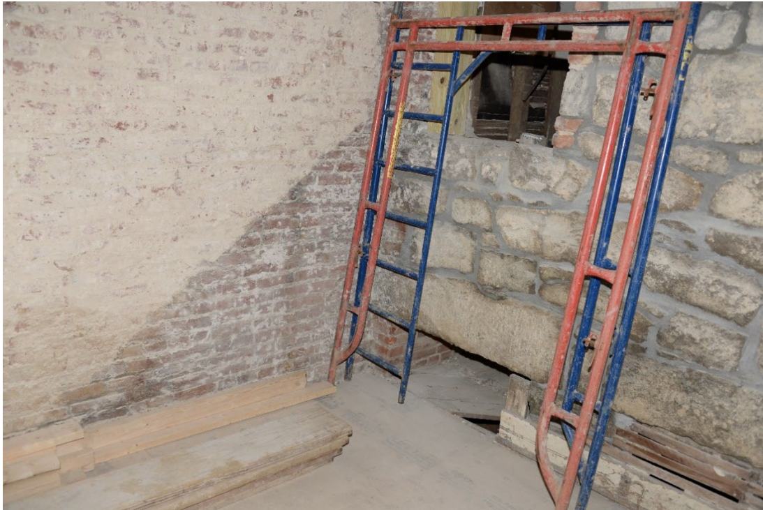
Photo 13 of 19: First story, addition, northeast corner with ghost of stair. 2/24/2017
