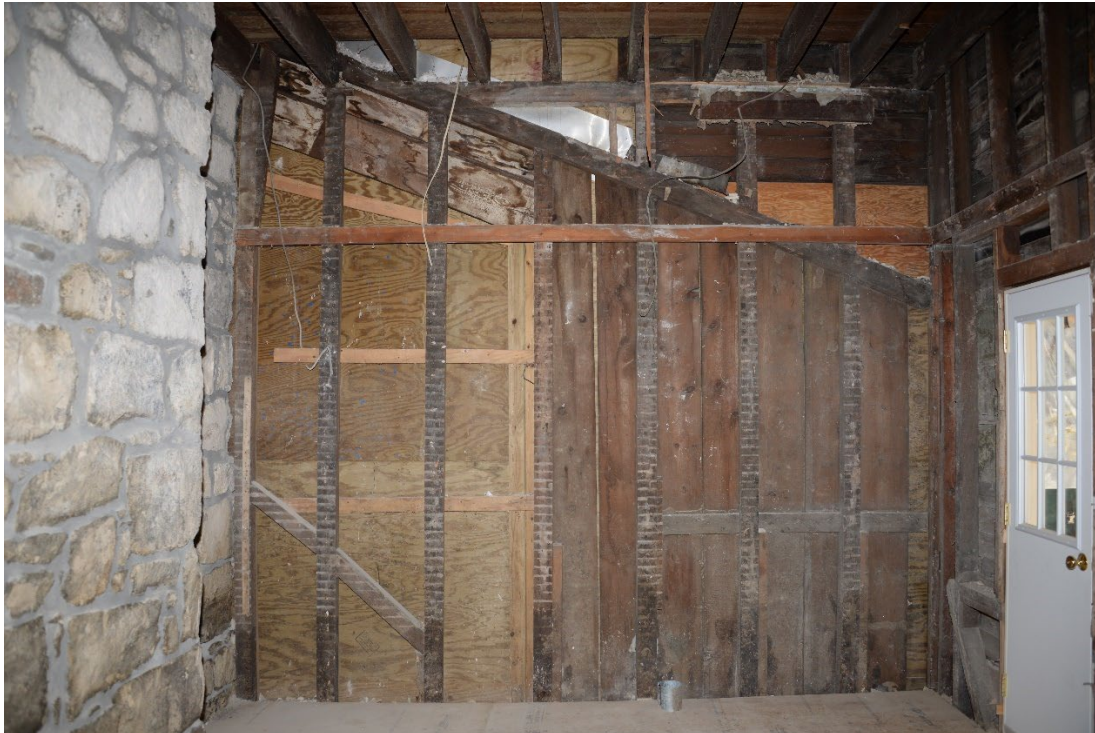
Photo 11 of 19: First story, addition, east wall. 2/15/2017
