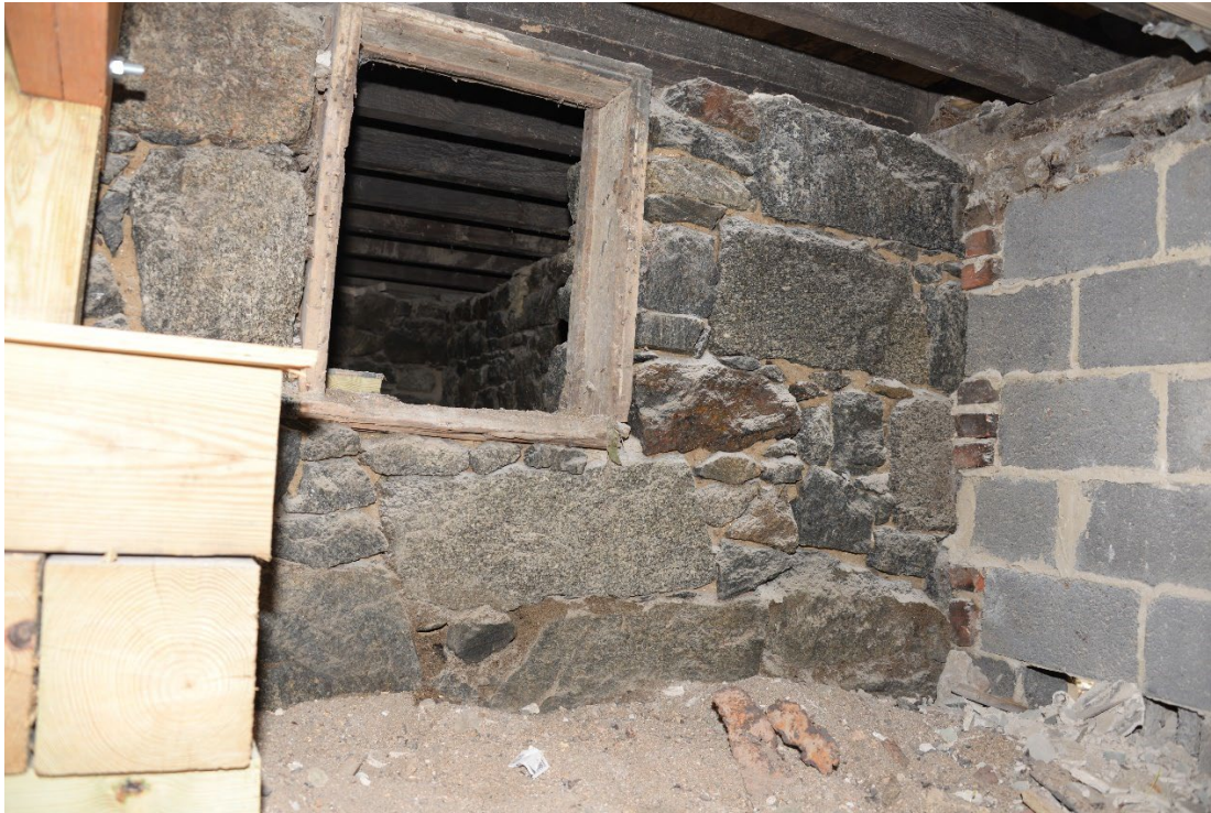
Photo 17 of 19: Basement, addition, west elevation. 2/24/2017
