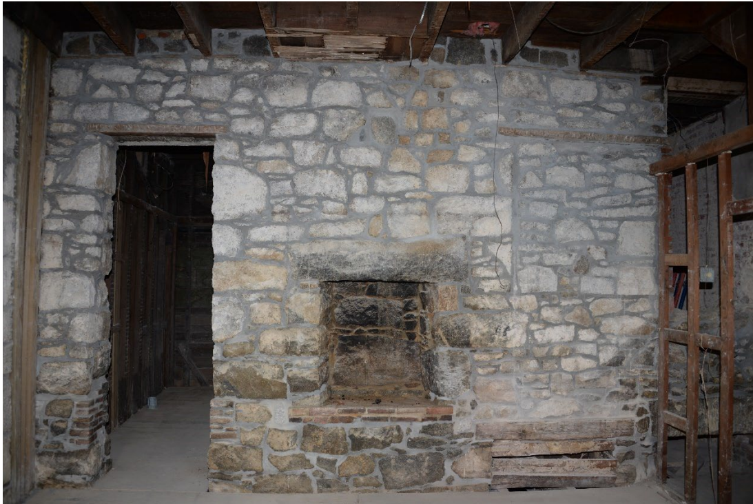
Photo 5 of 19: First story, main block, south wall. 2/15/2017
