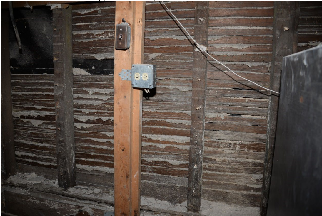
Photo 8 of 19: First story, main block, west wall. 2/15/2017
