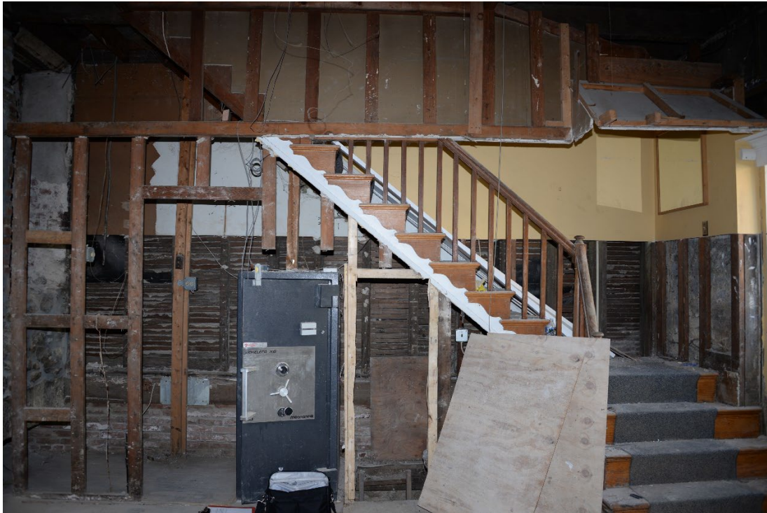
Photo 7 of 19: First story, main block, view west. 2/15/2017
