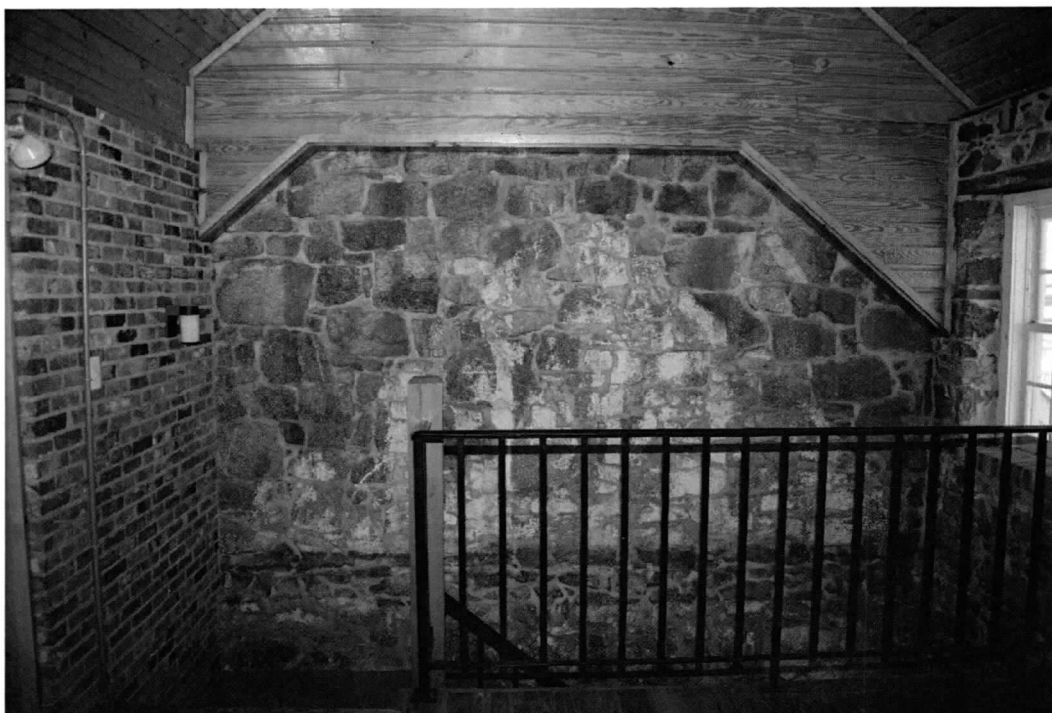
Photo 8 of 10: Third story, west elevation. 9/15/2016
