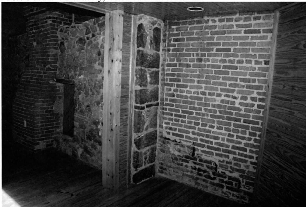
Photo 9 of 10: Third story, south and east walls, view northeast from addition. 9/15/2016
