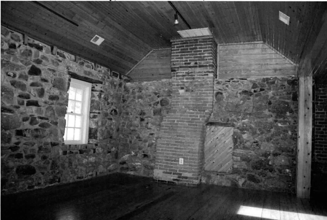
Photo 7 of 10: Third story, view northeast. 9/15/2016
