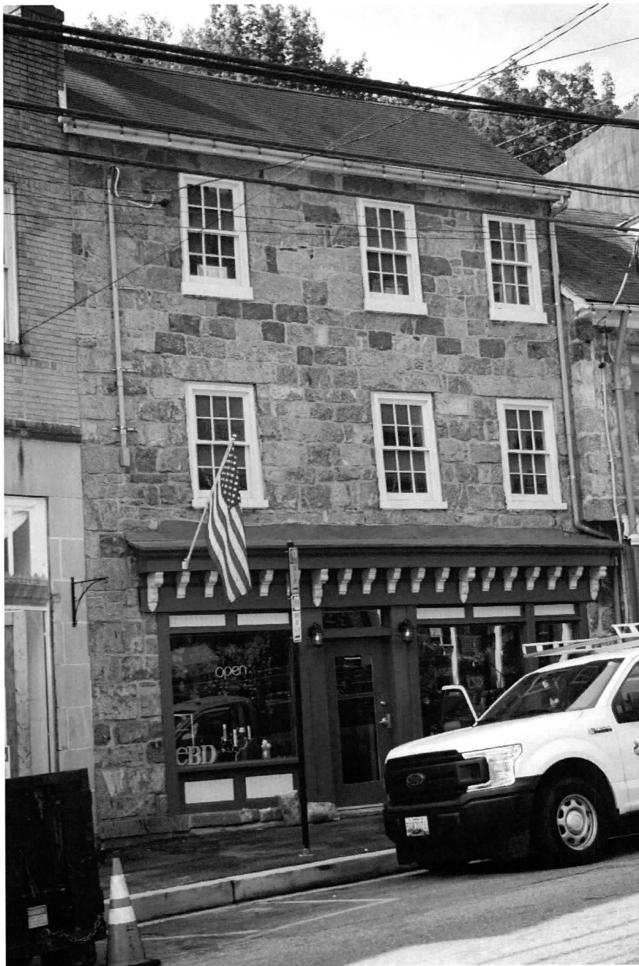
Photo 1 of 10: North elevation. 8/25/2020
