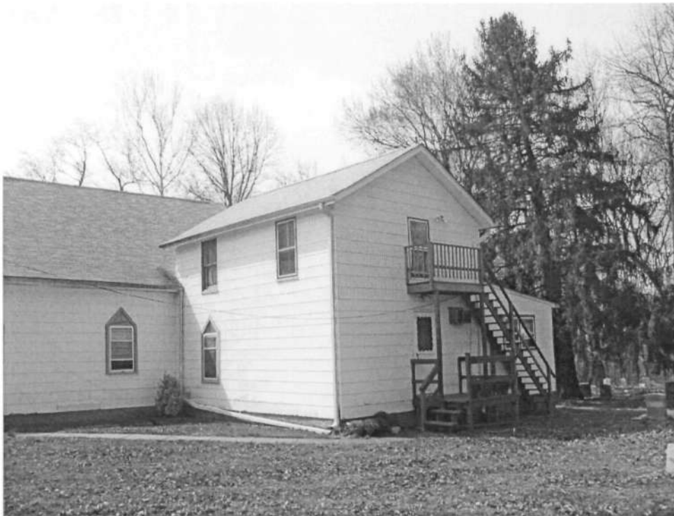
North elevation and north wing
