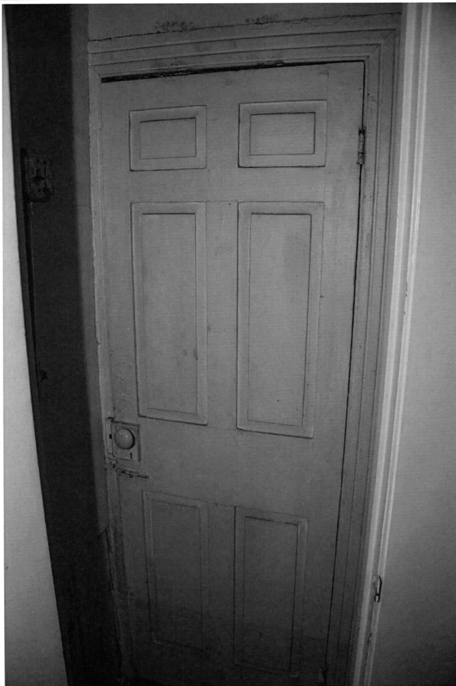
Photo 12 of 19: 8329 – South room, door to cellar. 8/2/2021
