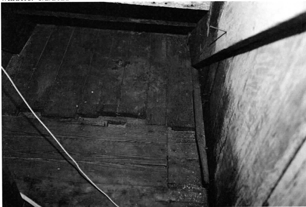
Photo 14 of 19: 8329 – South room, floor under stairs with mortises for south wall studs. 8/2/2021
