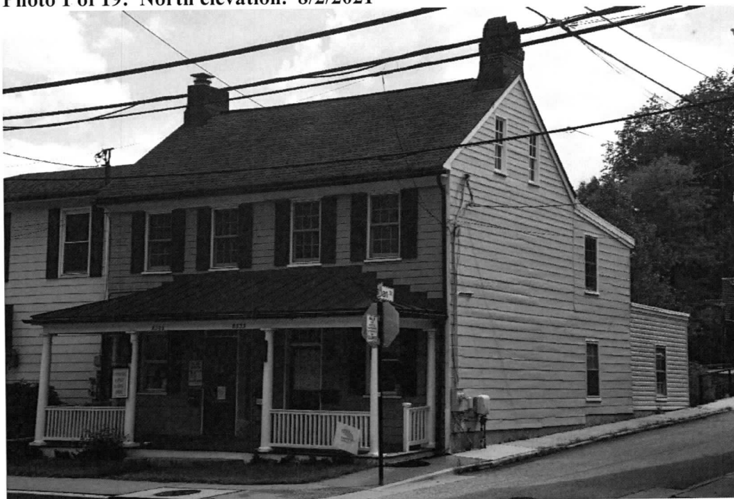
Photo 2 of 19: North & west elevations. 8/2/2021
