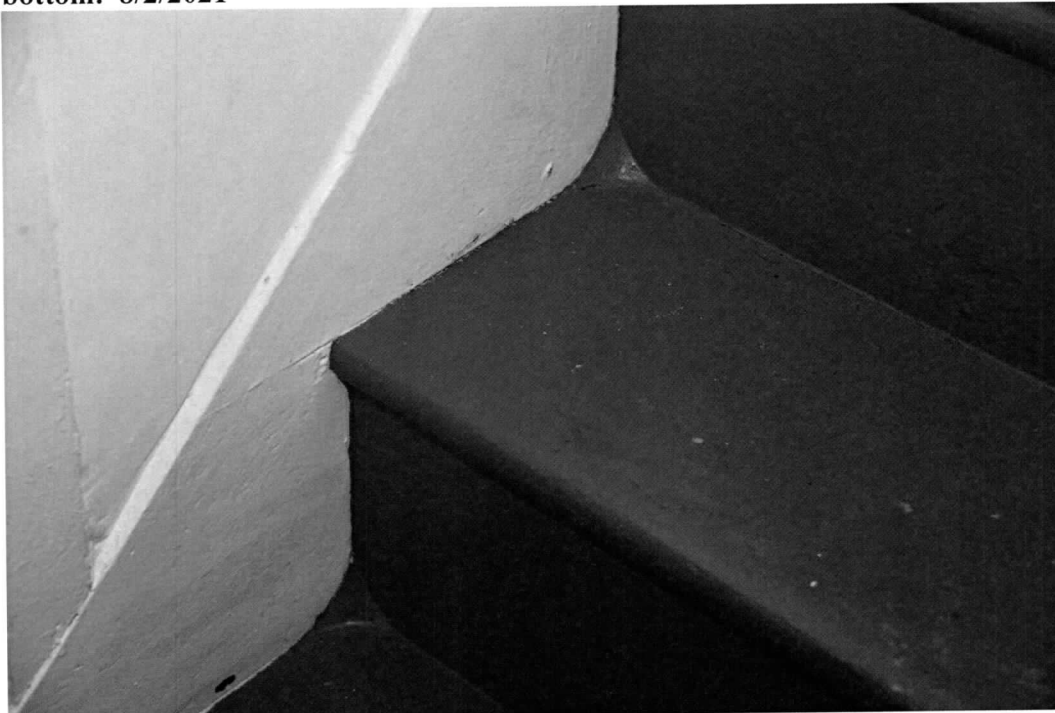
Photo 8 of 19: 8333 – South room stairs showing dust corners. 8/2/2021
