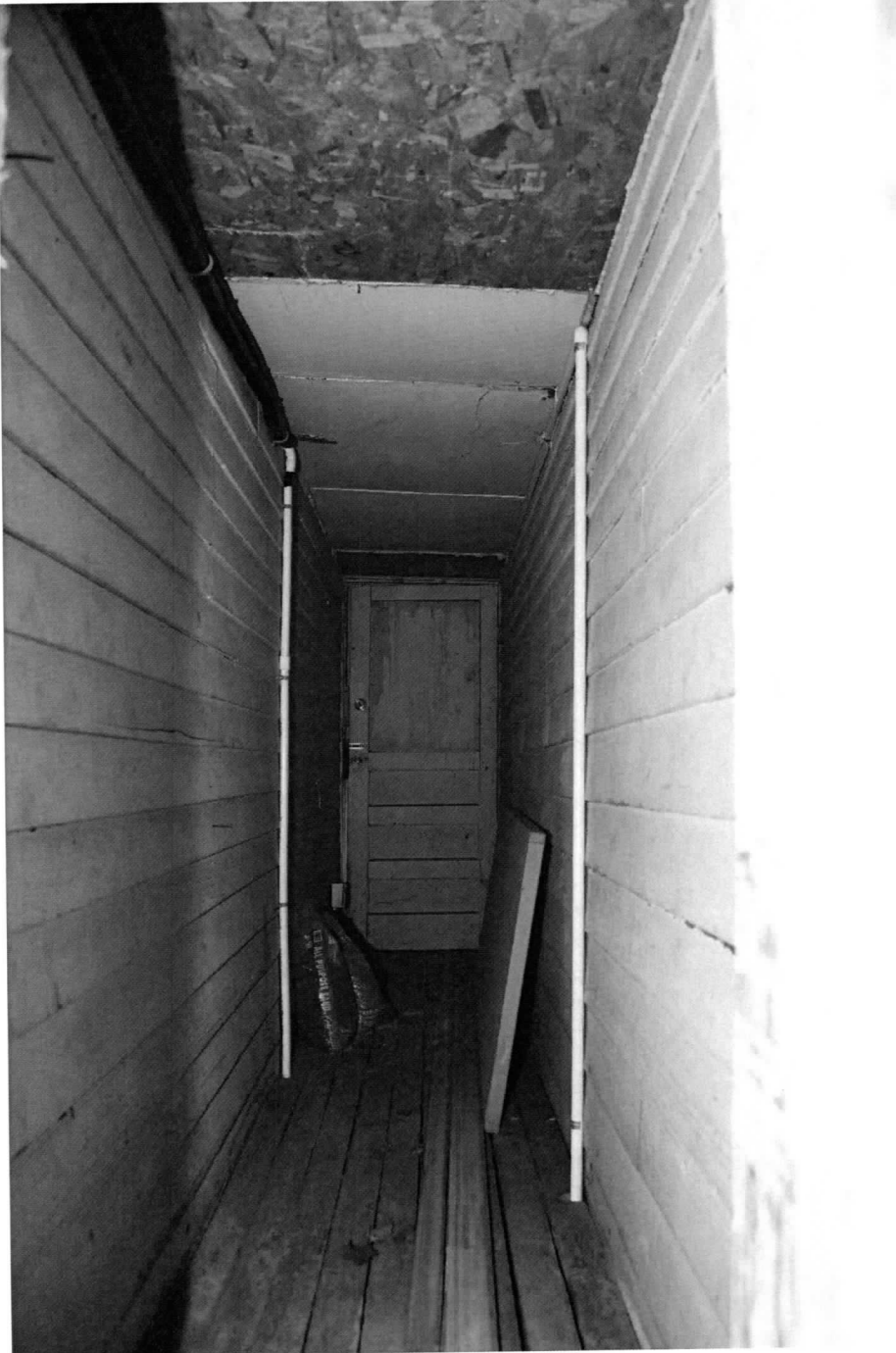
Photo 4 of 19: Sallyport, first story, view north. 8/2/2021
