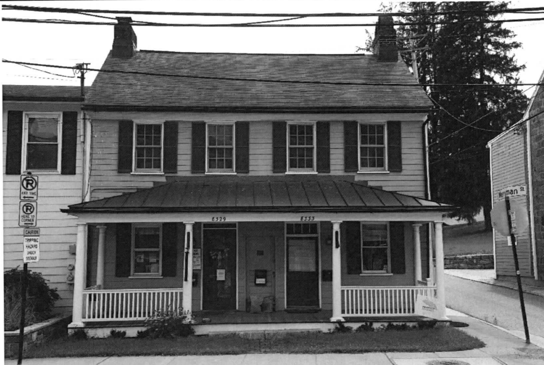
Photo 1 of 19: North elevation. 8/2/2021
