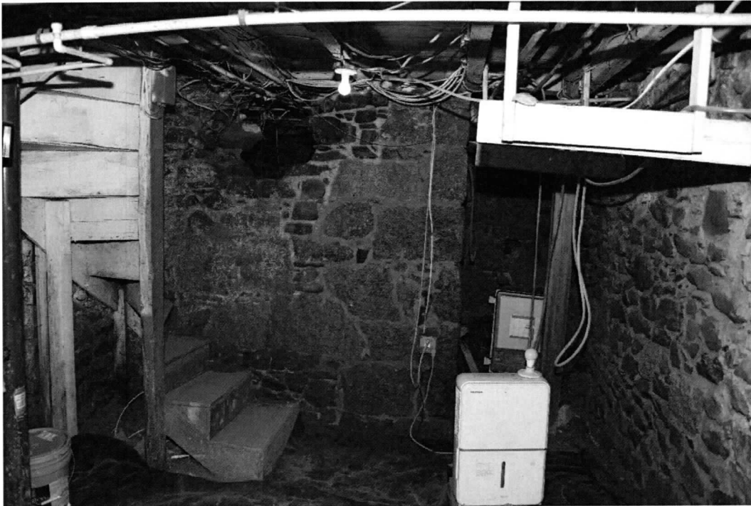
Photo 19 of 19: 8329 – Cellar, view south. 8/2/2021
