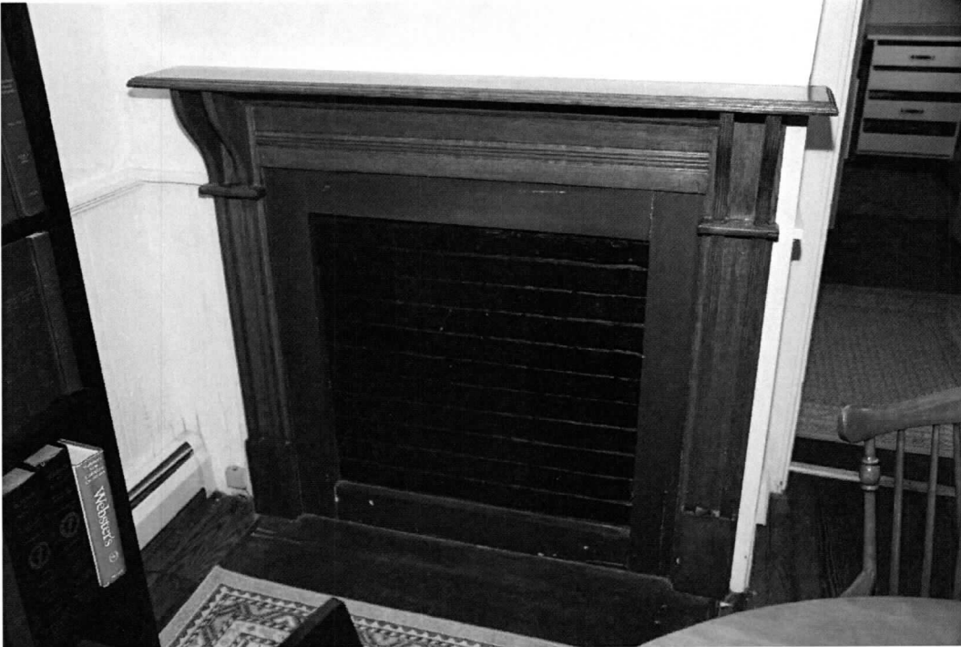
Photo 15 of 19: 8329 – Ell, fireplace on south. 8/2/2021
