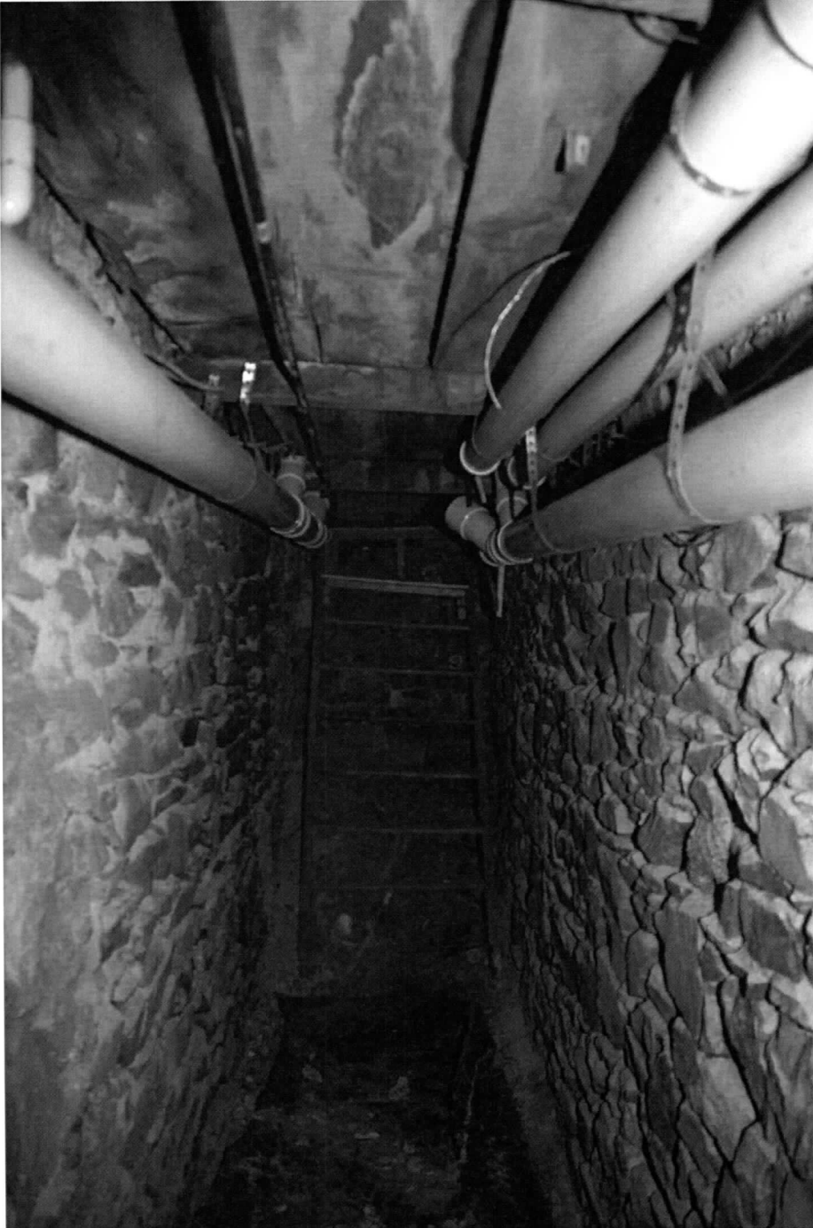
Photo 18 of 19: Sallyport, basement, view south. 1/18/2015
