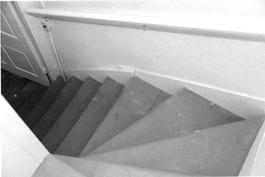
Photo 7 of 19: 8333 – South room stairs, view down from second story showing alteration at bottom. 8/2/2021
