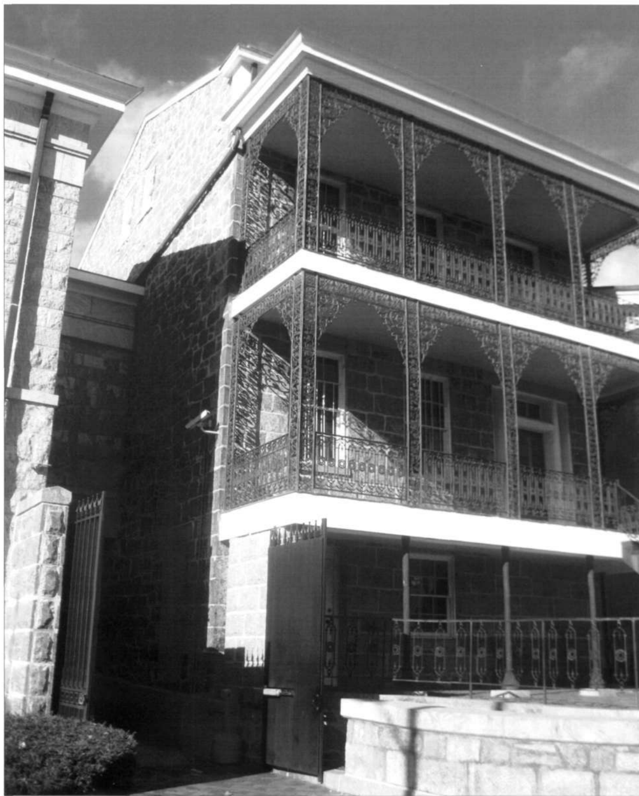
HO-284 Oak Lawn (Hayden House, former Board of Ed. Building) 8360 Court Place, Ellicott City Photos by Jennifer K. Cosham, 12/5/2012 South elevation
