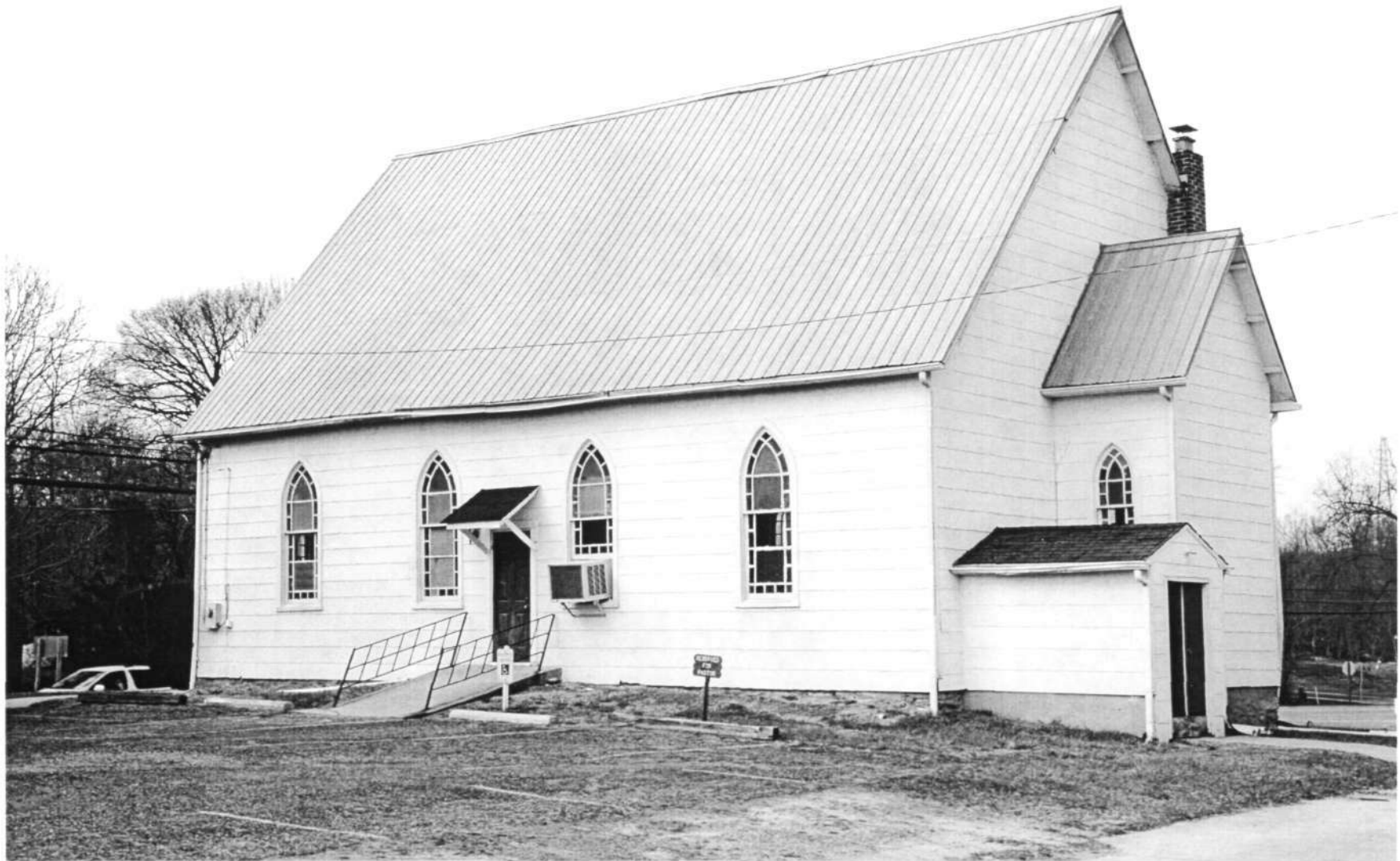
HO-0276 Mt. Gregory United Methodist Church 2325 Maryland Route 97, South & east elevations Ken Short, March 2006 4/11
