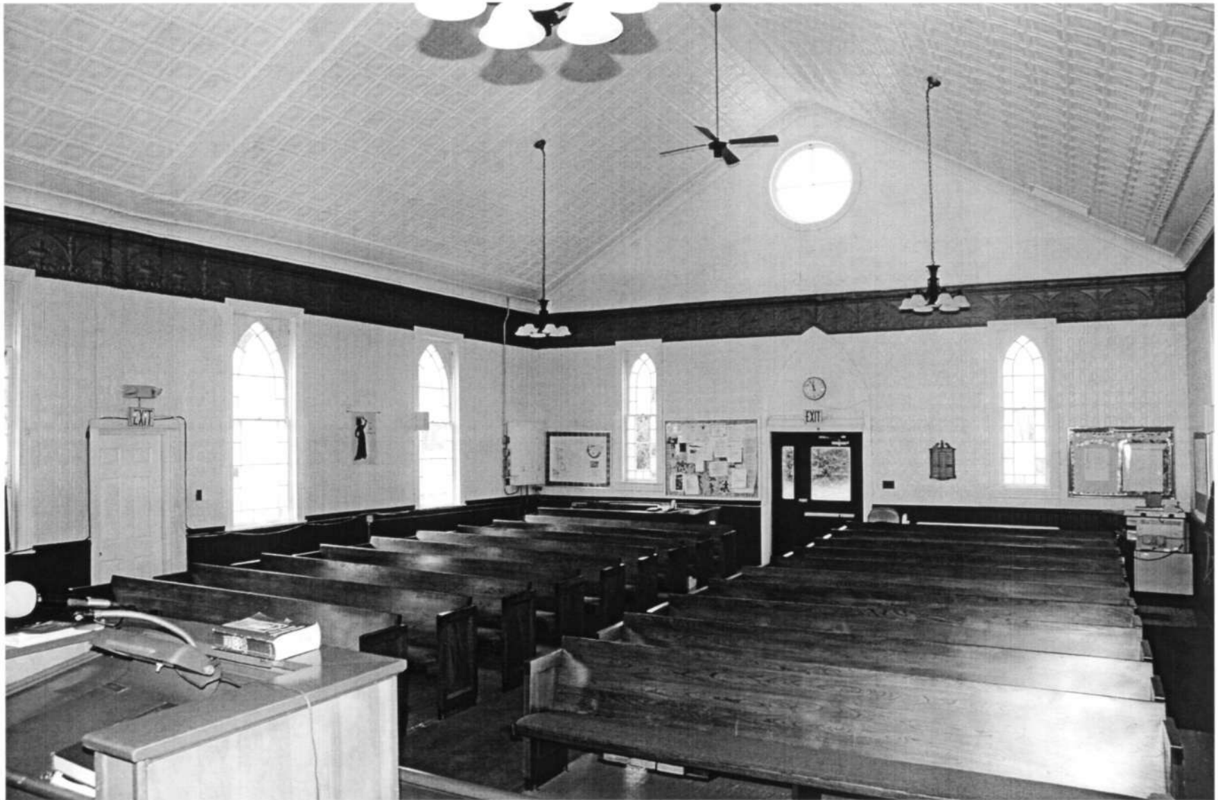
HO-0276 Mt. Gregory United Methodist Church 2325 Maryland Route 97, Interior, view southwest Ken Short, March 2006 7/11
