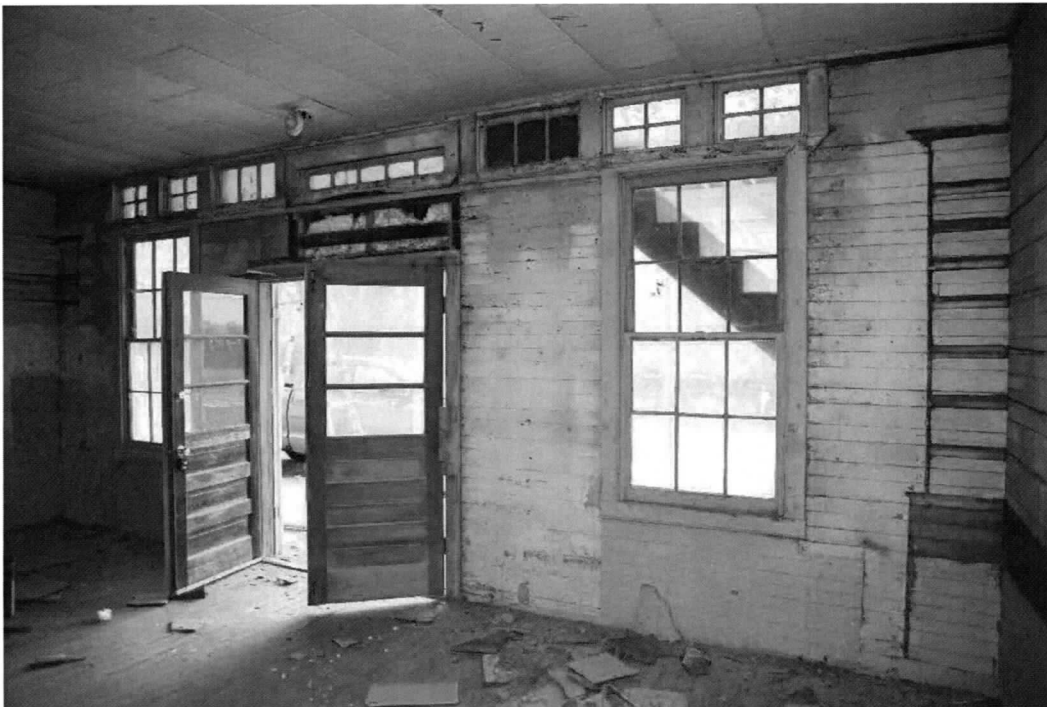
Photo 1 of 13: Store interior, south elevation. 5/14/2020
