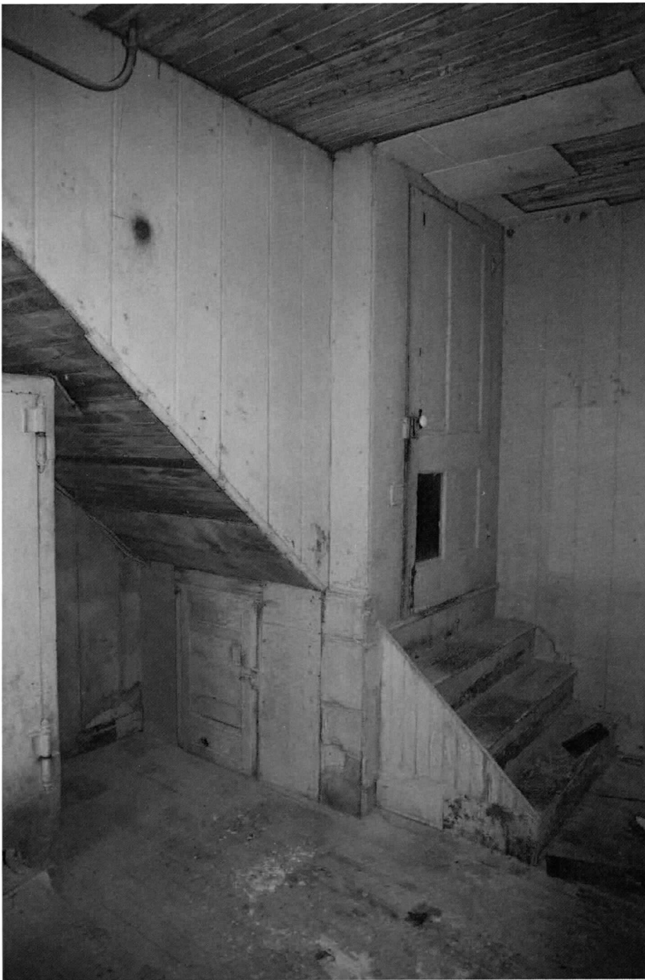
Photo 7 of 13: Store interior, stairway in northeast corner. 5/14/2020
