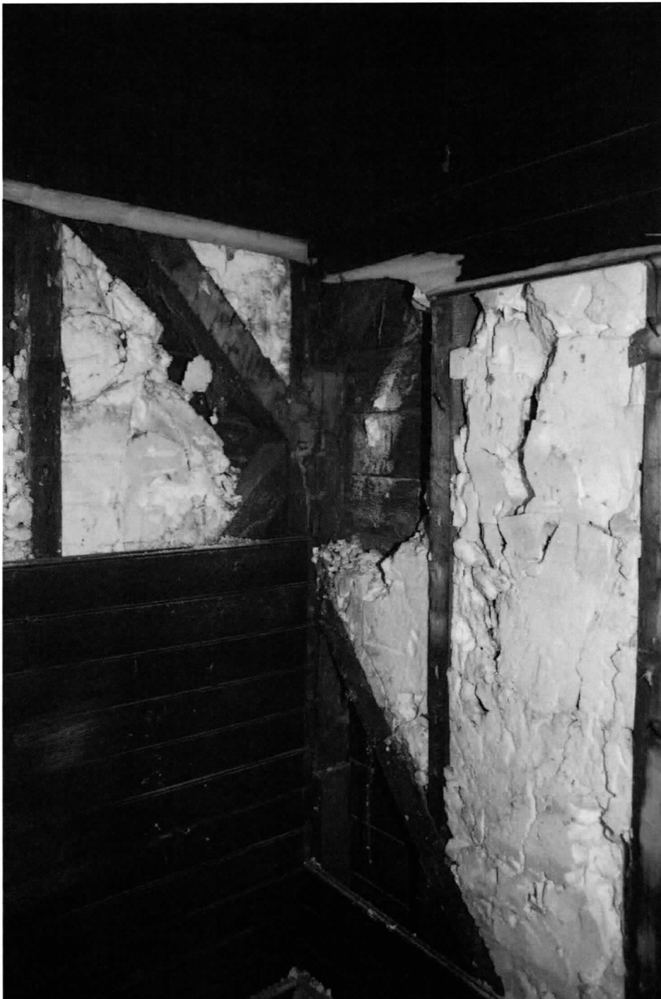
Photo 10 of 13: Store interior, second story, southeast corner framing. 5/14/2020
