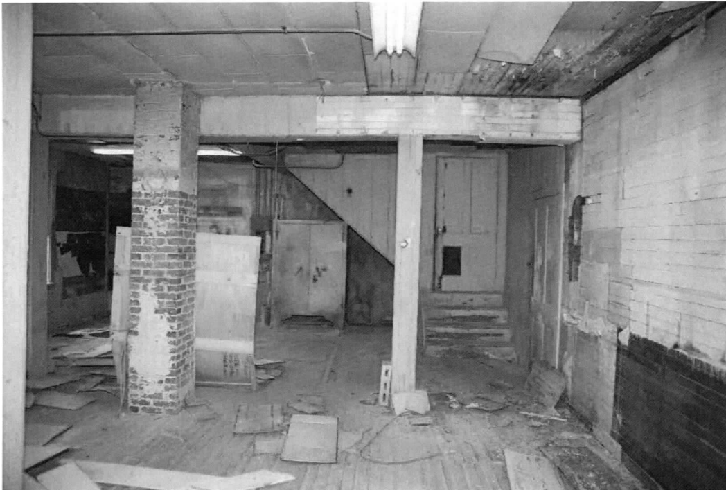
Photo 5 of 13: Store interior, north elevation. 5/14/2020
