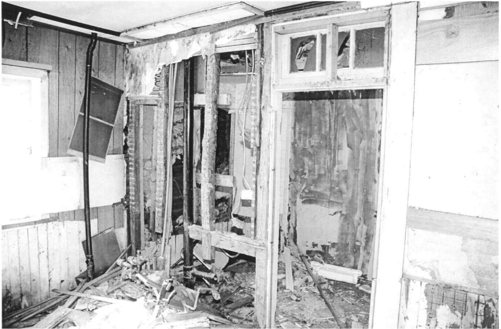
HO-0253 Old Florence School 3055 Florence Road, interior, view south toward vestibule Ken Short, April 2006 6/9
