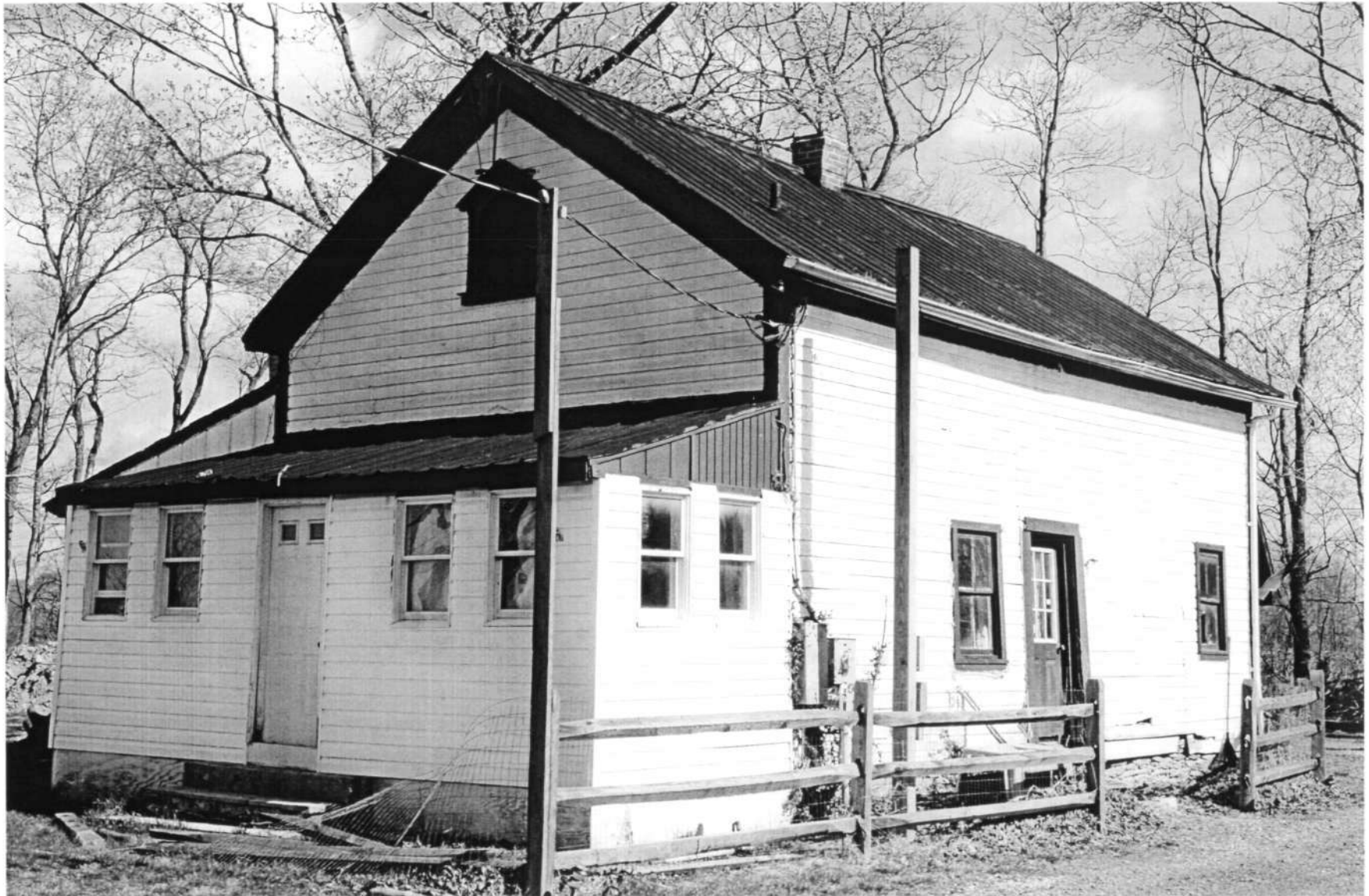
HO-0253 Old Florence School 3055 Florence Road, Southwest & southeast elevations Ken Short, April 2006 1/9
