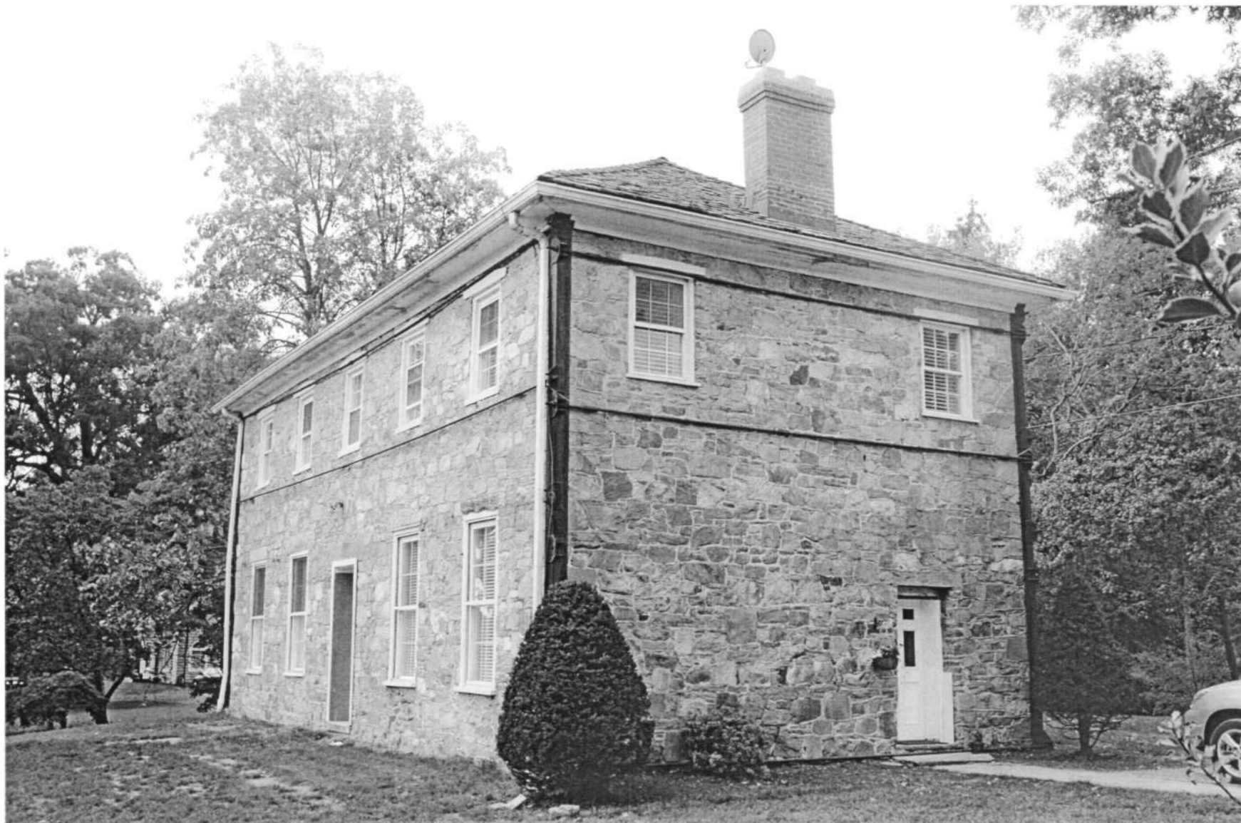
HO-238 "Glenelg" Gardener's House 12789 Folly Quarter Road Southeast & northeast elevations Ken Short, September 2006 4/6
