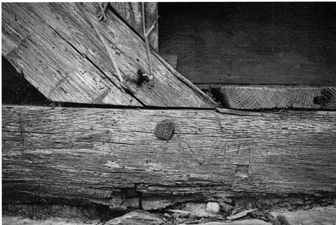
Photo 5 of 20: East elevation, down-brace & sill. 7/11/2018
