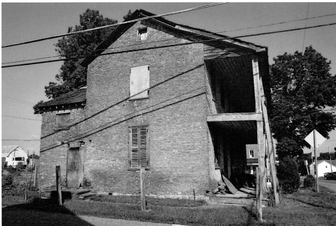
Photo 2 of 20: West elevation. 3/8/2019
