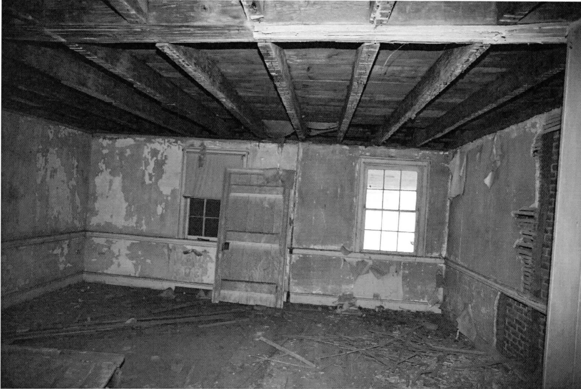
Photo 17 of 20: Second-story frame section, view south. 7/11/2018
