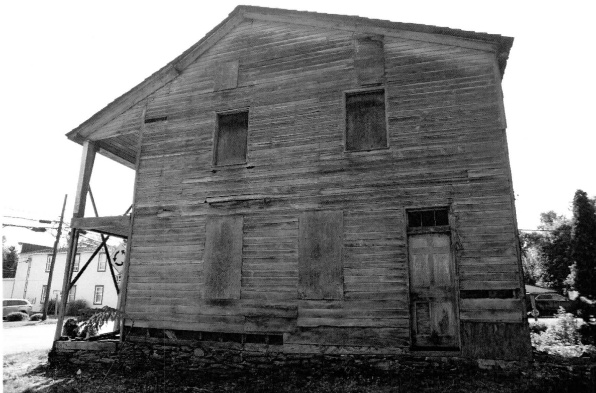
Photo 4 of 20: East elevation. 7/11/2018
