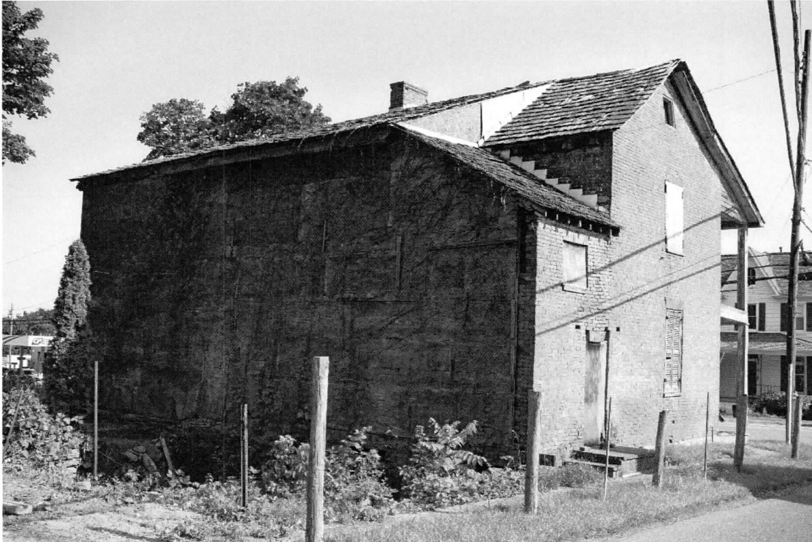
Photo 3 of 20: North & west elevations. 7/11/2018
