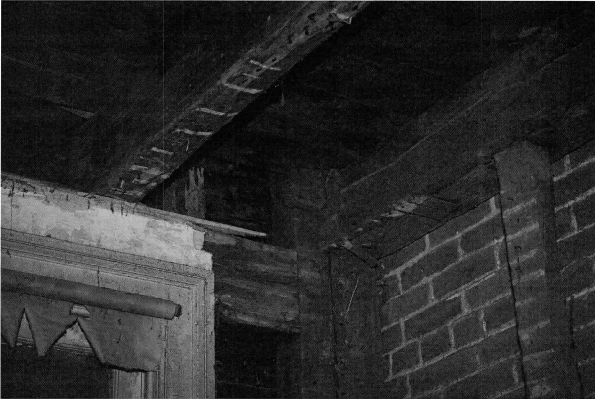
Photo 10 of 20: Southeast room, southwest guttered cornerpost detail. 7/11/2018
