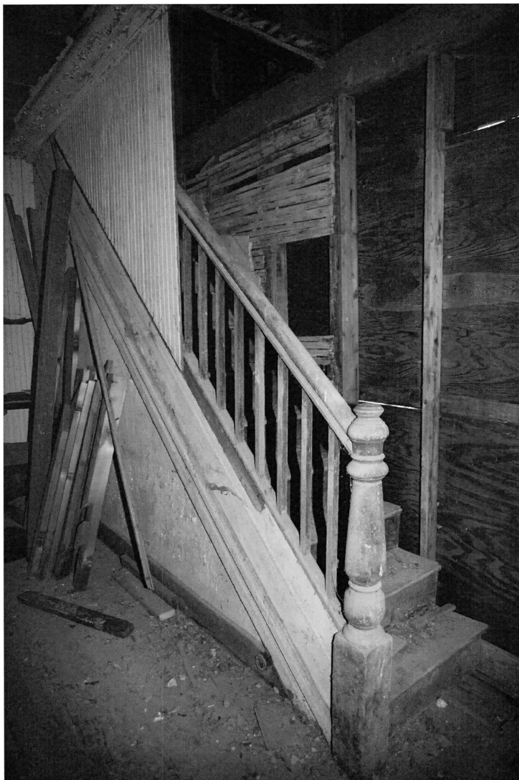
Photo 11 of 20: First story stairway, view northwest. 7/11/2018
