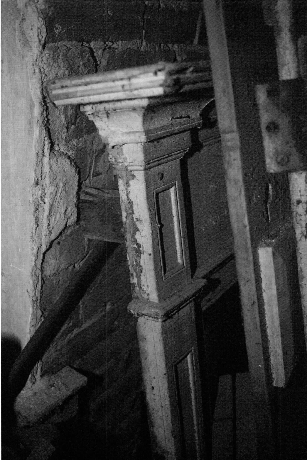
Photo 7 of 20: Southwest room, mantel detail. 7/11/2018
