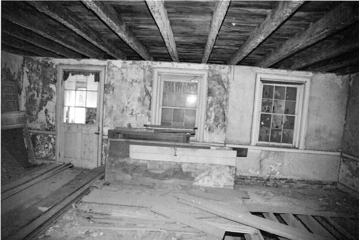
Photo 14 of 20: Second-story southwest chamber, view south. 7/11/2018
