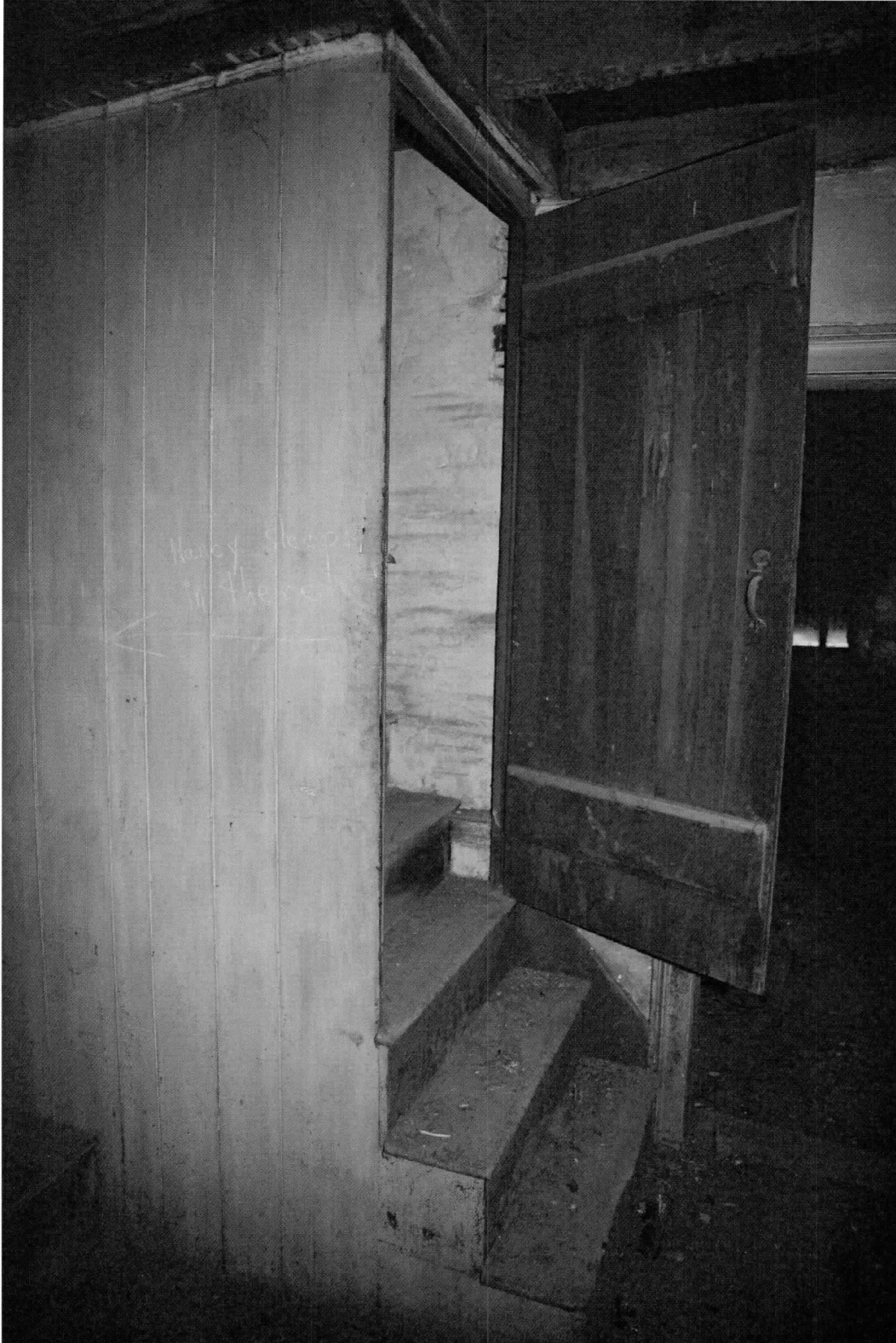
Photo 18 of 20: Second story, frame section, stairs to attic along west wall. 7/11/2018
