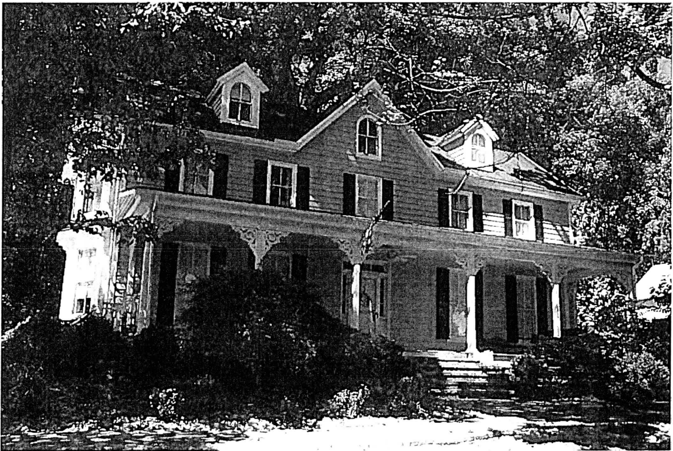
MD_HowardCounty_ForestView_0001.tif House, east elevation (September, 2013) 1 of 15
