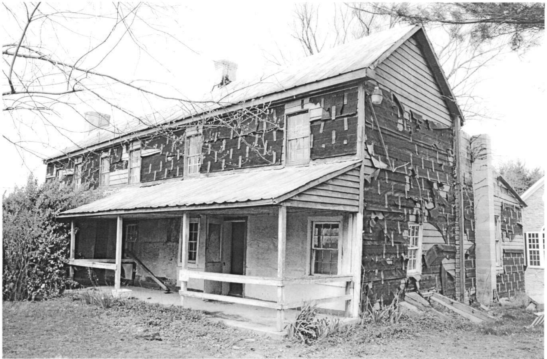
HO-183 Day House and Store 14040 Triadelphia Road South & east elevations Ken Short, April 2007 1/14
