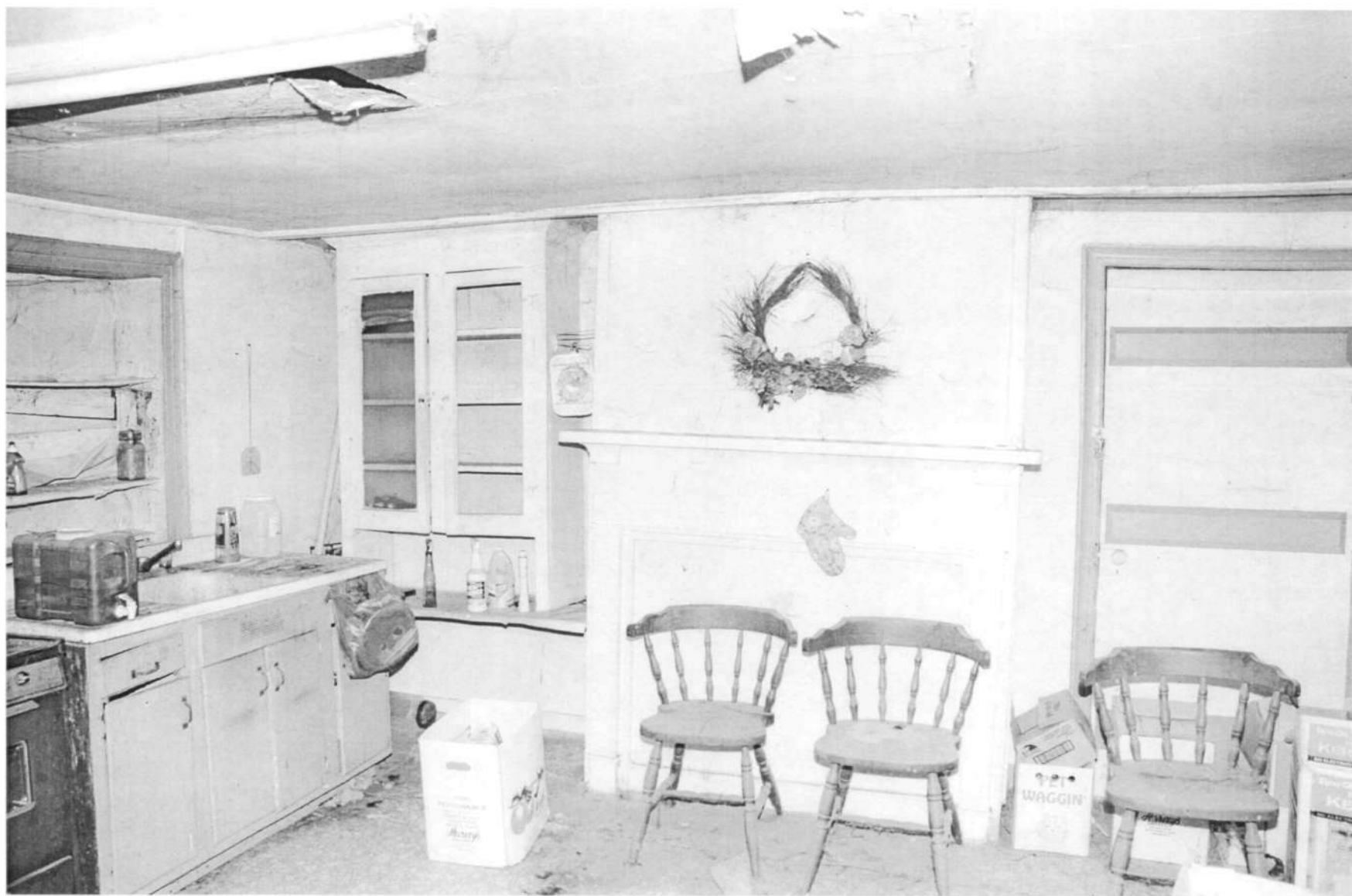
HO-183 Day House and Store 14040 Triadelphia Road Center room, east elevation Ken Short, April 2007 9/14
