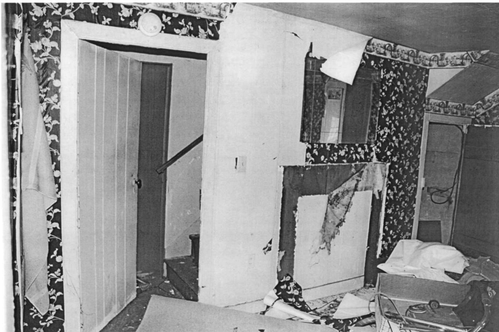
HO-183 Day House and Store 14040 Triadelphia Road East room, west elevation Ken Short, April 2007 8/14
