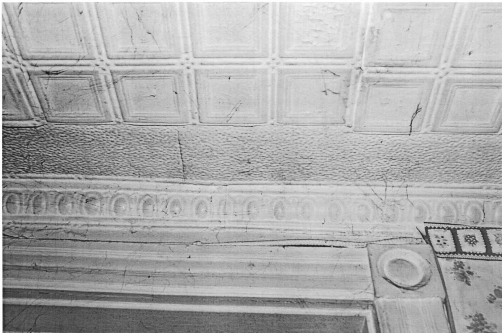
HO-183 Day House and Store 14040 Triadelphia Road Northeast addition, west room, ceiling & cornice detail Ken Short, April 2007 14/14
