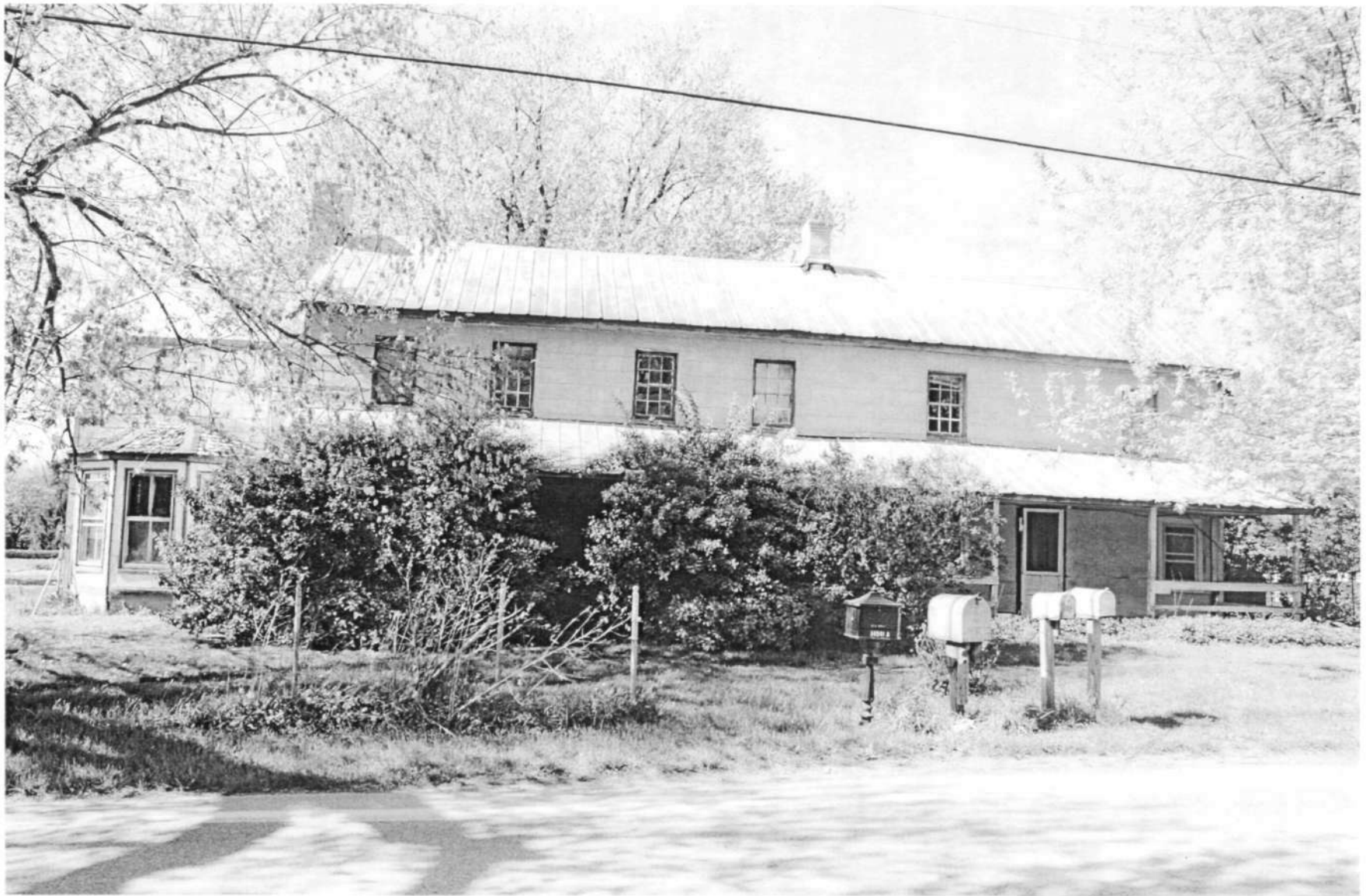
HO-183 Day House and Store 14040 Triadelphia Road South elevation Ken Short, April 2006 1/5
