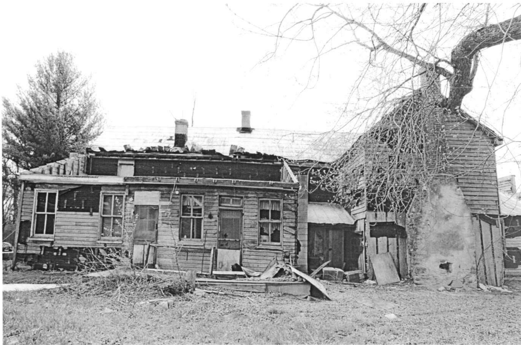
HO-183 Day House and Store 14040 Triadelphia Road North elevation Ken Short, April 2007 3/14
