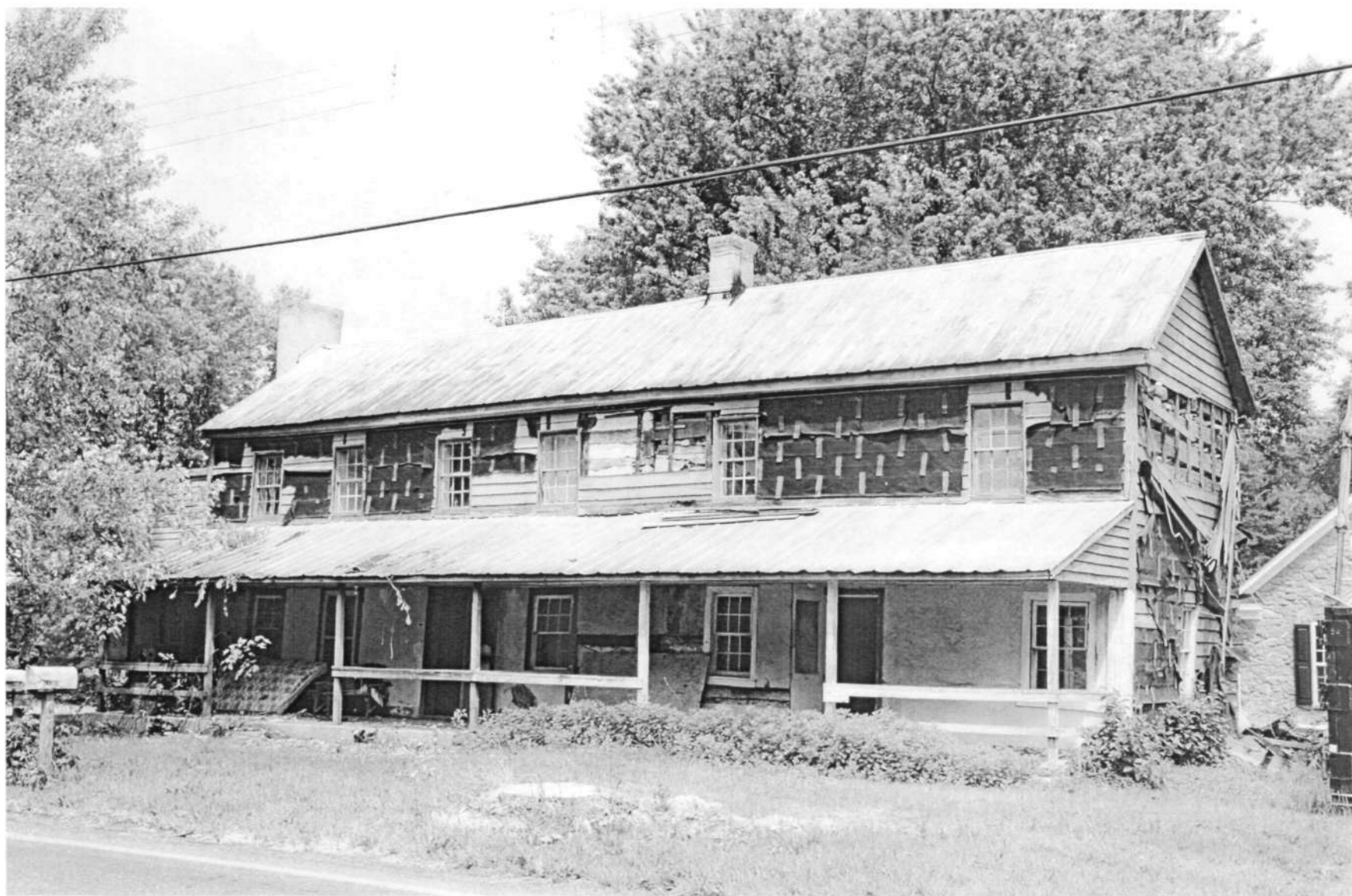
HO-183 Day House and Store 14040 Triadelphia Road South & east elevations Ken Short, June 2007 1/3
