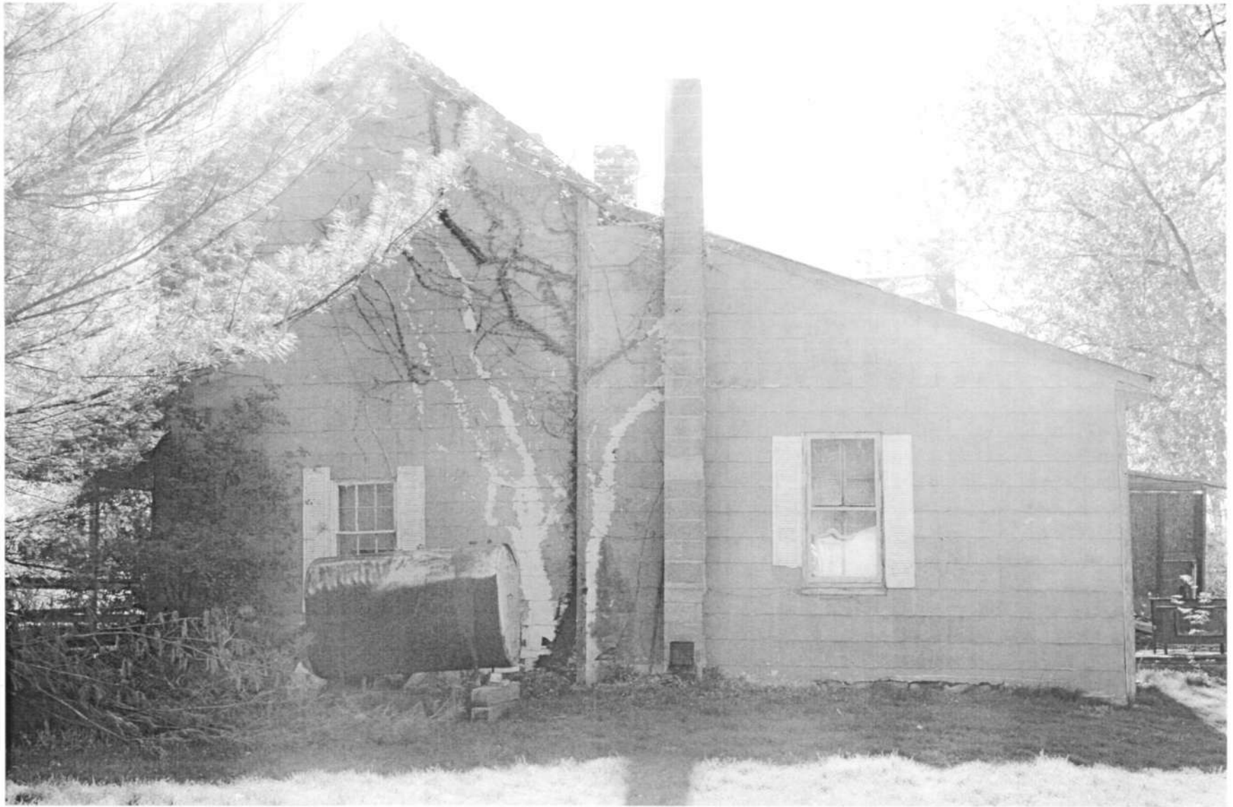
HO-183 Day House and Store 14040 Triadelphia Road East elevation Ken Short, April 2006 2/5
