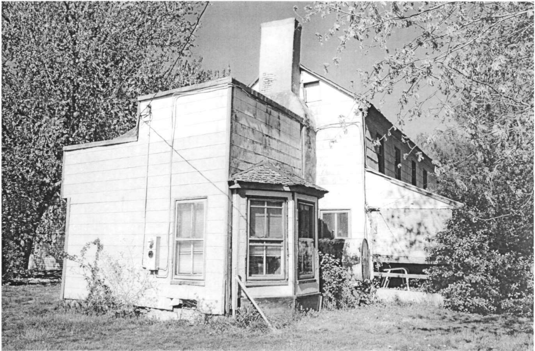
HO-183 Day House and Store 14040 Triadelphia Road West & south elevations Ken Short, April 2006 5/5
