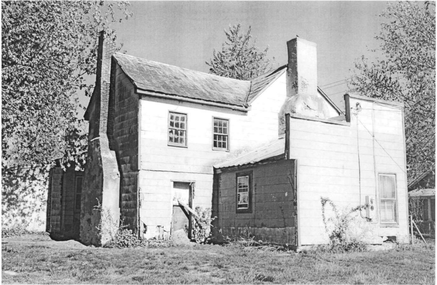
HO-183 Day House and Store 14040 Triadelphia Road North & west elevations Ken Short, April 2006 4/5
