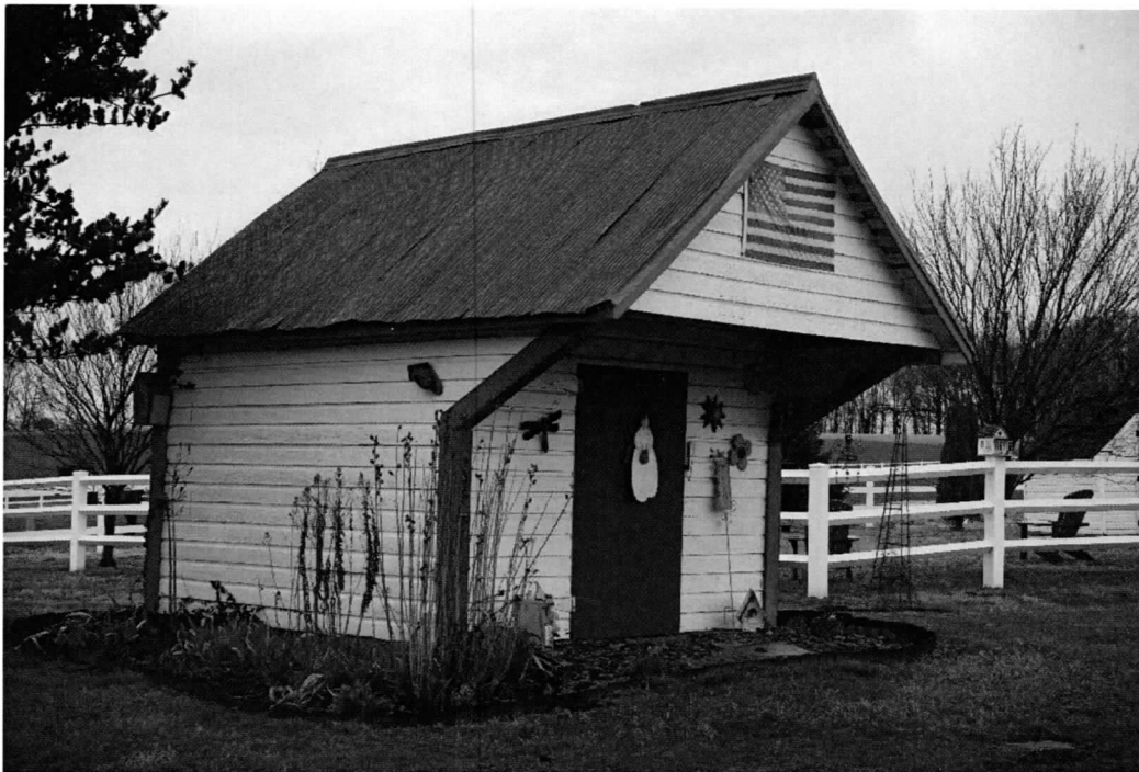
Photo 1 of 8: Smokehouse, southwest & southeast elevations.
