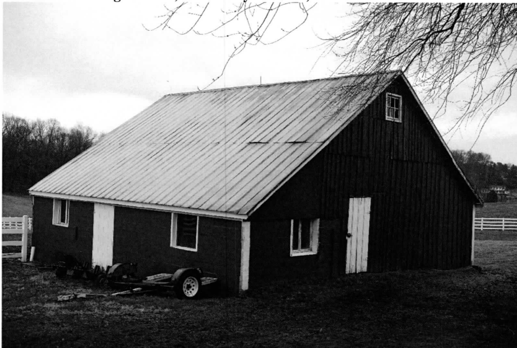
Photo 6 of 8: Hay Barn, northeast & northwest elevations.
