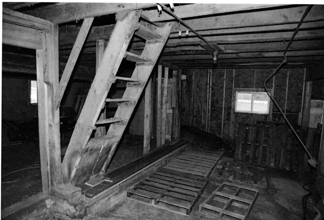
Photo 7 of 8: Hay Barn, interior, view southeast.
