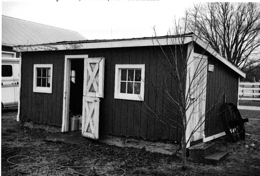
Photo 8 of 8: Poultry House, southeast & northeast elevations.
