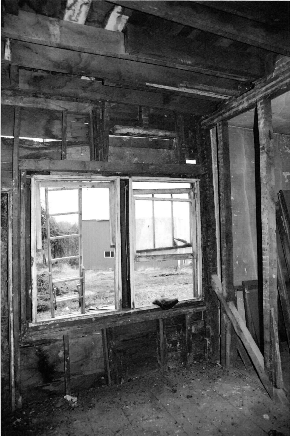
Photo 21 of 36: Wing east wall framing for original window, heavy timber braced frame of main block, and overhanging joists from main block. 12/27/2019
