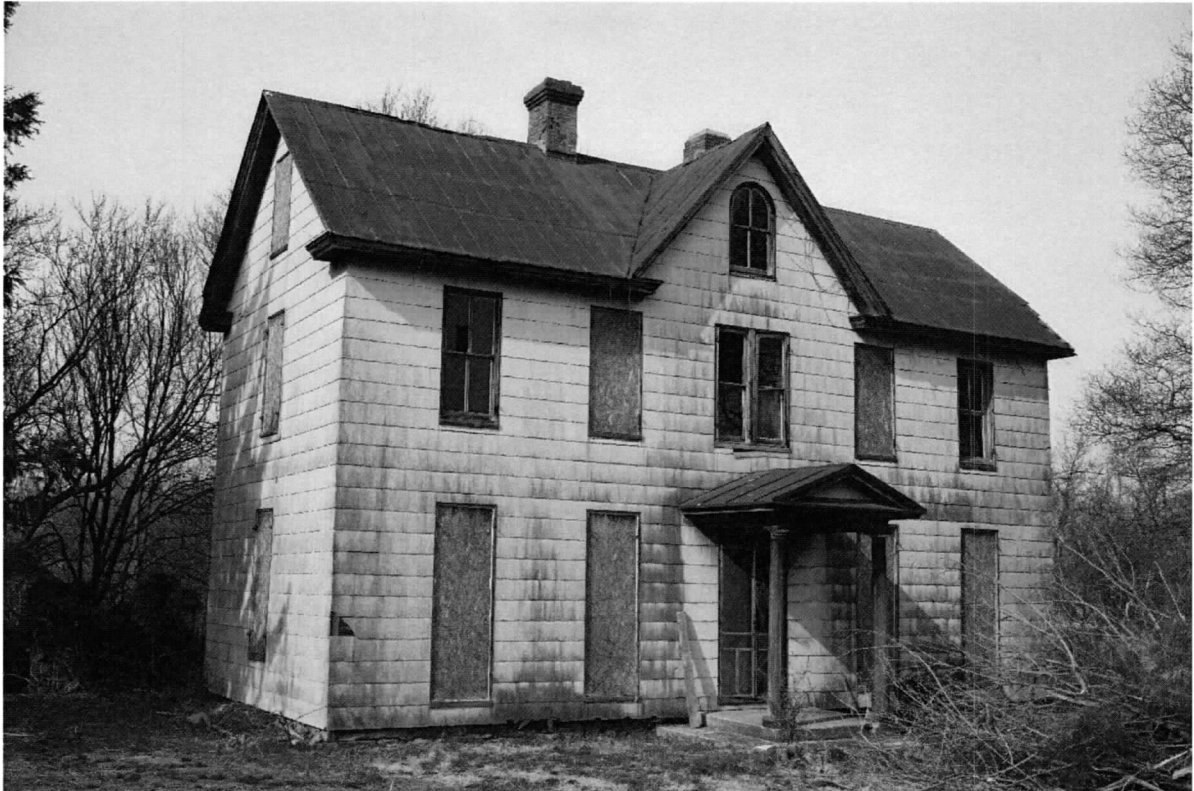
Photo 1 of 24: South elevation. 3/20/2019
