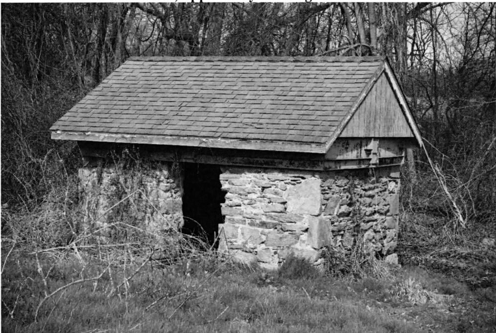
Photo 36 of 36: Springhouse, west & south elevations. 3/20/2019
