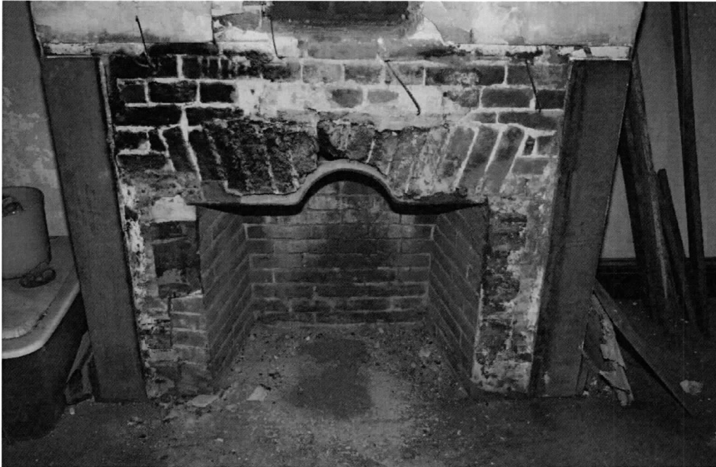
Photo 22 of 36: East room fireplace with mantel removed. 3/13/2020
