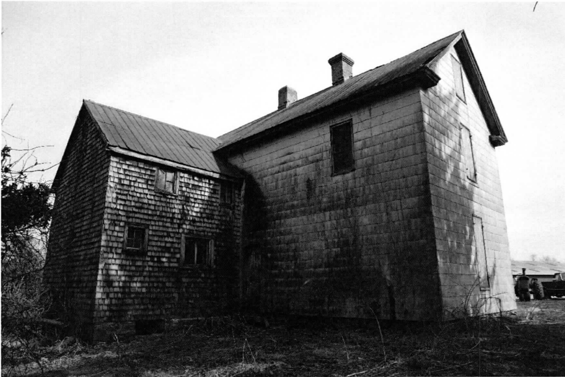
Photo 3 of 24: North & west elevations. 3/20/2019
