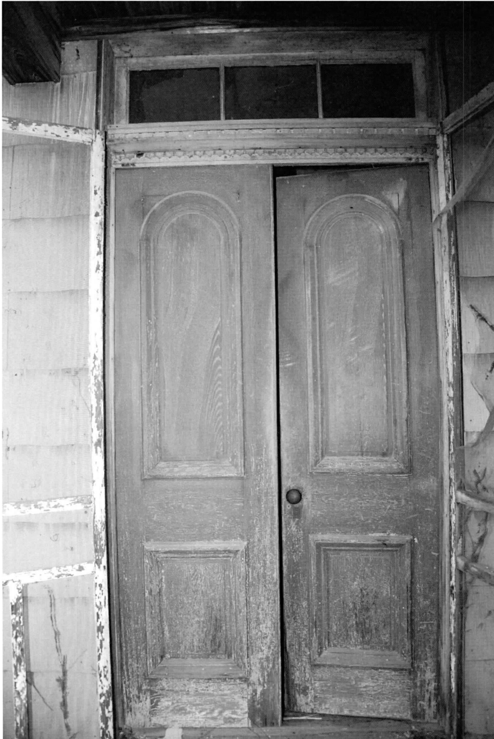
Photo 2 of 24: South elevation, front door. 11/16/2016
