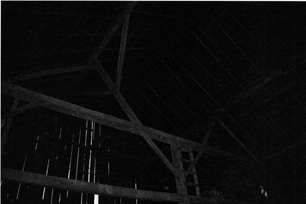
Photo 35 of 36: Bank barn, upper story framing. 11/16/2016
