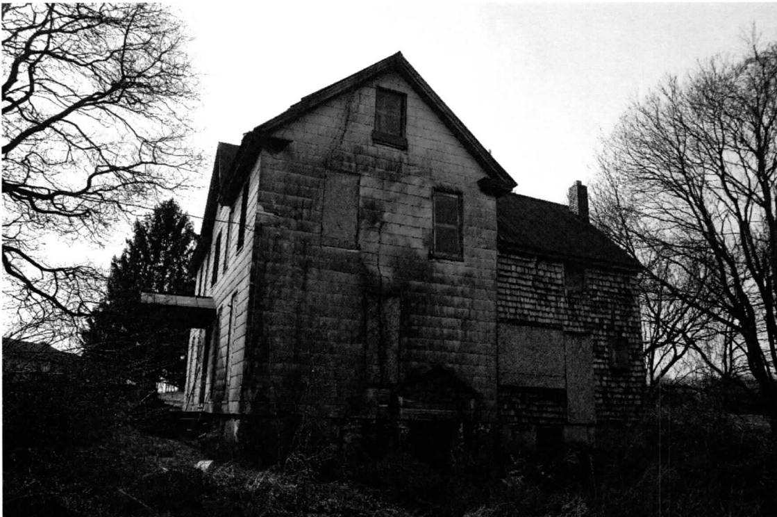
Photo 4 of 24: East elevation. 3/20/2019
