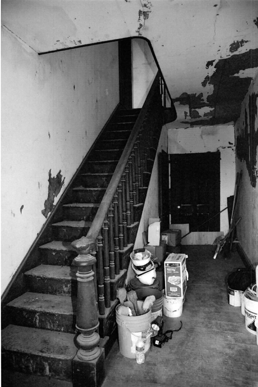
Photo 5 of 24: Passage, view north. 12/27/2019
