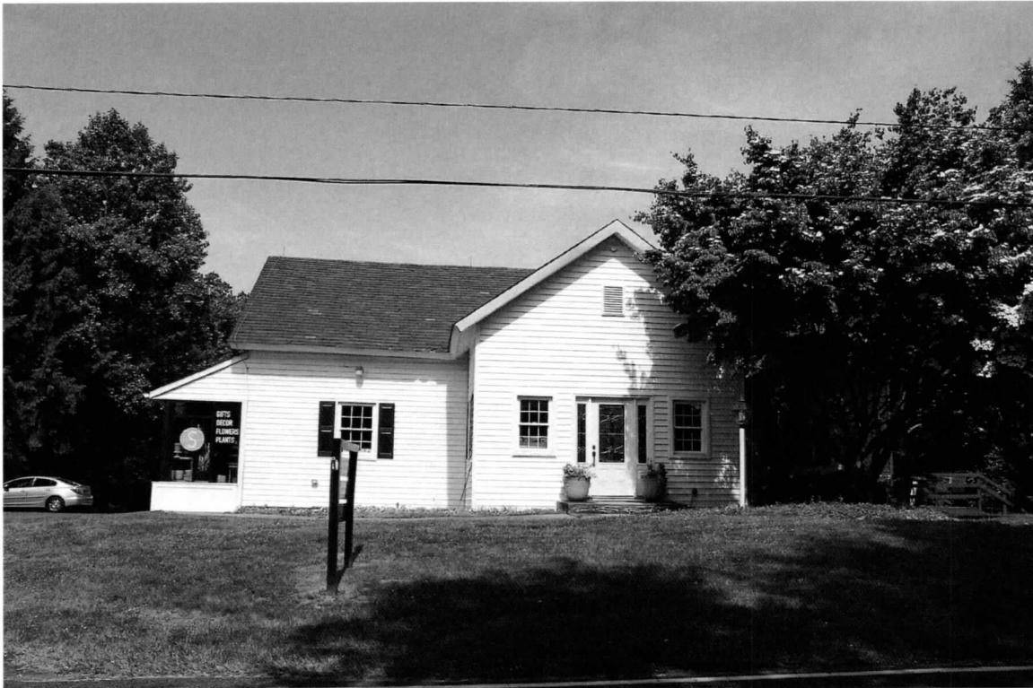
Photo 1 of 10: Façade, camera facing west.
