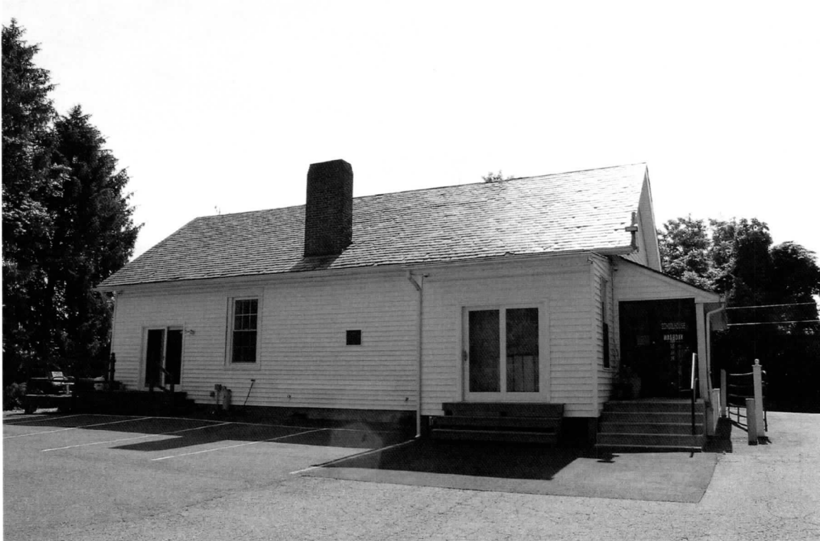
Photo 3 of 10: West Elevation, camera facing east.
