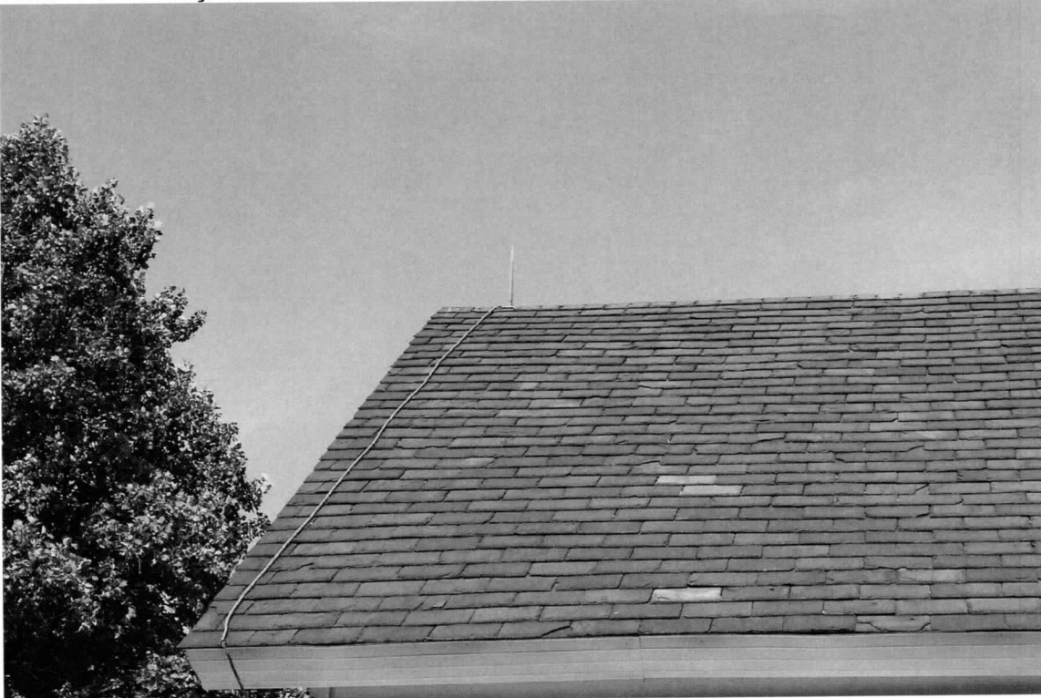
Photo 6 of 10: Detail of Lightning Rod and Slate Roof.
