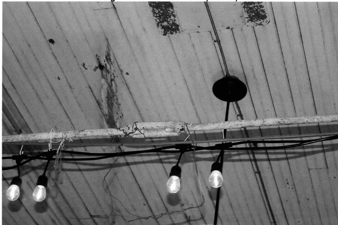
Photo 10 of 10: Detail of Tie Rod (Interior).
