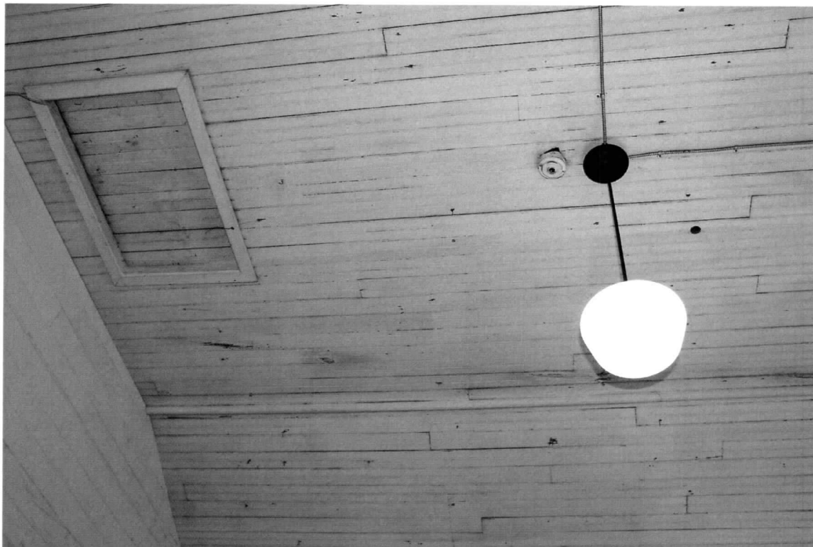
Photo 9 of 10: Detail of Ceiling and Attic Access Panel (Interior).
