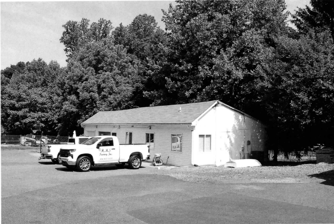
Photo 5 of 10: Façade and East Elevations of Modern Office Building, camera facing northwest.
