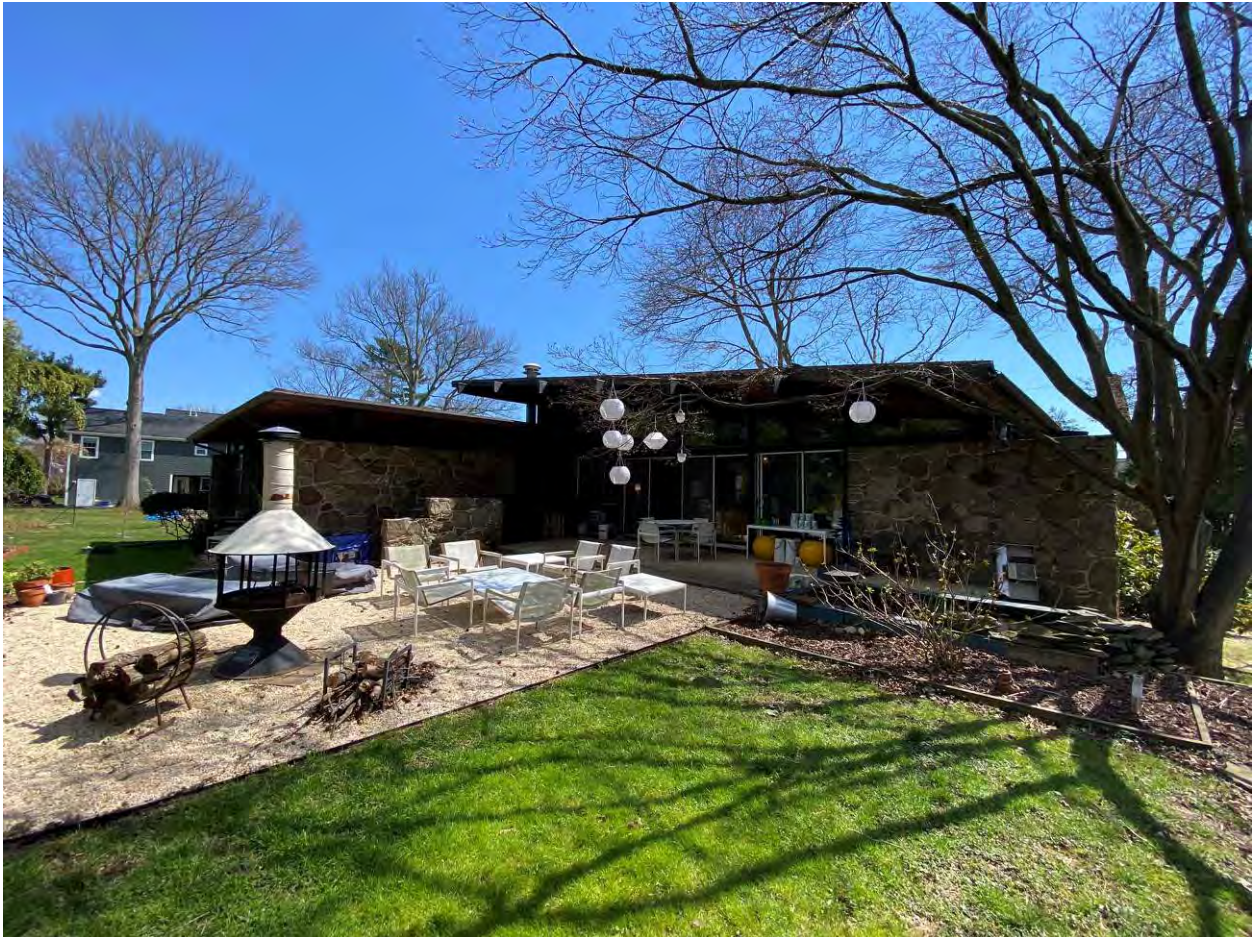
Photo #7 MD_Harford County_Hirsch Residence_0007 north and west elevations, looking southeast
