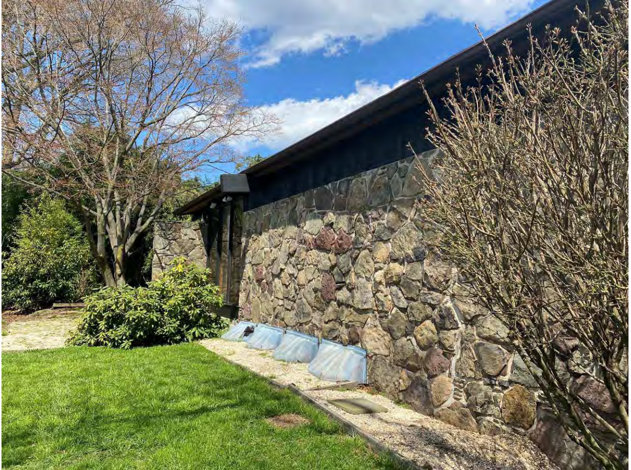
Photo #9 MD_Harford County_Hirsch Residence_0009 west elevation, looking north
