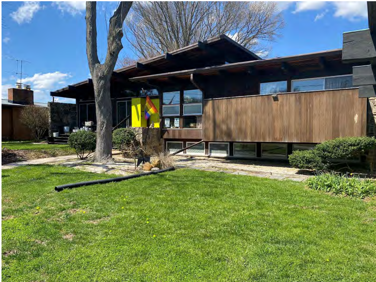
Photo #2 MD_Harford County_Hirsch Residence_0002 south elevation, looking northwest
