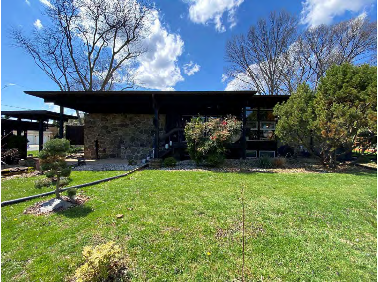
Photo #5 MD_Harford County_Hirsch Residence 0005 east elevation, looking west
