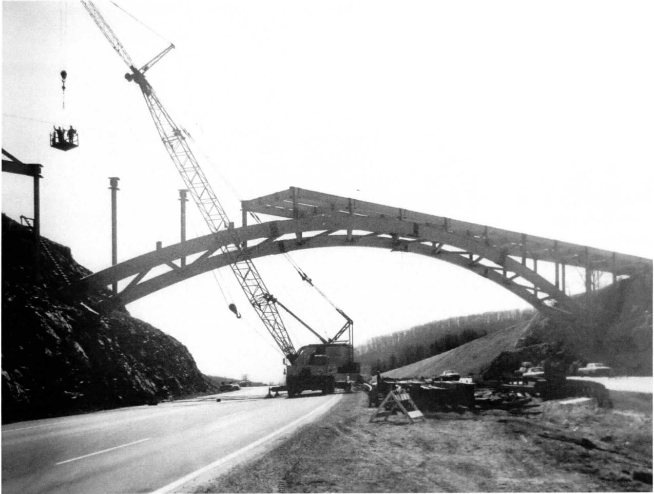
Construction of the bridge, c. 1970 ( Moving Maryland Forward )
