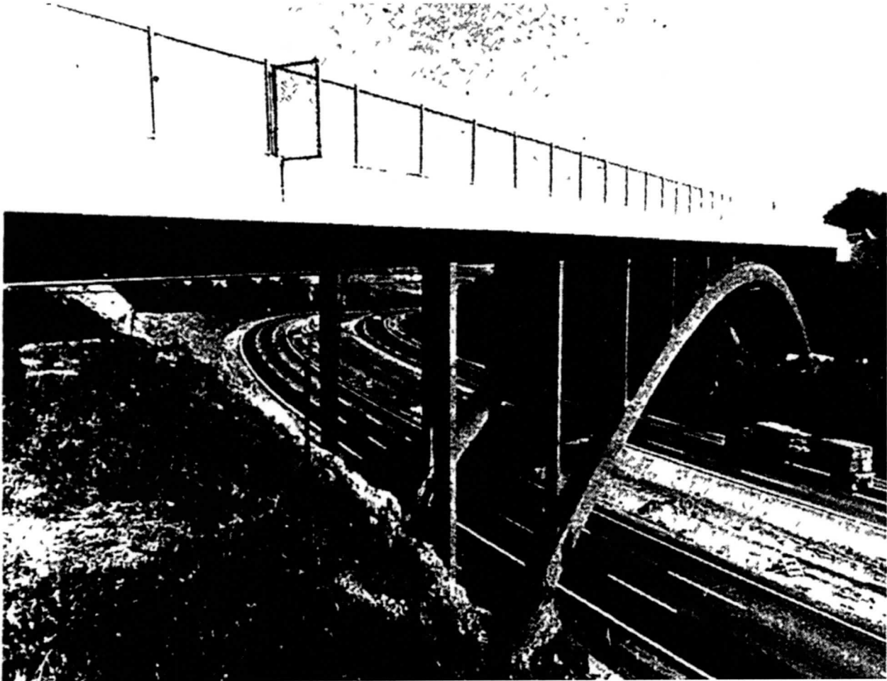
Photograph of the bridge at the time of its opening, 1972 ( The News , May 26, 1972)
