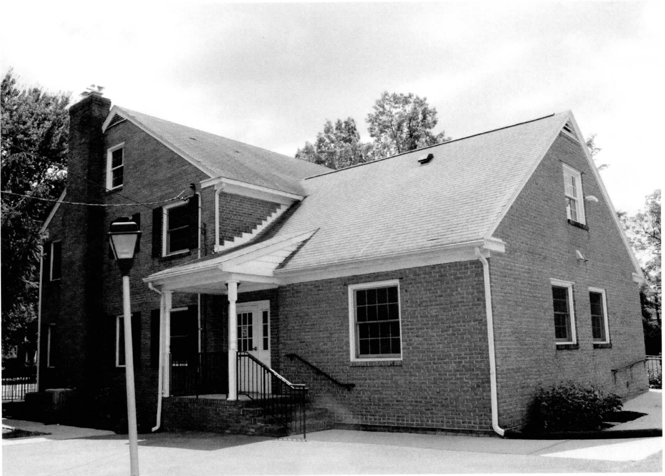
F-3-288 Maryland School for the Deaf Historic District Frederick City, Frederick County, Maryland Meredith Katz August 02, 2021 Building 11; Shockley House, east and north elevations 25/25
