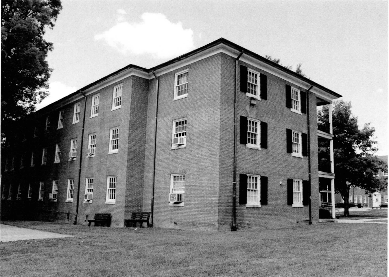
F-3-288 Maryland School for the Deaf Historic District Frederick City, Frederick County, Maryland Meredith Katz August 02, 2021 Building 5; Faupel Hall, east elevation 12/25
