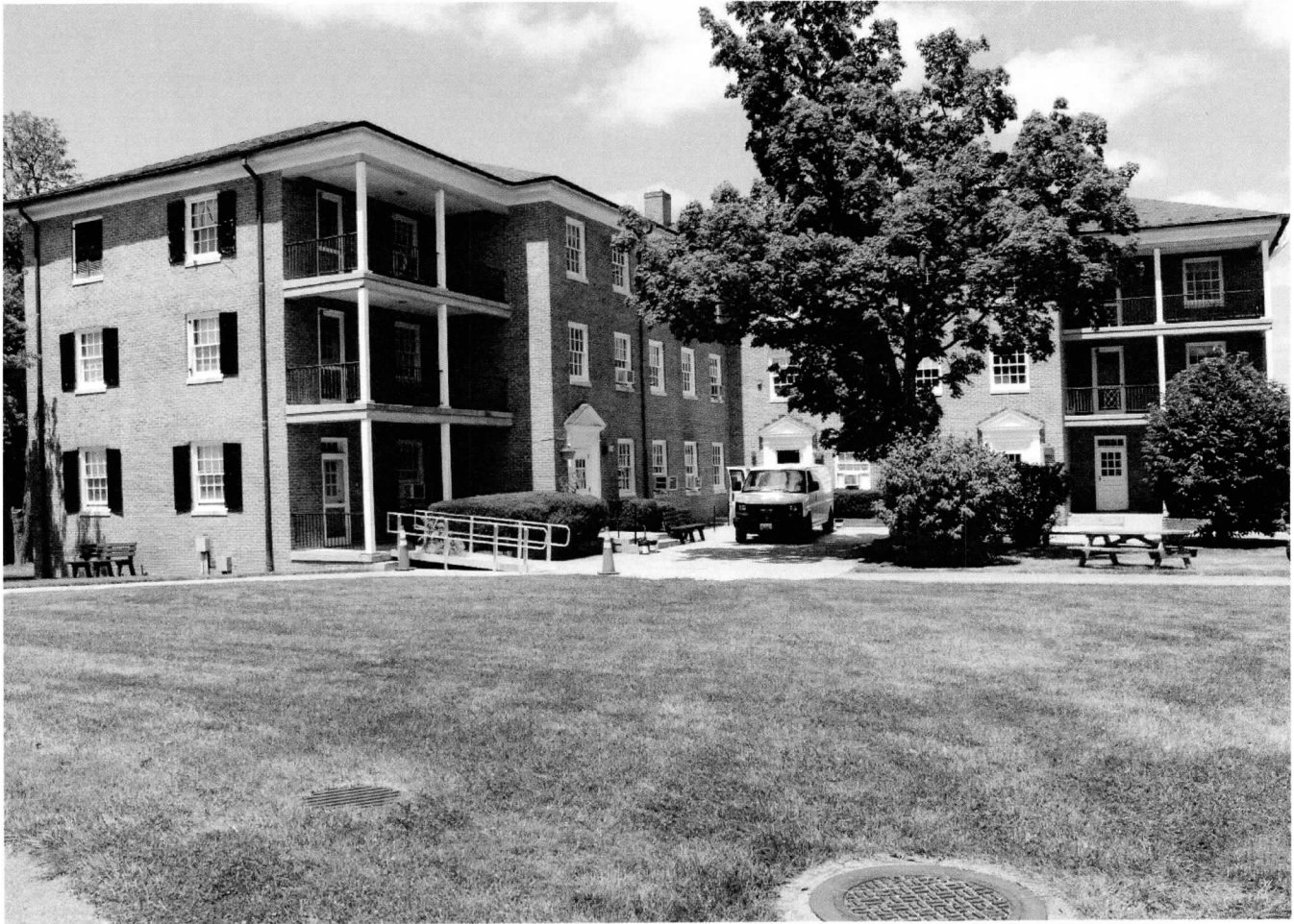
F-3-288 Maryland School for the Deaf Historic District Frederick City, Frederick County, Maryland Meredith Katz August 02, 2021 Building 3; Foxwell-Moylan Hall, south and east elevations 05/25
