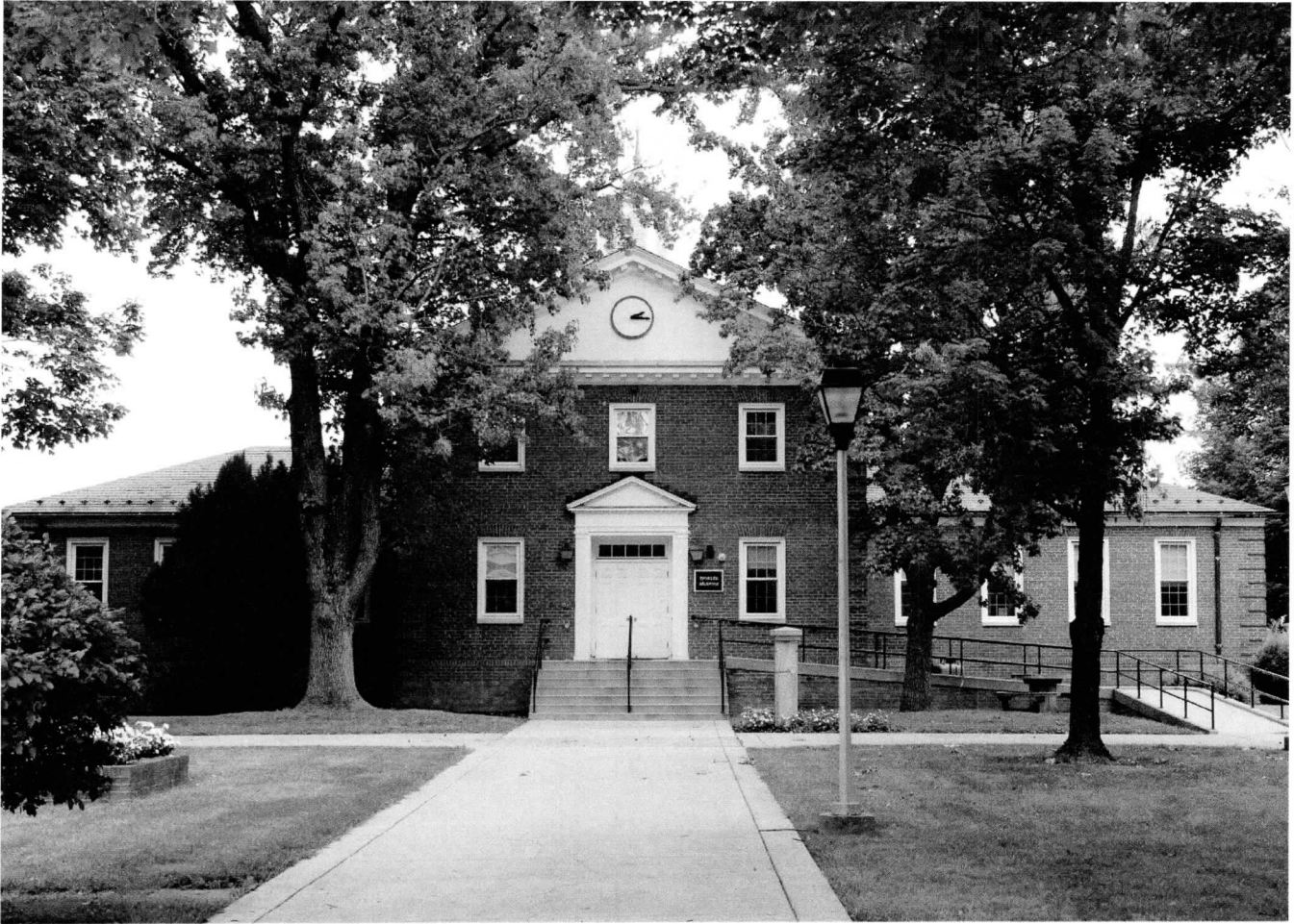
F-3-288 Maryland School for the Deaf Historic District Frederick City, Frederick County, Maryland Meredith Katz August 02, 2021 Building 9; BJORLEE MUSEUM, west elevation 19/25
