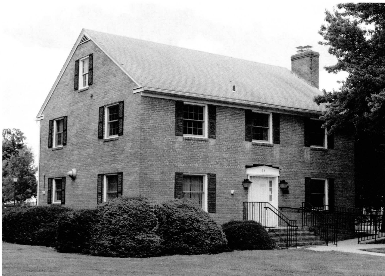
F-3-288 Maryland School for the Deaf Historic District Frederick City, Frederick County, Maryland Meredith Katz August 02, 2021 Building 11; Shockley House, west and south elevations 23/25
