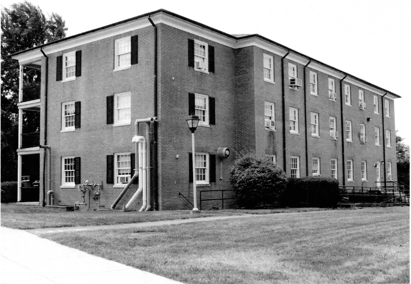
F-3-288 Maryland School for the Deaf Historic District Frederick City, Frederick County, Maryland Meredith Katz August 02, 2021 Building 4; Klipp-Redmond Hall, north and east elevations 08/25
