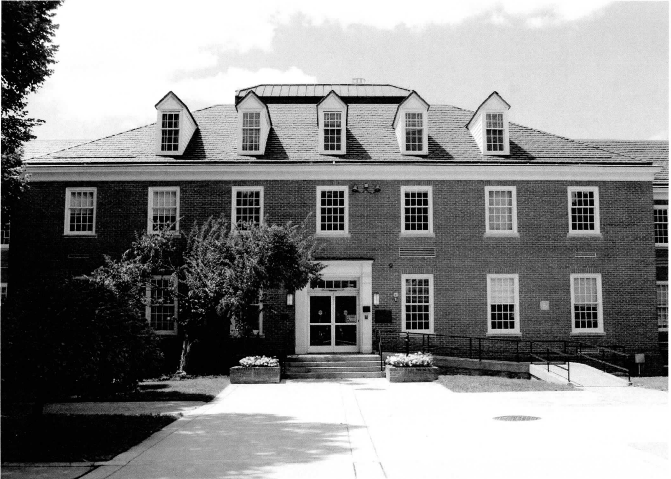
F-3-288 Maryland School for the Deaf Historic District Frederick City, Frederick County, Maryland Meredith Katz August 02, 2021 Building 7; Ely Building-Auditorium, east elevation 16/25
