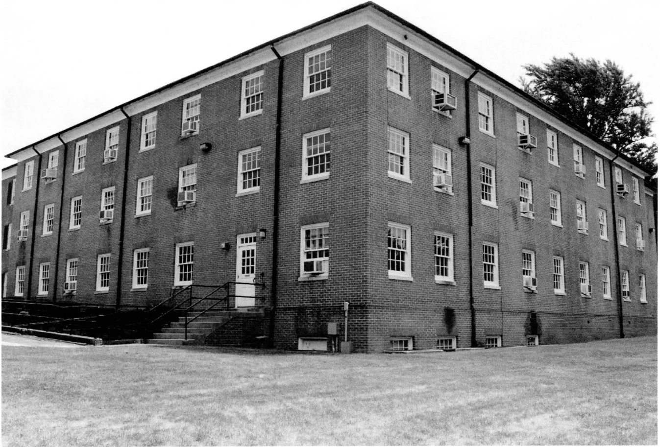
F-3-288 Maryland School for the Deaf Historic District Frederick City, Frederick County, Maryland Meredith Katz August 02, 2021 Building 4; Klipp-Redmond Hall, north and west elevations 09/25
