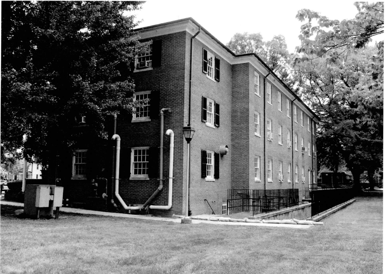
F-3-288 Maryland School for the Deaf Historic District Frederick City, Frederick County, Maryland Meredith Katz August 02, 2021 Building 5; Faupel Hall, north elevation 11/25
