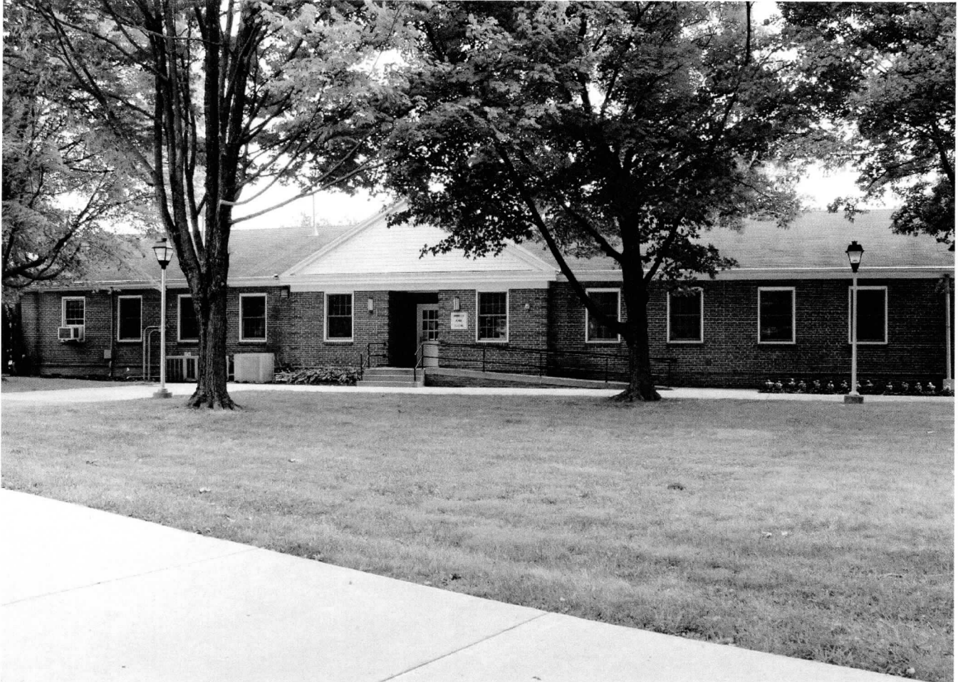
F-3-288 Maryland School for the Deaf Historic District Frederick City, Frederick County, Maryland Meredith Katz August 02, 2021 Building 10; Ambrosen Building, north elevation 21/25
