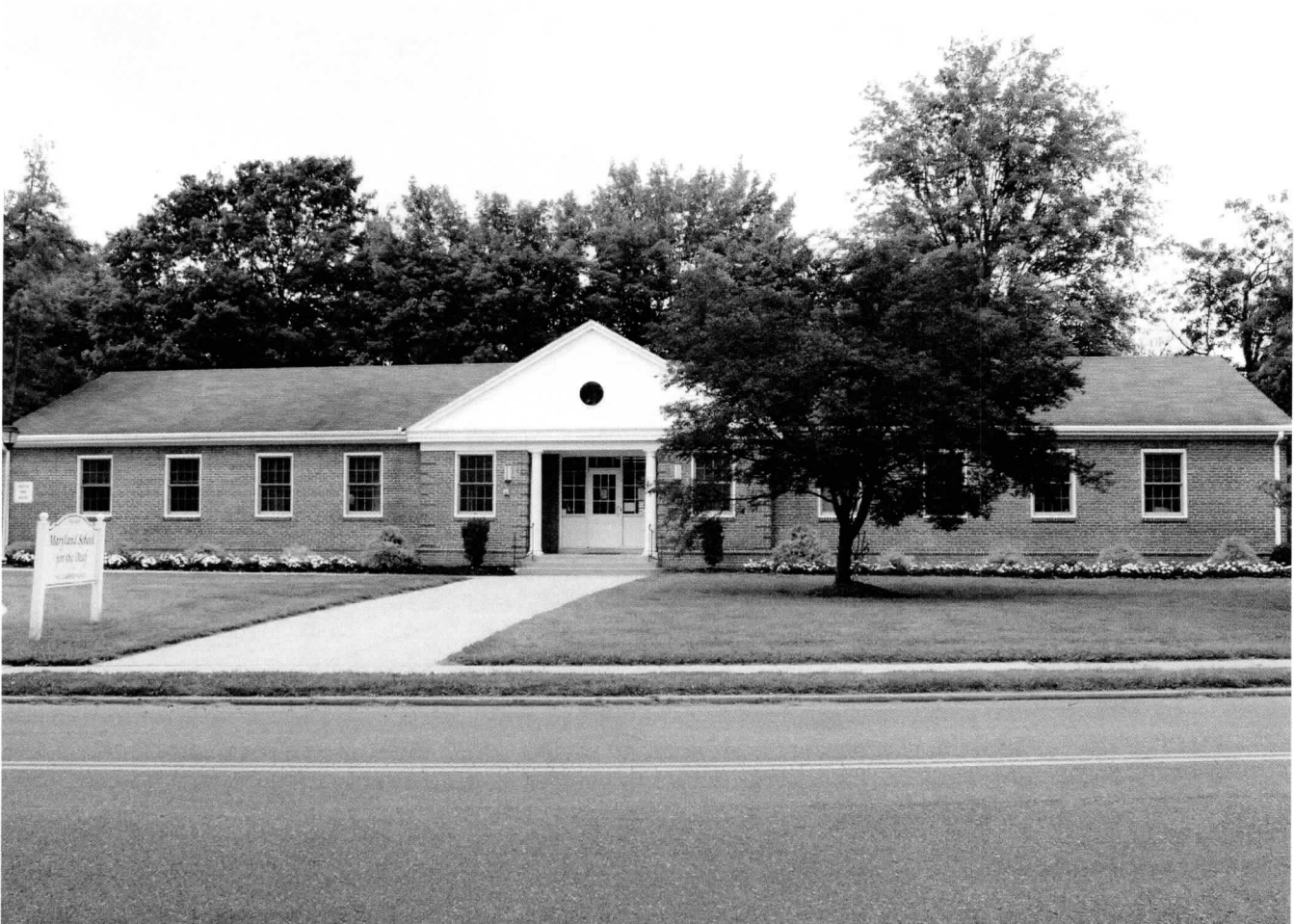
F-3-288 Maryland School for the Deaf Historic District Frederick City, Frederick County, Maryland Meredith Katz August 02, 2021 Building 10; Ambrosen Building, south elevation 22/25
