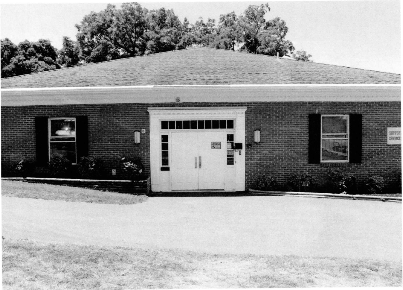
F-3-288 Maryland School for the Deaf Historic District Frederick City, Frederick County, Maryland Meredith Katz August 02, 2021 Building 2; Maintenance Building, south elevation 03/25
