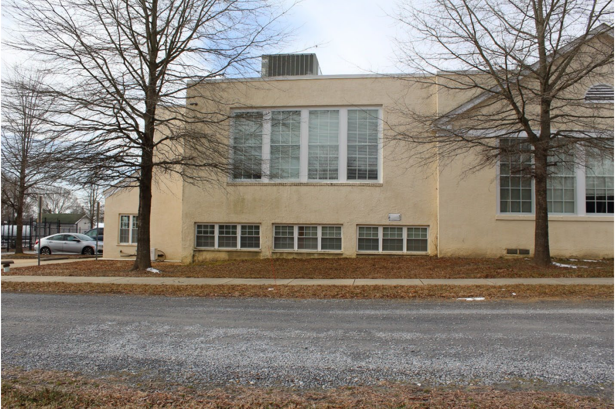
7 of 41 (MD_Charles_BelAltonHighSchool_0007) View of Bel Alton High School cafeteria front looking west
