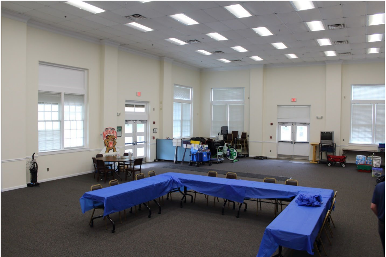
28 of 41 (MD_Charles_BelAltonHighSchool_0028) View of Bel Alton High School showing Auditorium looking northeast at exist doors and windows
