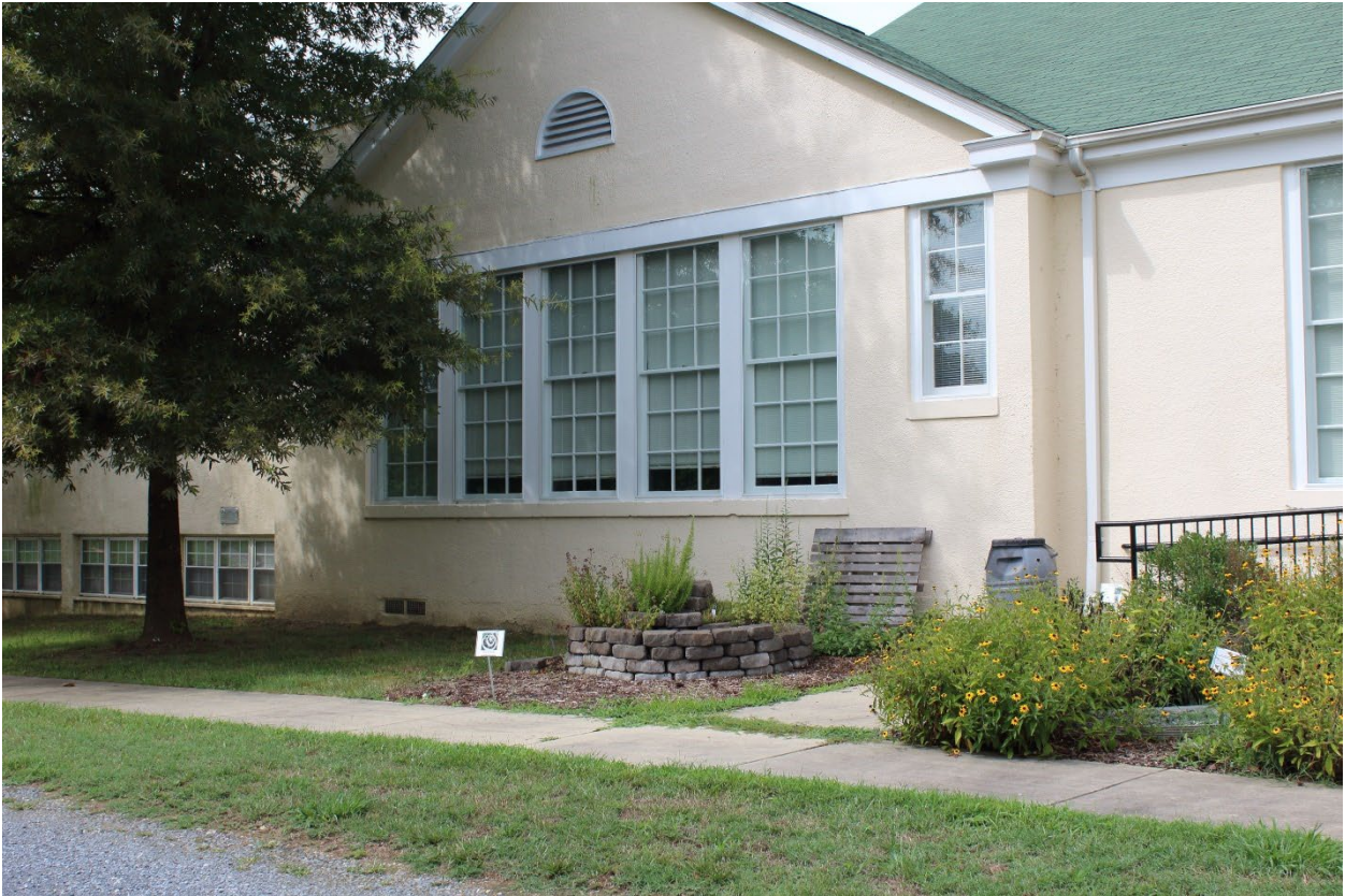
6 of 41 (MD_Charles_BelAltonHighSchool_0006) View of Bel Alton High School south wing
