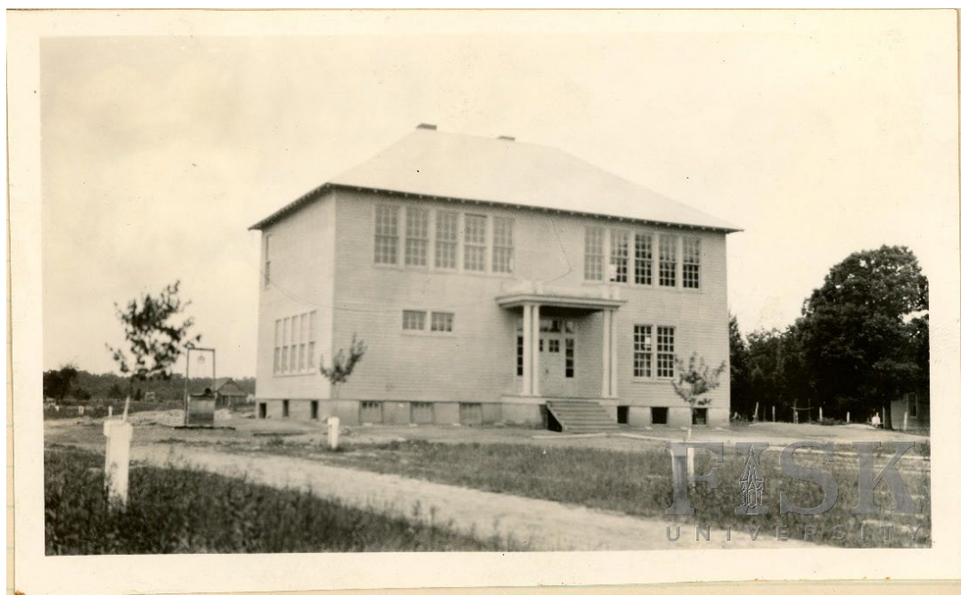
Figure 4. Pomonkey High School, Pomonkey, Charles County, c.1920-1923 (Courtesy of Fisk University, Rosenwald Fund Archives). This building became the Pomonkey Elementary School, but was subsequently destroyed by fire.
