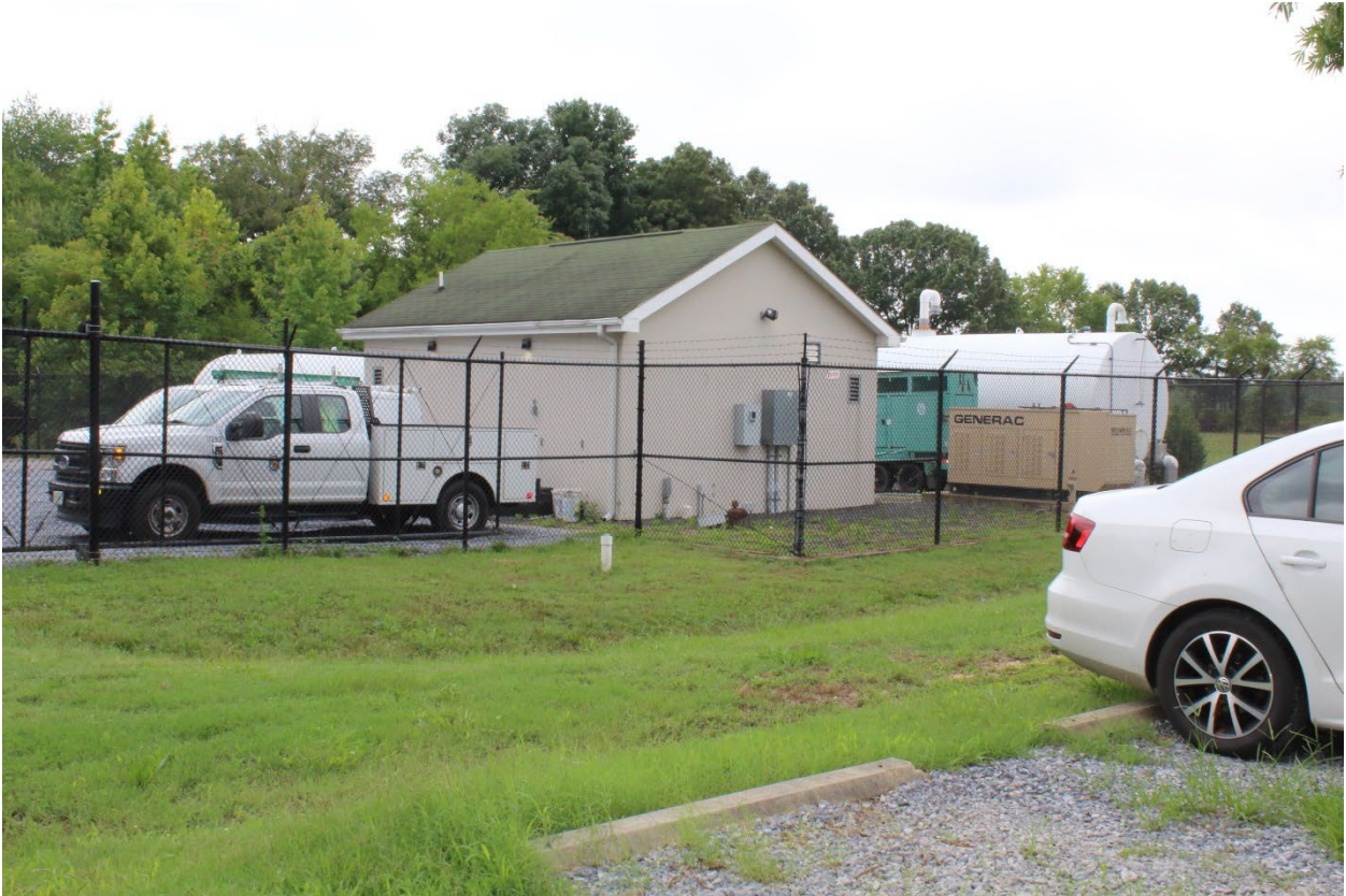
24 of 41 (MD_Charles_BelAltonHighSchool_0024) View of Bel Alton High School looking southwest at 2006 pumping station
