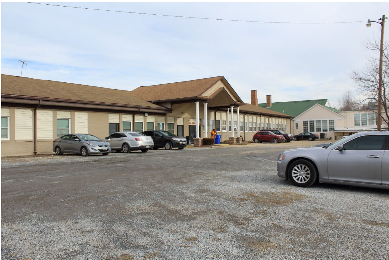
21 of 41 (MD_Charles_BelAltonHighSchool_0021) View of Bel Alton High School at south façade of former High School Annex/Bel Alton Elementary School/Jude House
