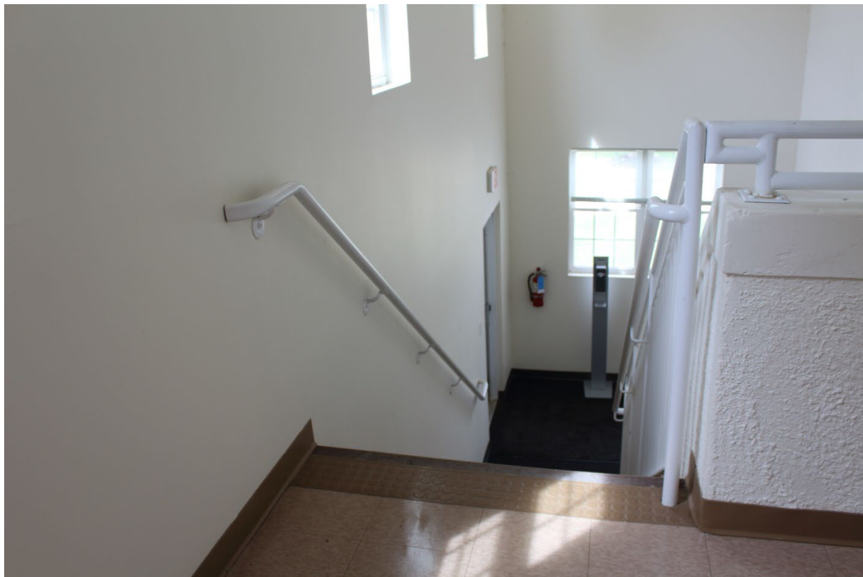
40 of 41 (MD_Charles_BelAltonHighSchool_0040) View of Bel Alton High School showing south exit stair with exit door on left
