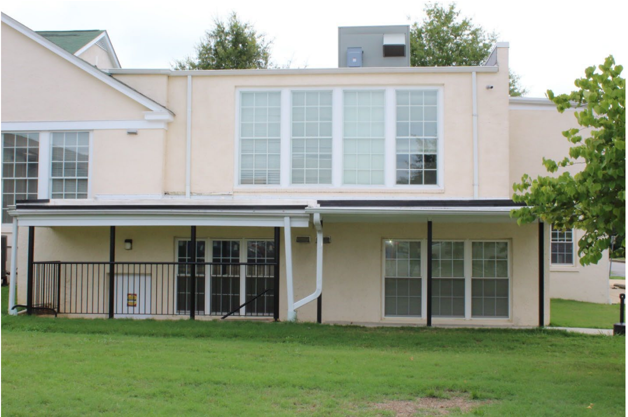
11 of 41 (MD_Charles_BelAltonHighSchool_0011) View of Bel Alton High School west elevation south bays looking east
