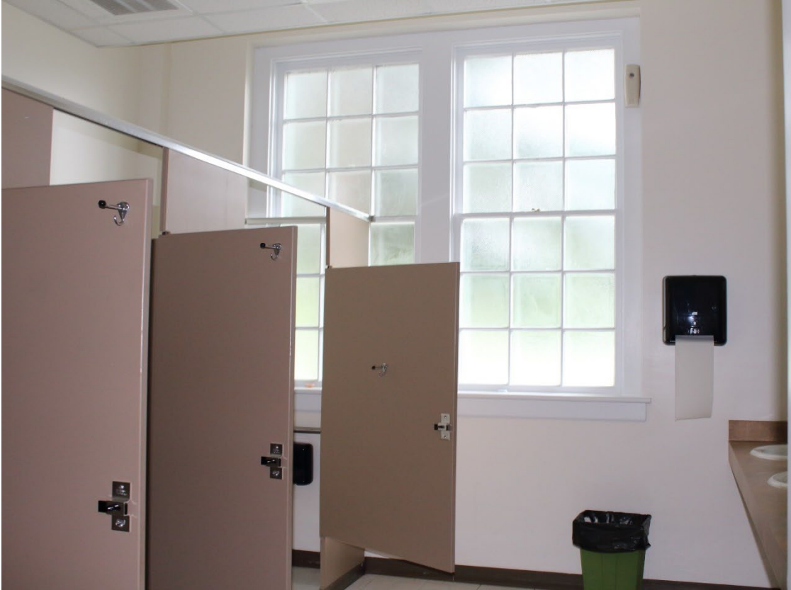
29 of 41 (MD_Charles_BelAltonHighSchool_0029) View of Bel Alton High School showing bathroom showing windows with cathedral glass
